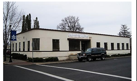
708 SW Deschutes Ave., built 1941
