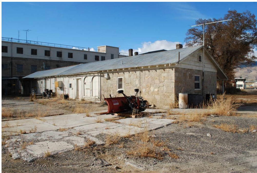
Figure 10. Storage and Maintenance Building.
