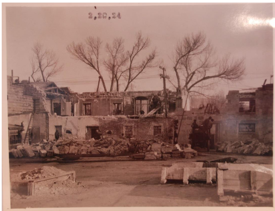
Figure 6. Construction at the Nevada State Prison, c. 1924. Nevada State Prison photograph collection, NSLA
