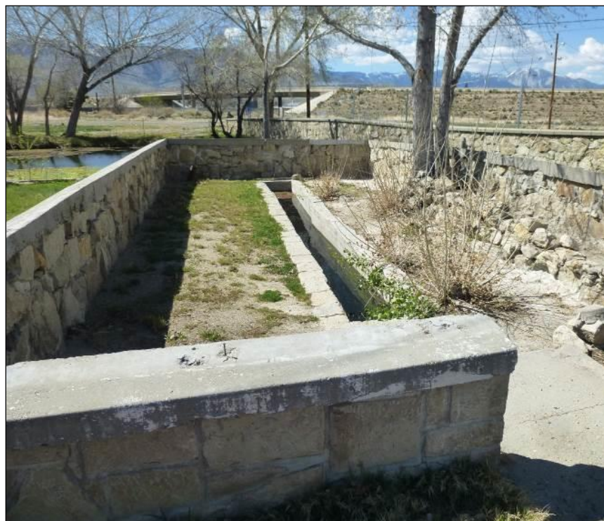
Figure 25. Greenhouse foundation.
