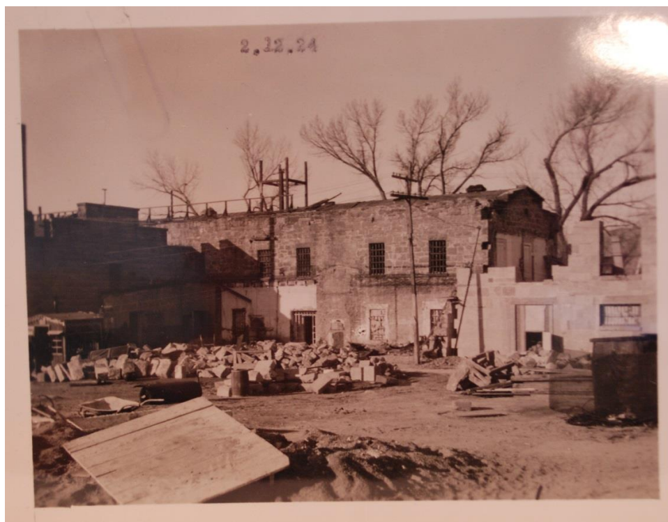
Figure 5. Construction at the Nevada State Prison, c. 1924. Nevada State Prison photograph collection, NSLA
