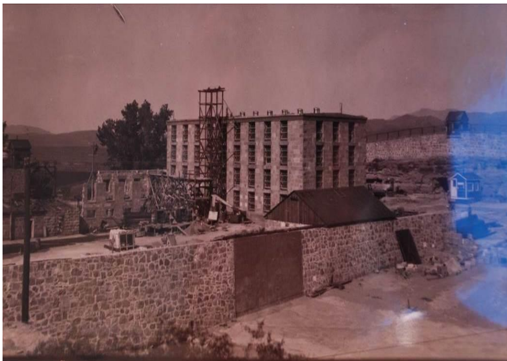
Figure 8. Cell Block A during construction (c. 1925).
