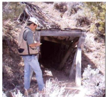
Adit with collapsing entrance.
