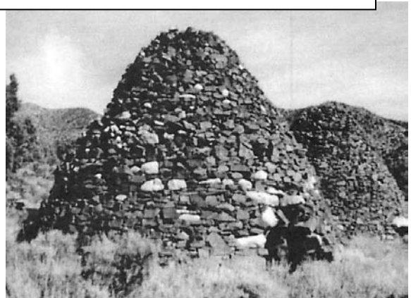
Tybo Charcoal Kilns built in 1874 to smelt the silver out of the difficult ore.*
