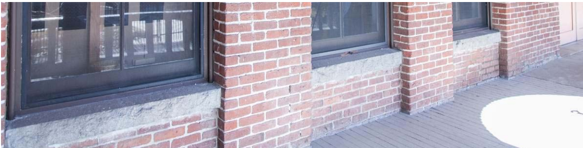
Figure 39: Porch floor as it appears today. Note warped floor boards along brick wall. Image Source: IS Architecture, March 2015.
