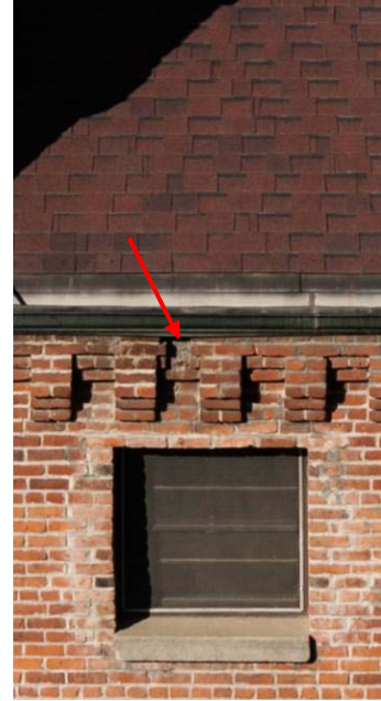
Figure 42 (left): Brick corbels on the north façade were removed when in 1952 a fire escape was installed. Figure 43 (right): Detail view of the east façade showing missing brick corbels. In this case, a downspout was installed at an unknown date and removed in 1952. Image Source: IS Architecture, March 2015.
