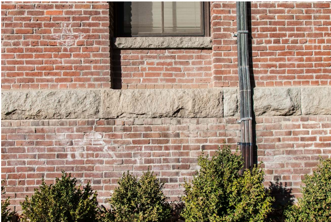
Figure 52: View of east façade showing brick experiencing efflorescence. Image Source: IS Architecture, March 2015.
