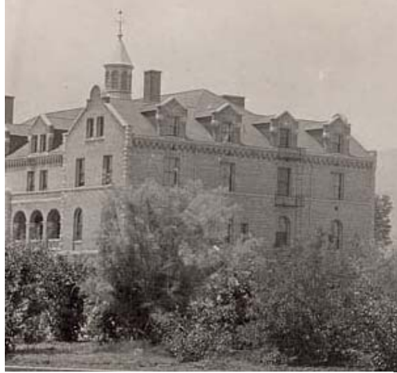
Figure 23: East façade fire escape, 1912. Image Source: UNRA-P229-1.
