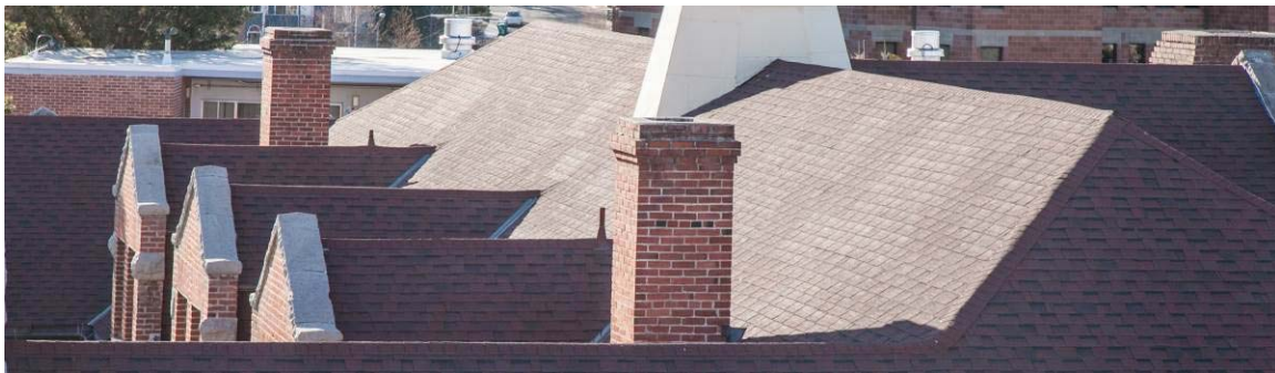
Figure 71: View west over roof line showing chimneys as they appeared in March 2015. Image Source: IS Architecture.
