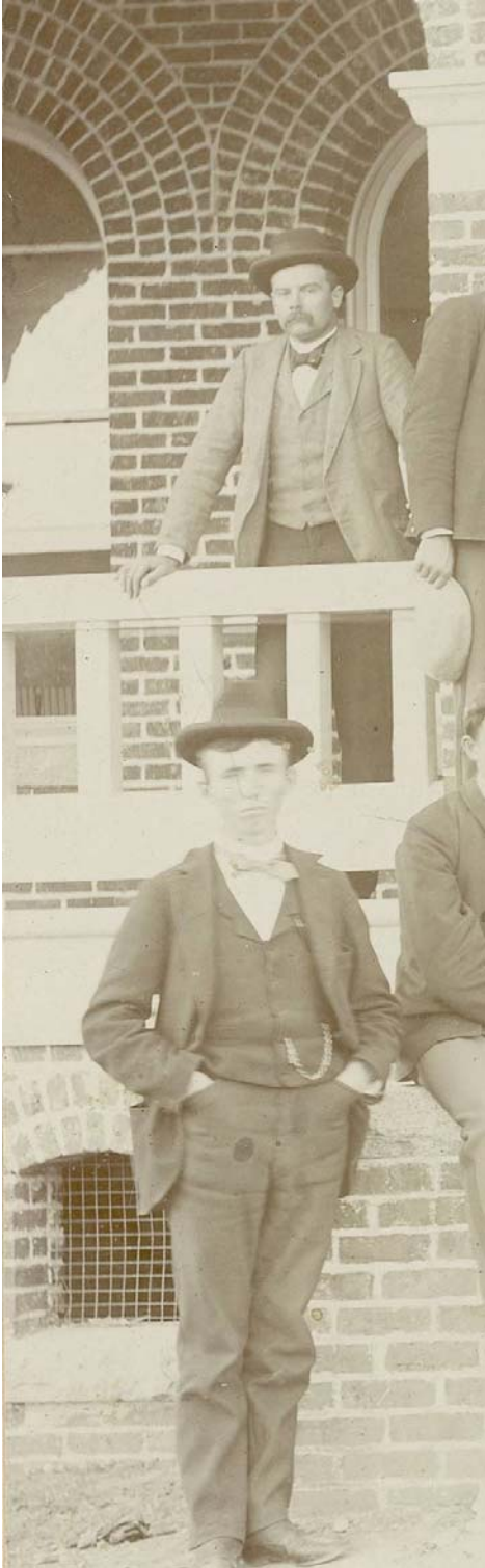
Figure 46 (left): Detail view of historic woven metal mesh at basement vent openings. Image Source: UNRA-P59-1, c.1907. Figure 47 (top right): Typical enlarged vent opening at west side of Lincoln Hall. Figure 48 (middle right): Vent openings on the south façade which have been modified. Figure 49 (bottom right): Vent opening on the north façade showing gap between wythes where woven metal mesh was once present. Image Source: IS Architecture, March 2015.
