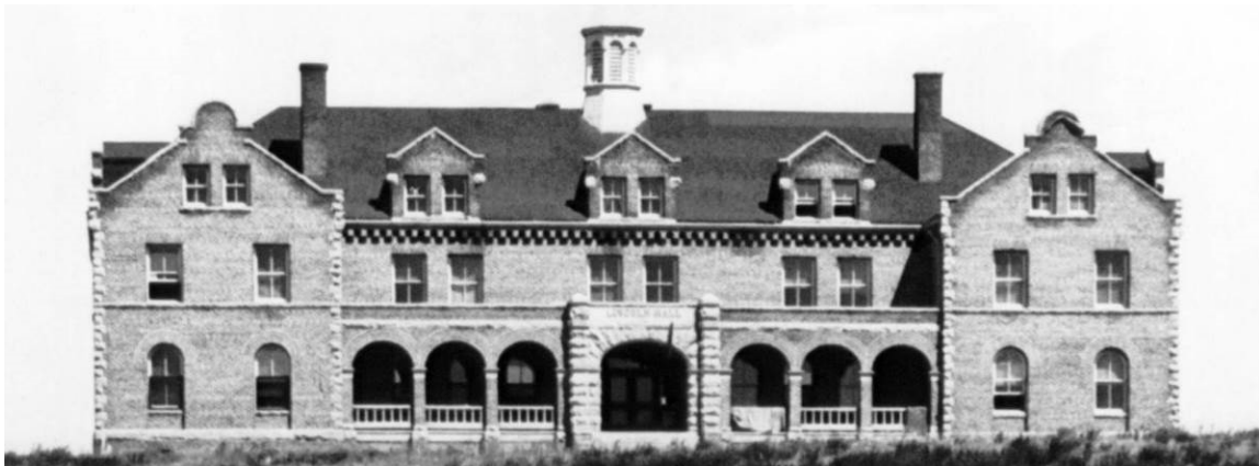
Figure 70: South façade of Lincoln Hall c. 1896 showing original height of chimneys. Image Source: UNRA-P232-01.
