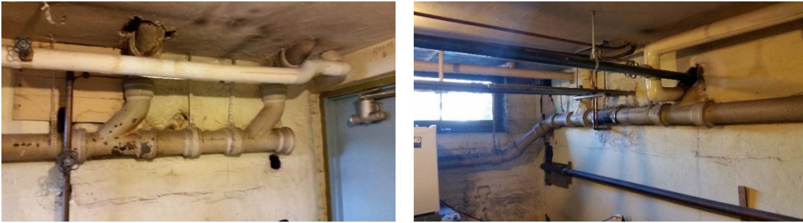
Figure 11: Building Waste Piping – Room 6
