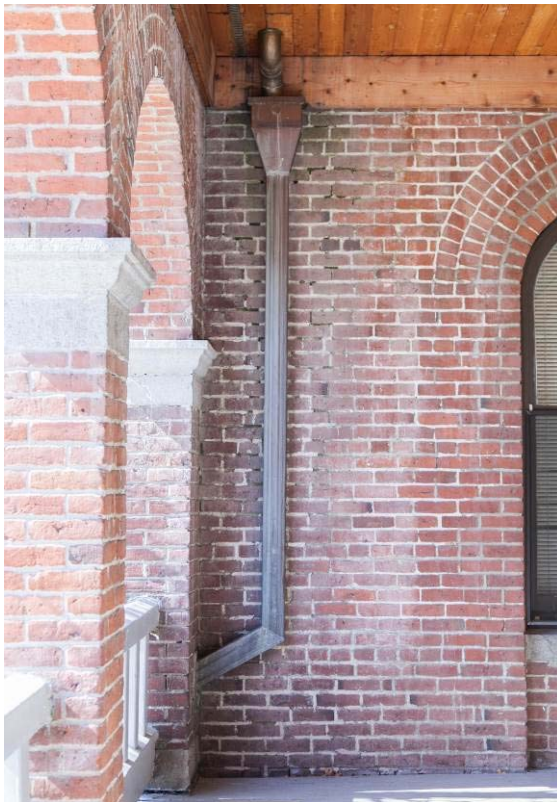
Figure 31 and Figure 32: West and east walls of porch showing water damage to brick wall. Image Source: IS Architecture, March 2015.
