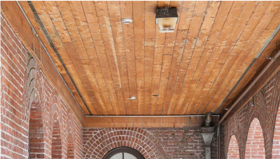
Figure 38: Porch ceiling as it appears today. Note: box beams are missing and ceiling boards have been replaced. No historic material remains. Image Source: IS Architecture, March 2015.
