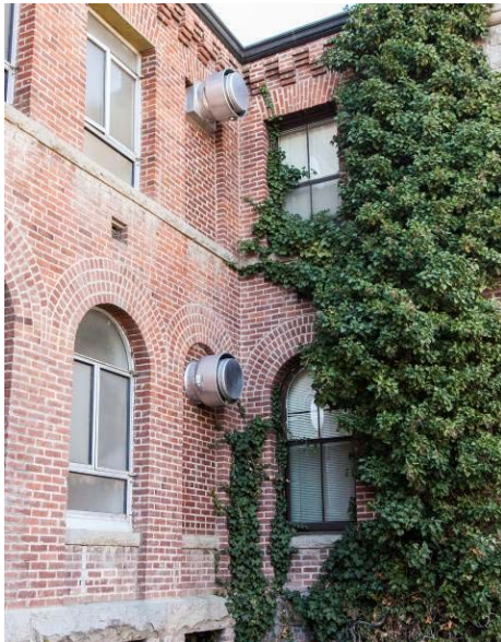
Figure 50 (left): West interior corner of north façade showing ivy growth over existing drainage assembly.
