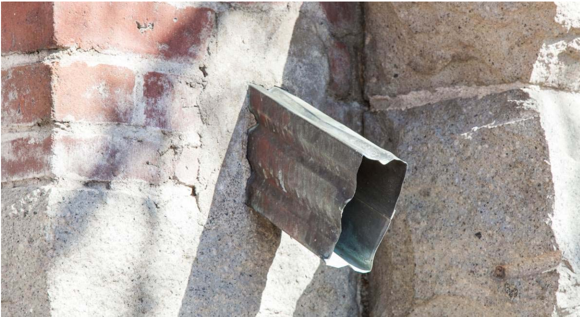
Figure 35: Detail view of downspout outlet. The west side of the porch has the same configuration. Image Source: IS Architecture, March 2015.
