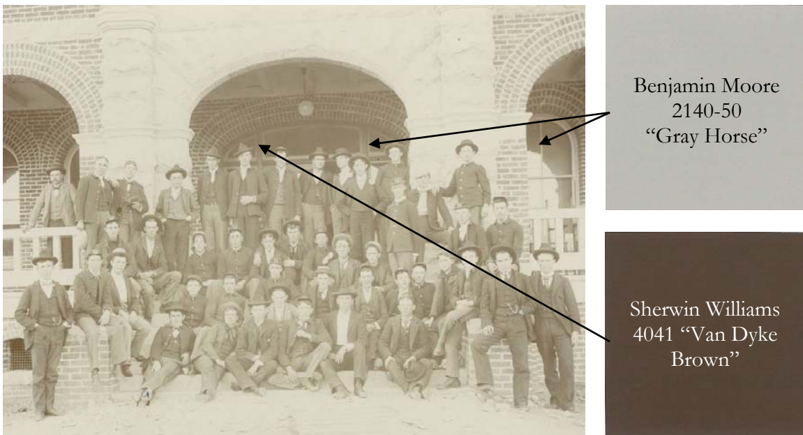
Figure 73: Historic photograph, c.1907 with men sitting on south entry steps of Lincoln Hall. Paint analysis revealed the exterior window trim was painted gray (Benjamin Moore 2140-50 “Gray Horse”) and the exterior door trim was painted with the same gray as well as a greenish-brown (Sherwin Williams 4041 “Van Dyke Brown”).
