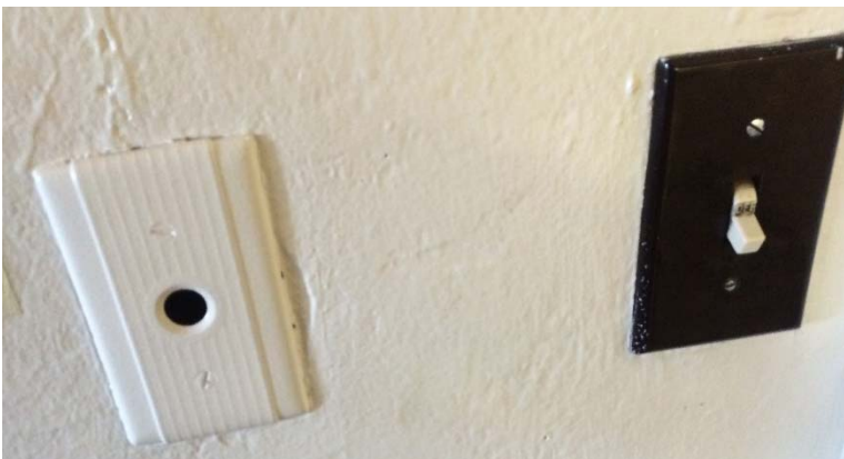
Figure 21: Typical lighting snap switch shown on the right with old pushbutton switch cover plate shown on the left.
