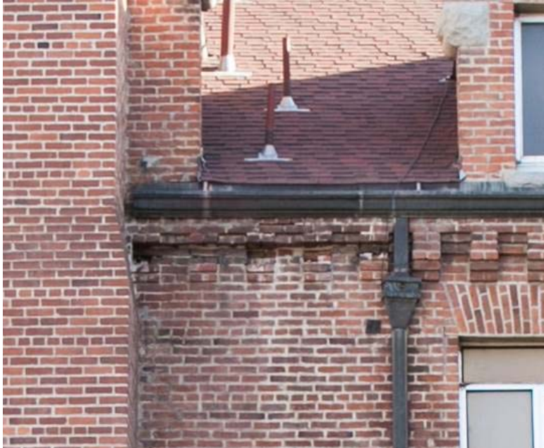
Figure 42 (left): Brick corbels on the north façade were removed when in 1952 a fire escape was installed. Figure 43 (right): Detail view of the east façade showing missing brick corbels. In this case, a downspout was installed at an unknown date and removed in 1952. Image Source: IS Architecture, March 2015.
