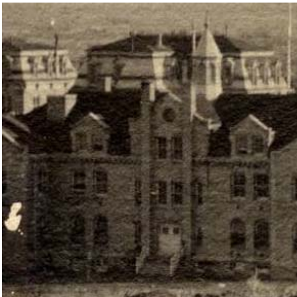
Figure 66: View of north facade c. 1900 showing the brick stacks of equal height. Image Source: UNRA-P254-2.
