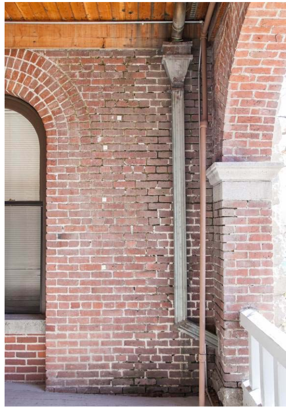
Figure 31 and Figure 32: West and east walls of porch showing water damage to brick wall. Image Source: IS Architecture, March 2015.
