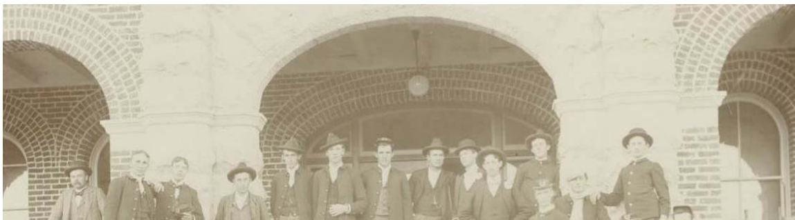
Figure 36: Historic photograph of men standing on south steps of Lincoln Hall. Visible is the original porch ceiling design and globe pendant. Image Source: UNRA-P59-1, c. 1907.
