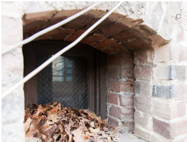
Figure 46 (left): Detail view of historic woven metal mesh at basement vent openings. Image Source: UNRA-P59-1, c.1907. Figure 47 (top right): Typical enlarged vent opening at west side of Lincoln Hall. Figure 48 (middle right): Vent openings on the south façade which have been modified. Figure 49 (bottom right): Vent opening on the north façade showing gap between wythes where woven metal mesh was once present. Image Source: IS Architecture, March 2015.
