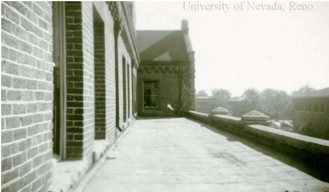
Figure 30: View east porch roof from Room 210. Image Source: UNRA-P3376124, c.1945.
