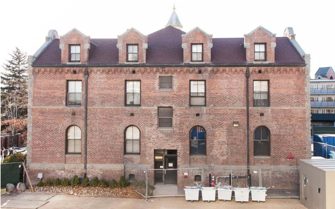
Figure 61: Overview of east facade showing typical historic first, second and third floor windows. Note: door and windows above are not original to Lincoln Hall. Image Source: IS Architecture, March 2015.
