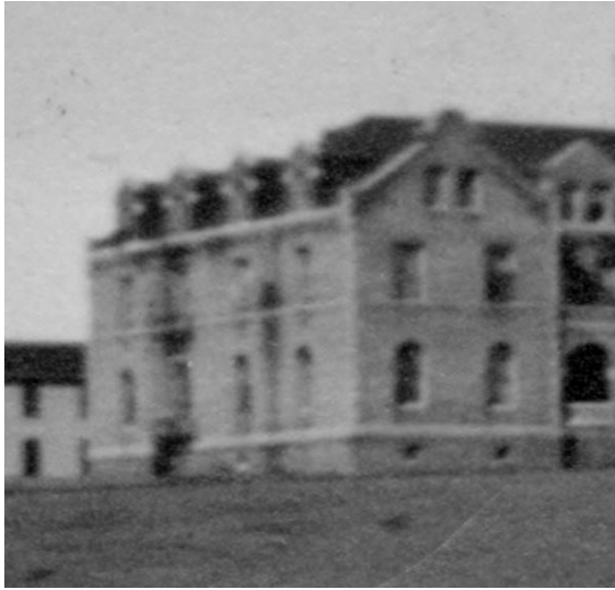
Figure 22: West façade fire escape, circa 1920. Image Source: UNRA-P3150.
