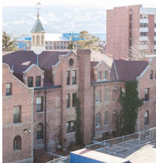
Figure 67: View of north facade showing newer brick mechanical stack in the background and shortened historic brick stack in the foreground. Image Source: IS Architecture, March 2015.
