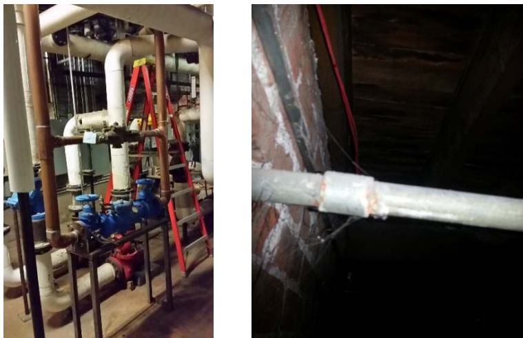
Figure 12: Domestic Water Piping – Room 7
