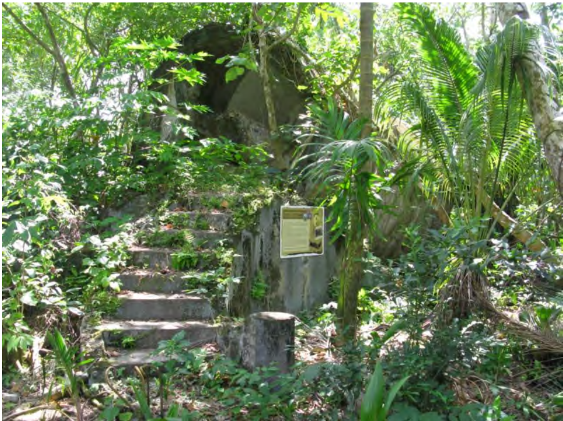
Photo 7. Remains of the old Japanese lighthouse at Dalap in Lebinaw Village, Gagil Municipality (source: missingaircrew.org ). Note the interpretive sign on the structure wall in the center of the photograph.
