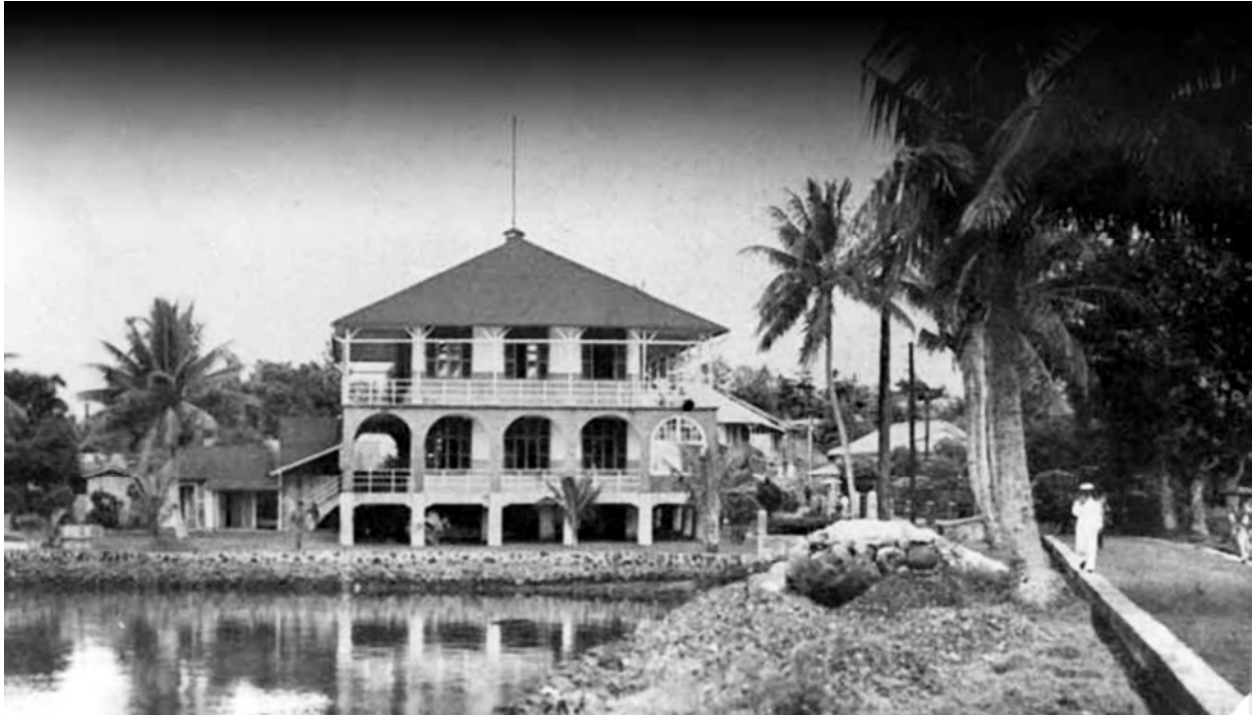
Photo 10. Headquarters for the German cable station on Marbaa; opened in 1905. The building was later converted into a post office by the Japanese administration (source: Micronesian Seminar and Trust Territory Photo Archives, University of Hawai'i).
