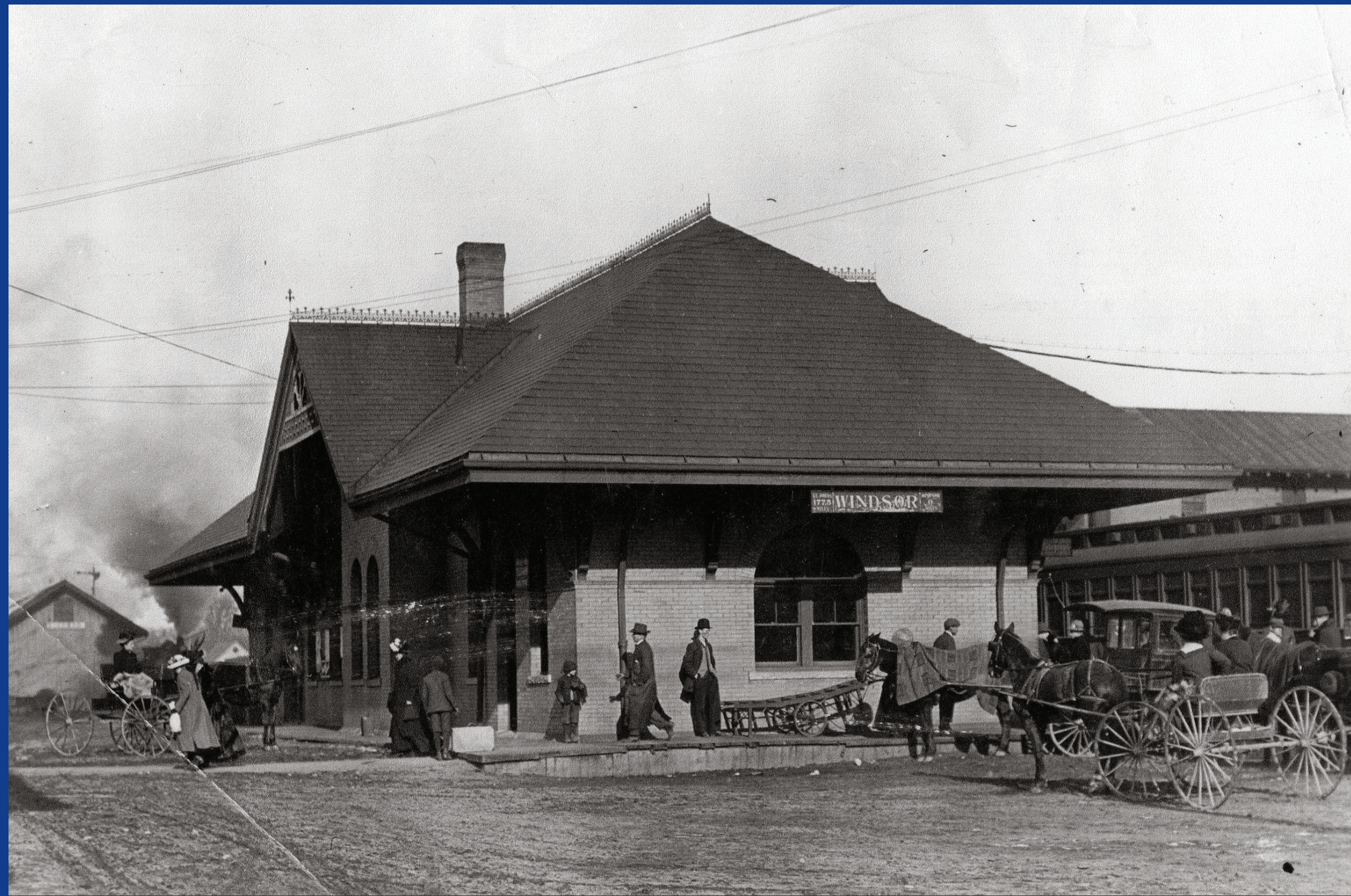
The 1901 passenger station boasted modern amenities like electric lighting and a sheltered platform.
