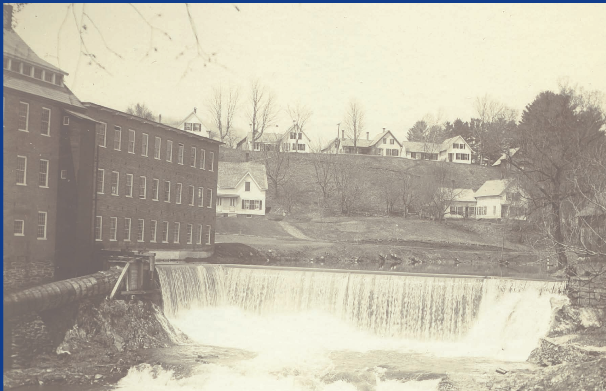
The wooden penstock ( above left ), installed in the early 1870s, fed a water turbine that worked with a steam engine to power the site. ( Factory Complex Sales Prospectus , c. 1915) Courtesy Windsor Historical Society
