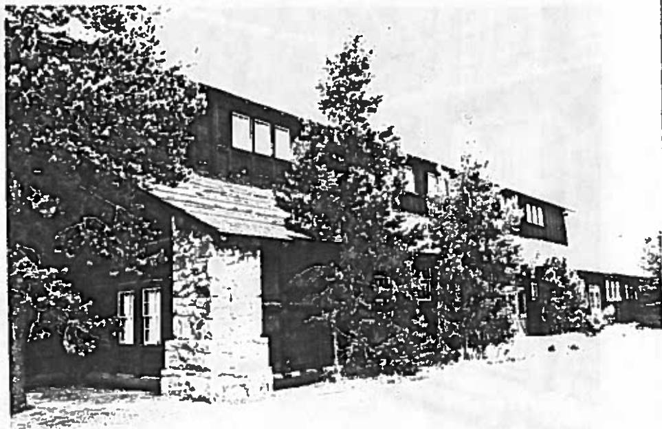
Figure 85: Looking northwest at the east side of the Recreation Hall. The upper windows have some weathered sills and there appears to be some open areas around the windows.
