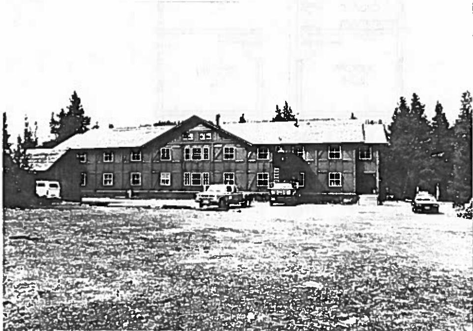
Figure 193: Looking north at the Dormitory building. The wood shingle roof is being replaced as this photo is taken.
