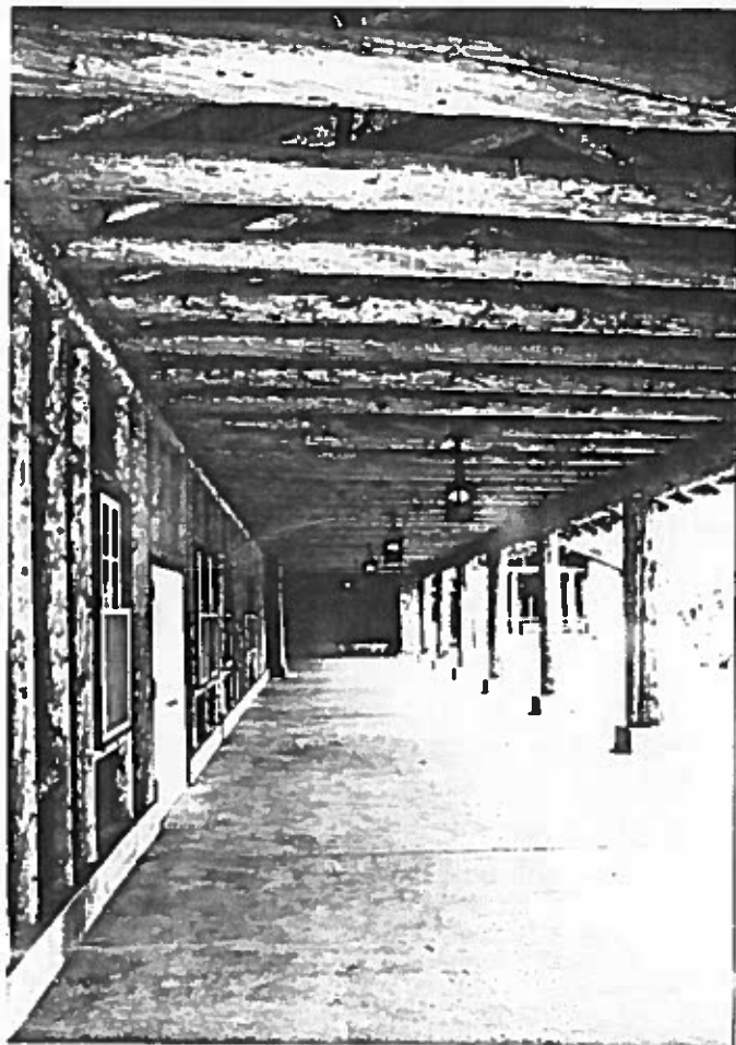
Figure 99: Looking east at a window under the covered connection between the Recreation Hall and the Lodge Building. The windows are in good condition.
