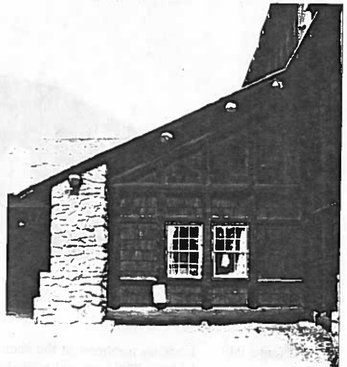
Figure 96: Looking north at the end wall of the side aisle on the south side.
