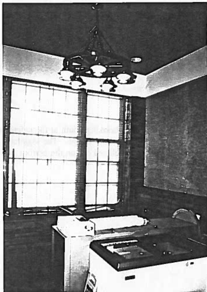
Figure 135: Looking west at an outside window in a workroom on the west side of the Lodge. Generally the windows are in good condition on the inside.
