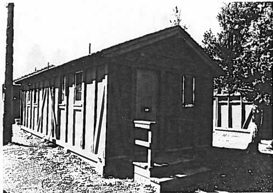
Figure 166: Looking northwest at a typical frame-out duplex cabin (#108-109). Note the use of a concrete stoop on one end and a wooden stoop and rail on the other end.
