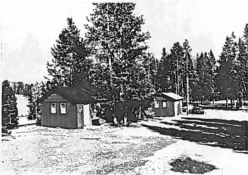
Figure 25: Looking east along the employee cabins on the north end of the site.
