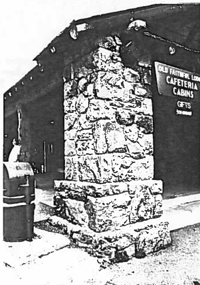
Figure 108: Looking at another stone pier on the southwest corner of the building and porch on the west side. The materials appear to be in good condition.
