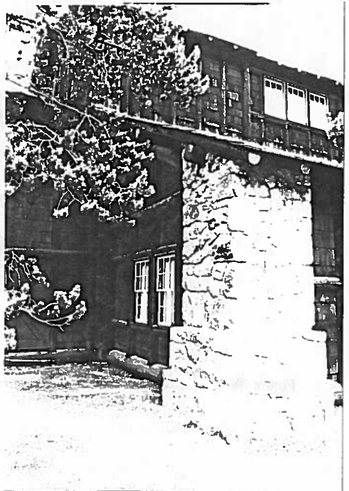
Figure 85: Looking northwest at the east side of the Recreation Hall. The upper windows have some weathered sills and there appears to be some open areas around the windows.
