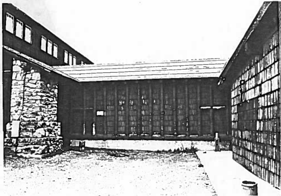
Figure 73: Looking south at a log-out structure which connects the kitchen storage area with the Rec Hall. The roof appears in good condition. The walls have some loss of stain.
