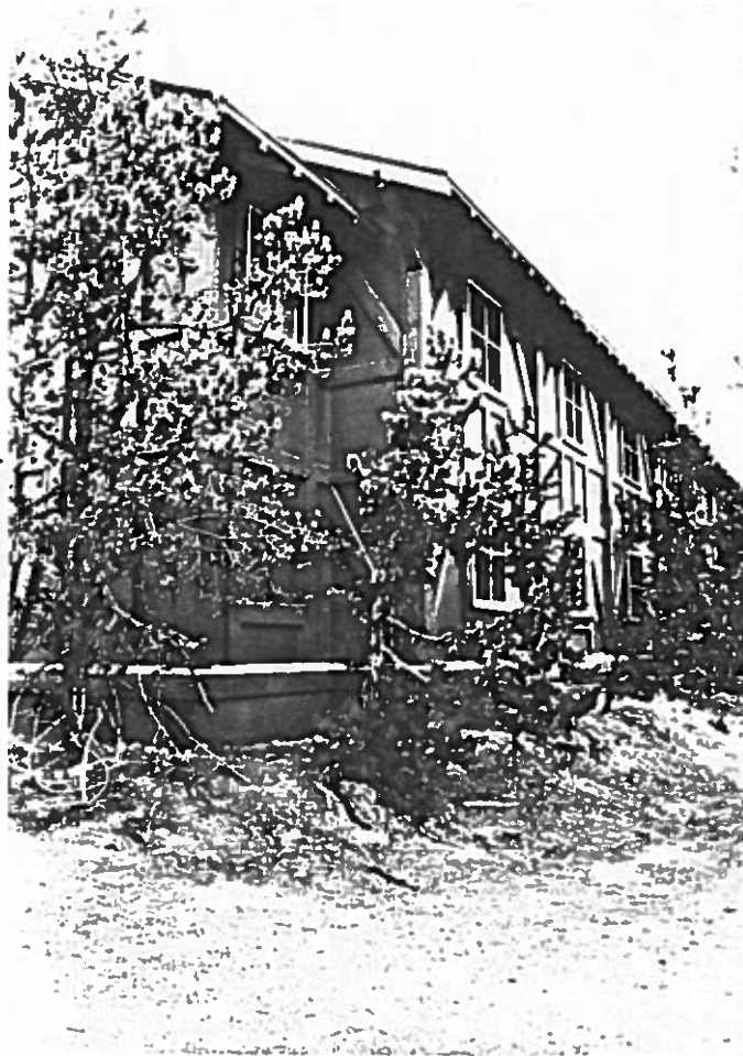
Figure 196: Looking southwest at the Dormitory building. The trees could become a problem because of the location next to the building.
