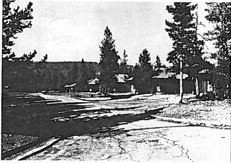
Figure 28: Looking north at the employee quad housing on the east side of the lower loop. This area has some curbs and designated parking which protects some of the fragile landscaped areas.
