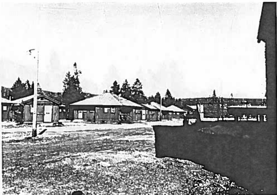
Figure 13: Looking east at the cabin area from the west end of Old Faithful Lodge. Note the street lights on the poles. This is also the view from the boardwalk of the geyser.
