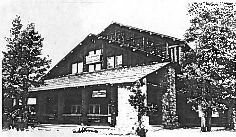
Figure 87: Looking northwest at a corner of the Rec Hall. Note the weathered base log and sills at the door and windows. The grade varies at this point allowing water to flow under the building.
