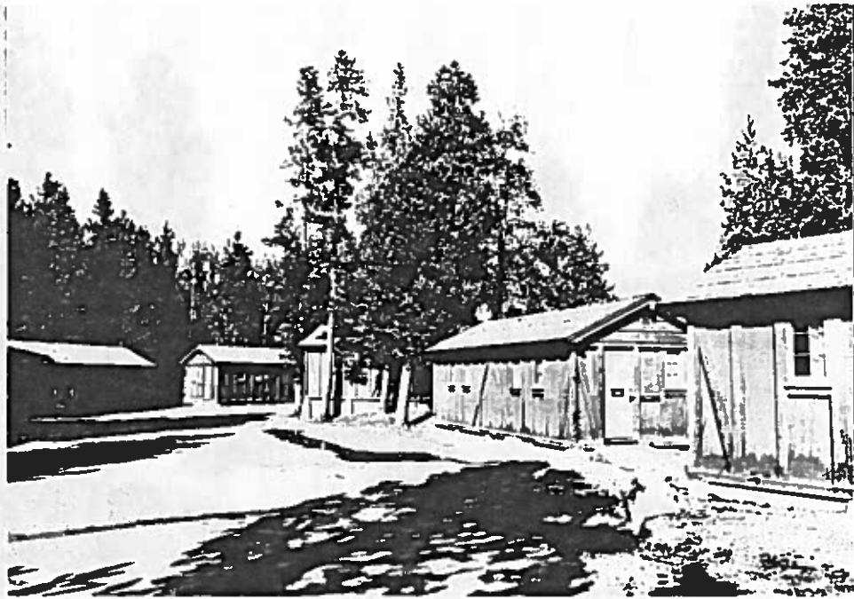
Figure 18: Looking north along the west roadway in the guest cabin area as it starts to turn east.
