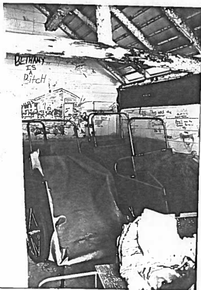
Figure 216: Looking at the interior of the upper loop linen building. Note the log interior with painted walls and logs.
