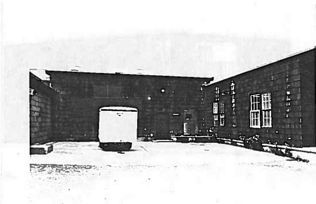
Figure 71: Looking at the infilled sections of original and added buildings tied together by the wood wall shingles. Note the weathering and staining of the wall material.
