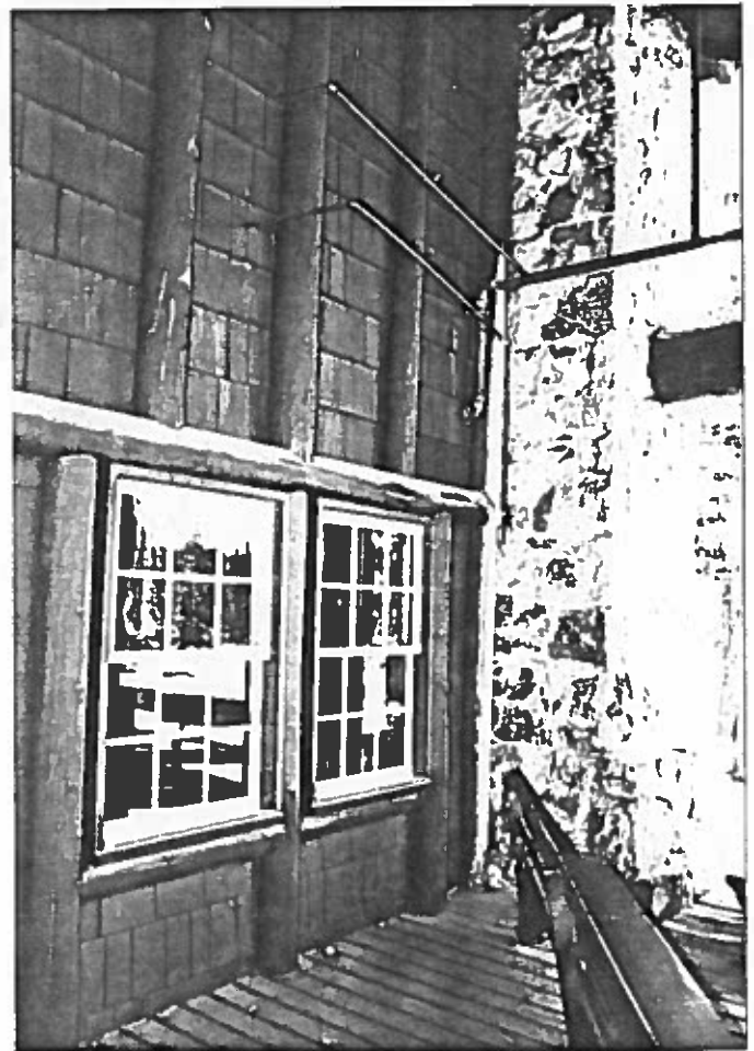
Figure 92: Looking northeast at some wood double-hung windows on the porch. The windows appear to be in good condition.
