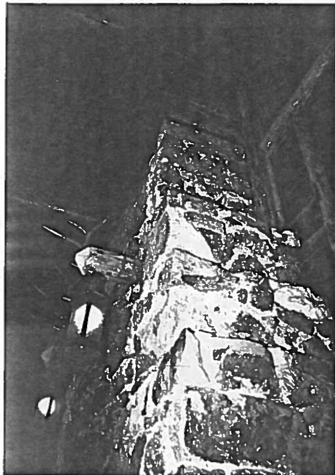
Figure 121: Looking northeast at a detail of the fireplace. The stonework with the exception of some mortar detailing is in good condition.
