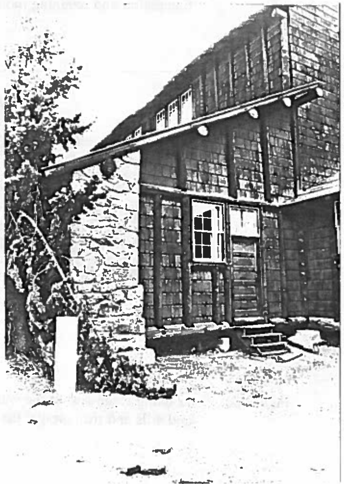
Figure 77: Looking southwest at the connection of the stage to the Rec Hall. All of the log roof rafters have been cut off at the eave line.
