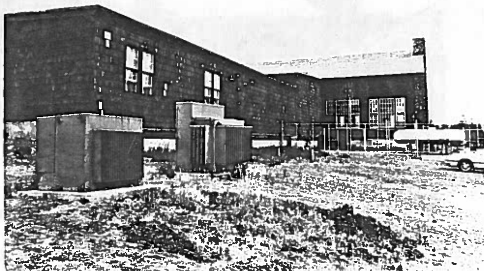
Figure 9: Looking west along the back side of the Old Faithful Lodge kitchen and employee dining area. Note the electrical transformers, and the propane tank area in the background. All of this faces the guest cabin area.
