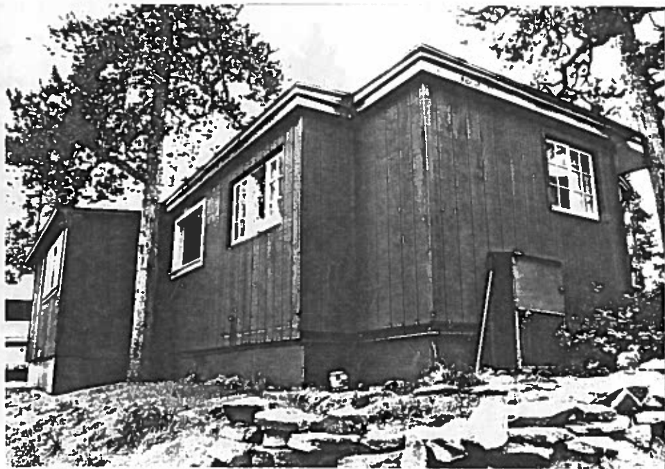
Figure 186: Looking south at the back of the maintenance managers cabin. Note the variety of windows and the shed roof additions.
