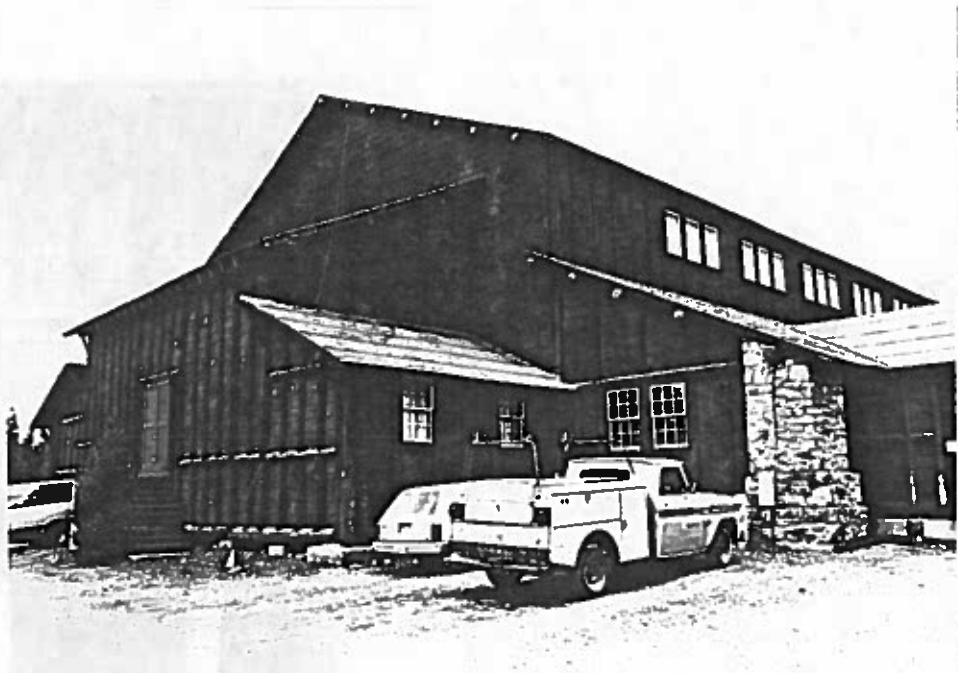
Figure 74: Looking southeast at the Rec Hall with the stage structure on the north end of the building. The log-out structure appears to be in good condition. There is minor rot and checks and weathered logs on the purlins, and in some of the sill logs.
