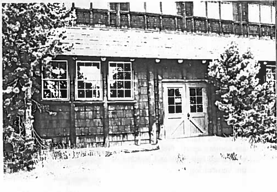
Figure 83: Looking west at a second set of doors on the east side of the Rec Hall. Note the weathered wood along the base and the close trees. The log rafter tips have been cut off on this side of the building also.
