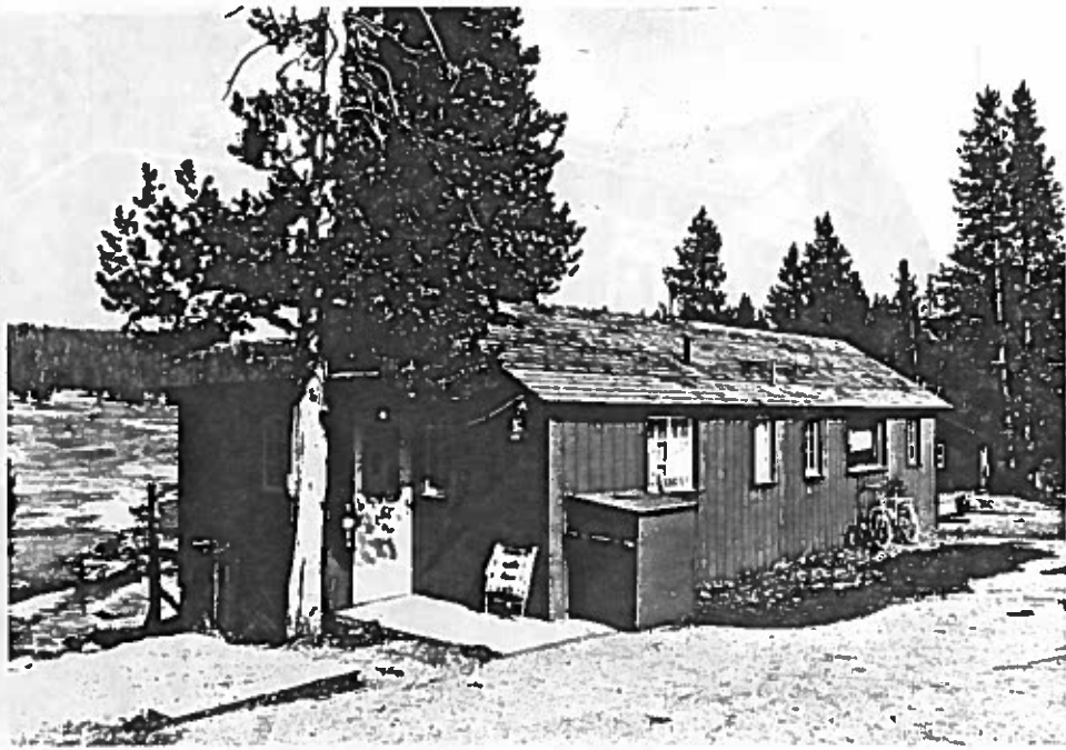
Figure 185: Looking east at the maintenance managers cabin. Note the texture 111 siding.
