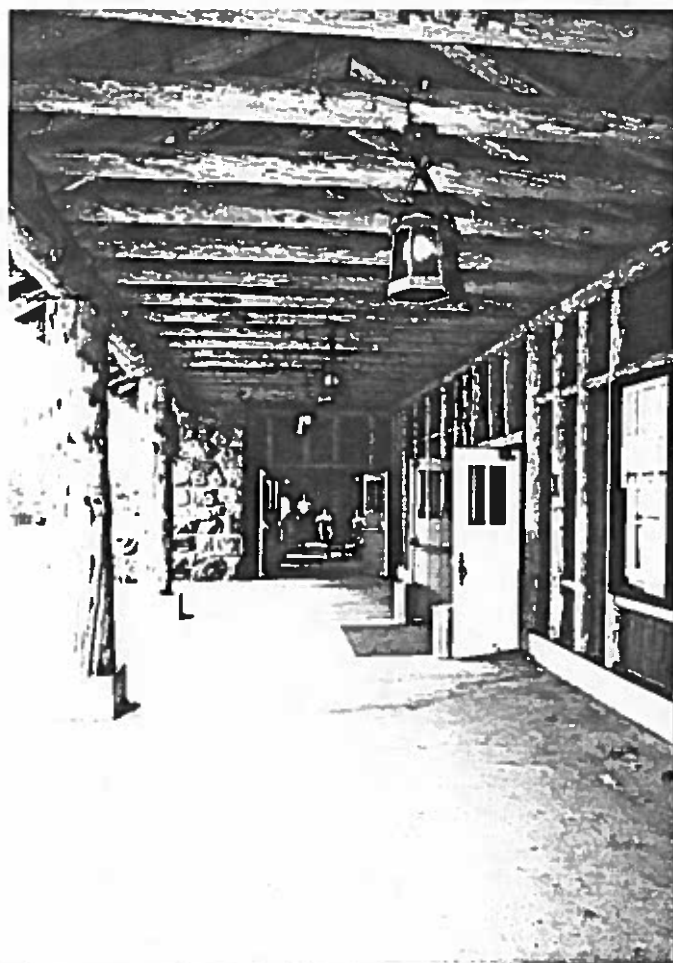
Figure 110: Looking north at the covered walkway along the west side of the building. Note the original light fixtures and wiring. The materials on this end of the building are in good condition.
