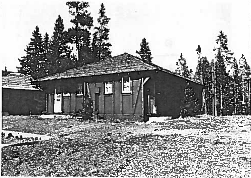
Figure 174: Looking northeast at a typical frame-out quad employee cabin (#417-420). These buildings appear to be in good condition.
