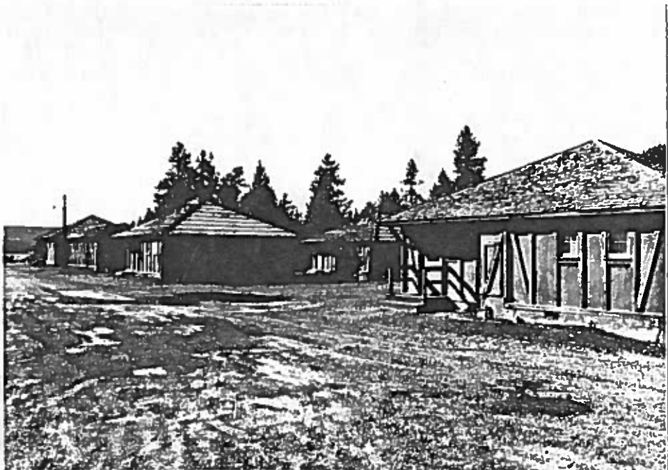
Figure 11: Looking northwest at the guest cabin area from the boiler building at Old Faithful Lodge. Note the little vegetation in this area.
