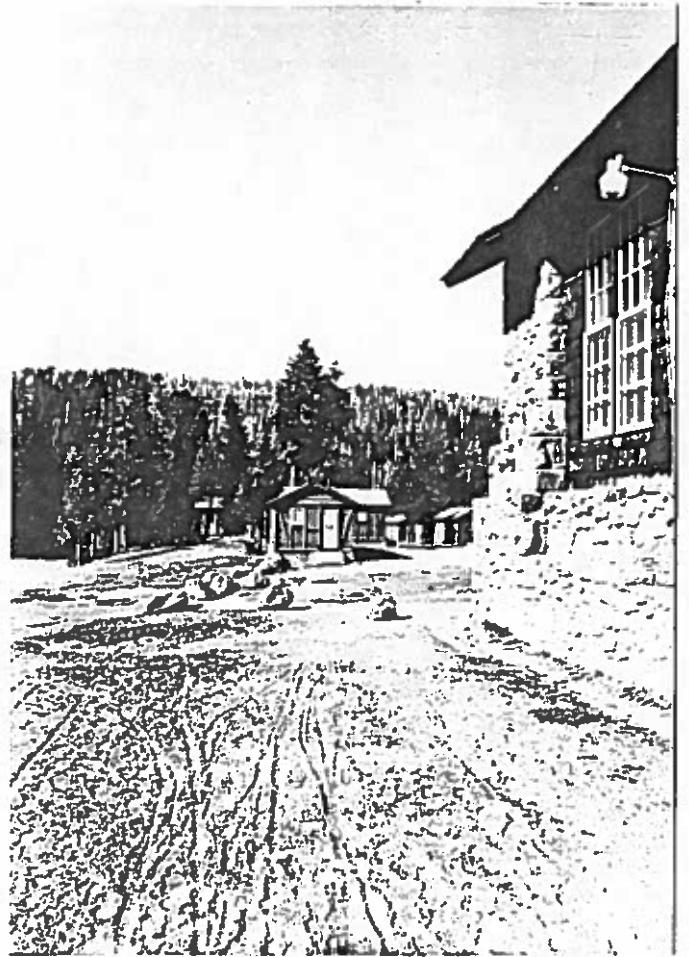
Figure 14: Looking north along the west side of Old Faithful Lodge towards the guest cabin area. Note the rocks that have been put out to discourage traffic along this side of the building. Also, note the wheel tracks from bicycles, and automobiles along this side of the building.
