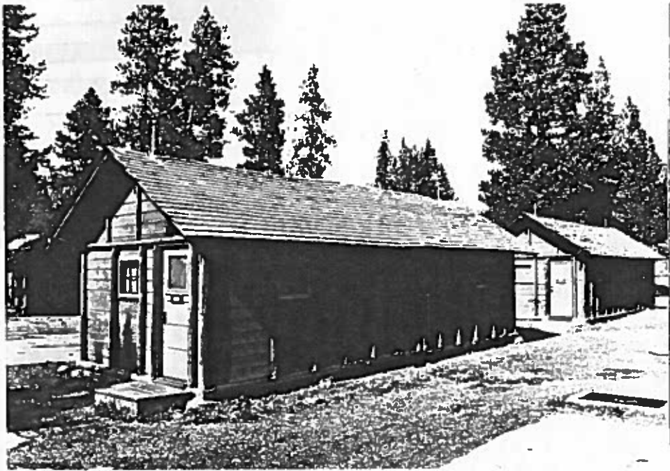
Figure 180: Looking northeast at a typical log-out duplex cabin (#236-237). This cabin is in good condition with the exception of some sill log rot and some rot in the wood stoop.
