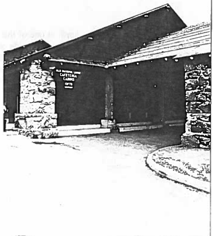
Figure 104: Looking northeast at the porte-cochere. The roof is in good condition and the log purlins have been capped with metal.
