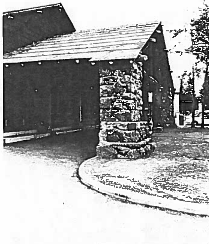
Figure 105: Looking east at the porte-cochere. The stonework is in good condition.
