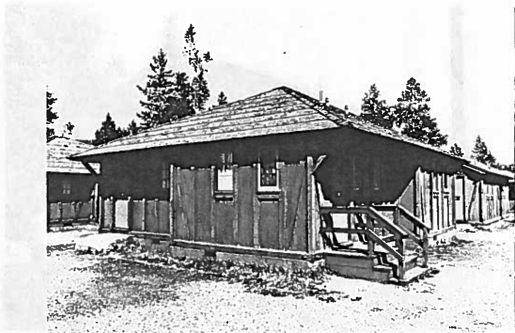
Figure 168: Looking northeast at a typical frame-out quad cabin (#110-113). Note the deteriorated concrete stoop which occurs on over thirty cabins in the area. The sill plate is weathered and is showing some rot in a few areas.
