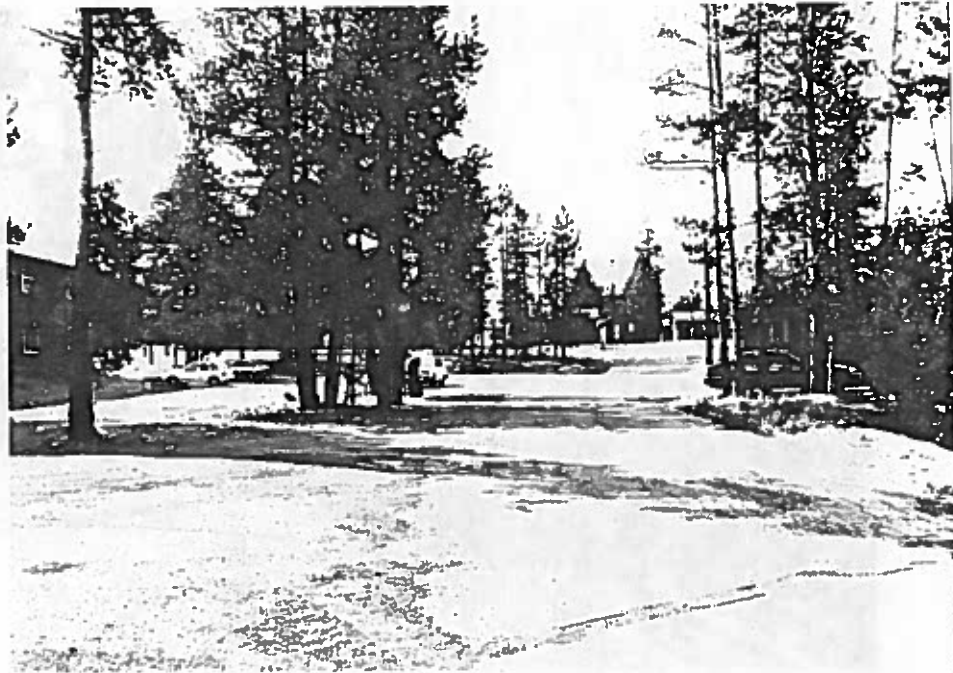
Figure 26: Looking west back towards the upper guest cabin area from the employee area to the east. Note the dormitory building with a large parking area on the left and employee cabins and parking on the right.
