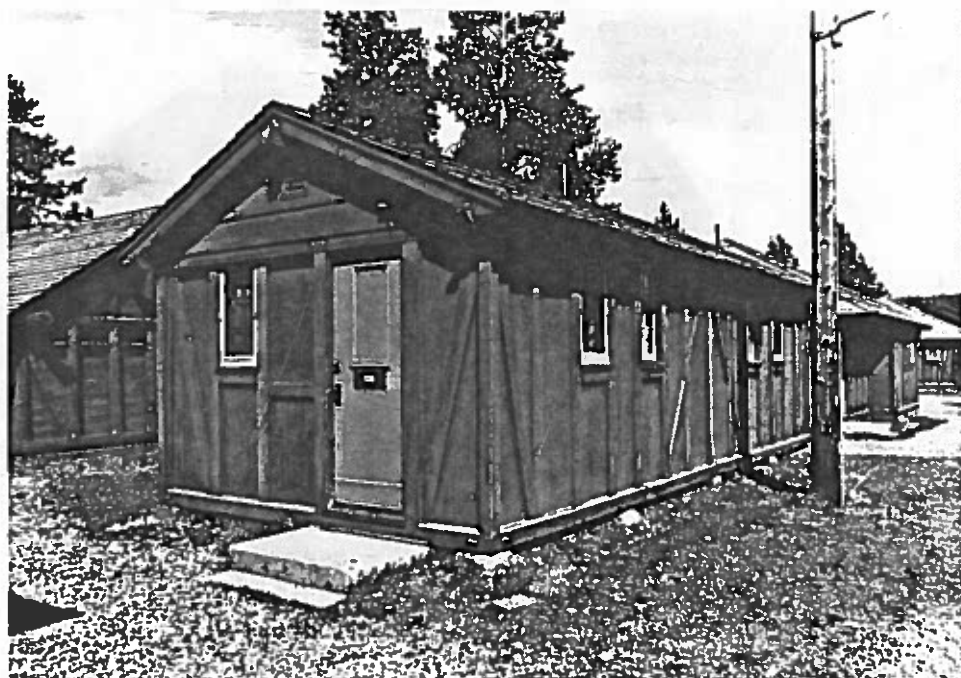
Figure 165: Looking northeast at a typical frame-out duplex cabin (#108-109). The cabin walls are dry and weathered.
