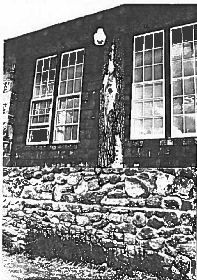
Figure 57: Looking east at the window bays on the north end of the west side of the Lodge. Some minor missing mortar occurs on this elevation. Note the lost bark on the column with the light fixture that allows water to penetrate into the bark area.
