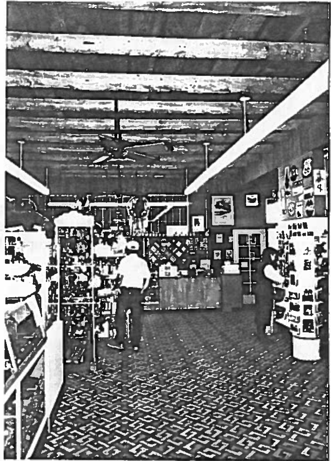
Figure 131: Looking east at the gift shop. Generally the logs appear to be in good condition.
