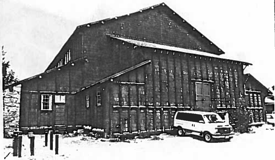
Figure 77: Looking southwest at the connection of the stage to the Rec Hall. All of the log roof rafters have been cut off at the eave line.
