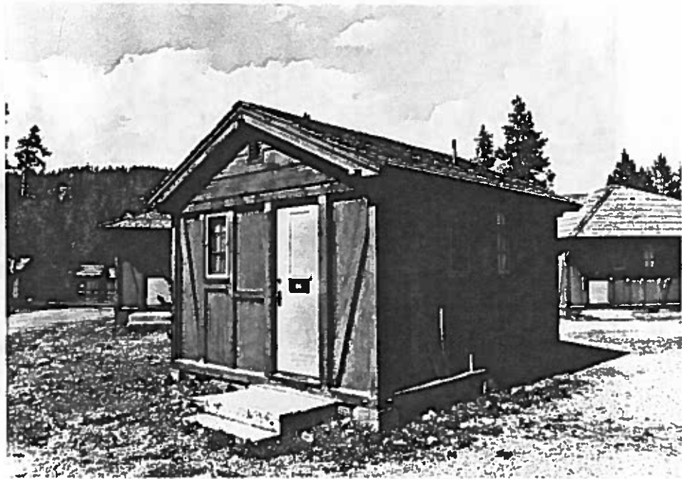
Figure 162: Looking north at a typical frame-out single cabin (#114). This building is in good condition with some minor rot on the sill plate. The siding and frame is dry and weathered.
