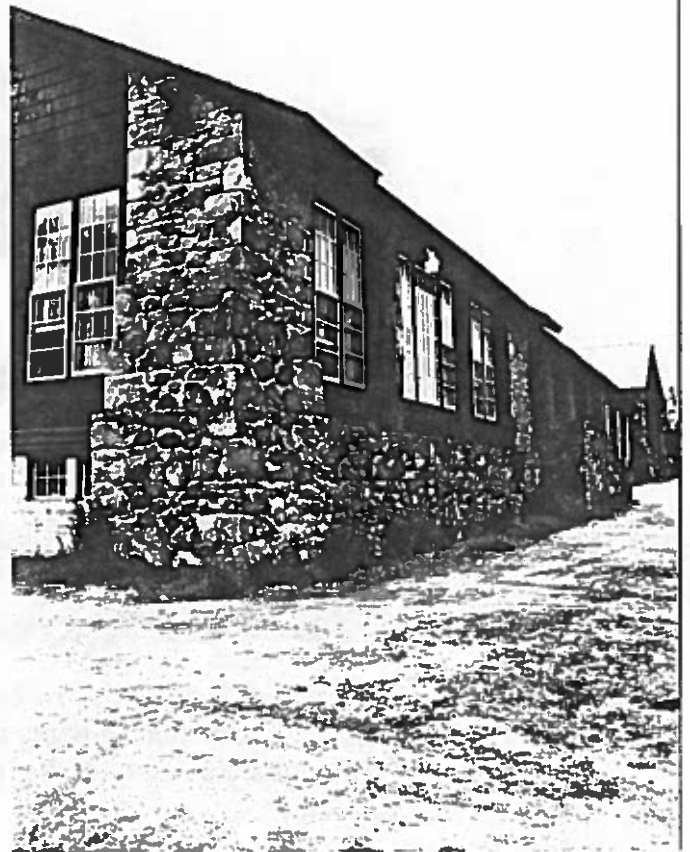
Figure 59: Looking northeast at the corner stonework. The stonework is generally in good condition.
