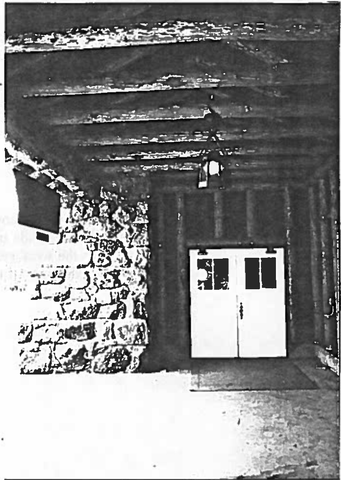
Figure 111: Looking north at the doors into the main public spaces of the Lodge. The doors with some minor wear and tear are in good condition.
