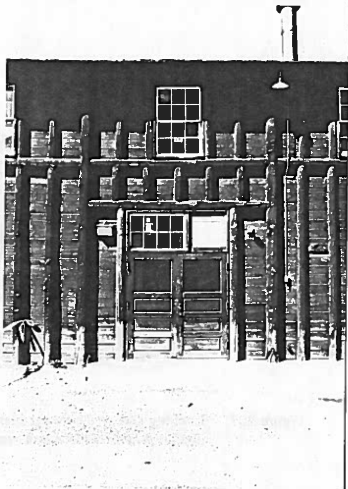
Figure 205: Looking north at the entrance doors on the Boiler Plant building. Note the weathered bottom panels on the doors and the base of the walls.
