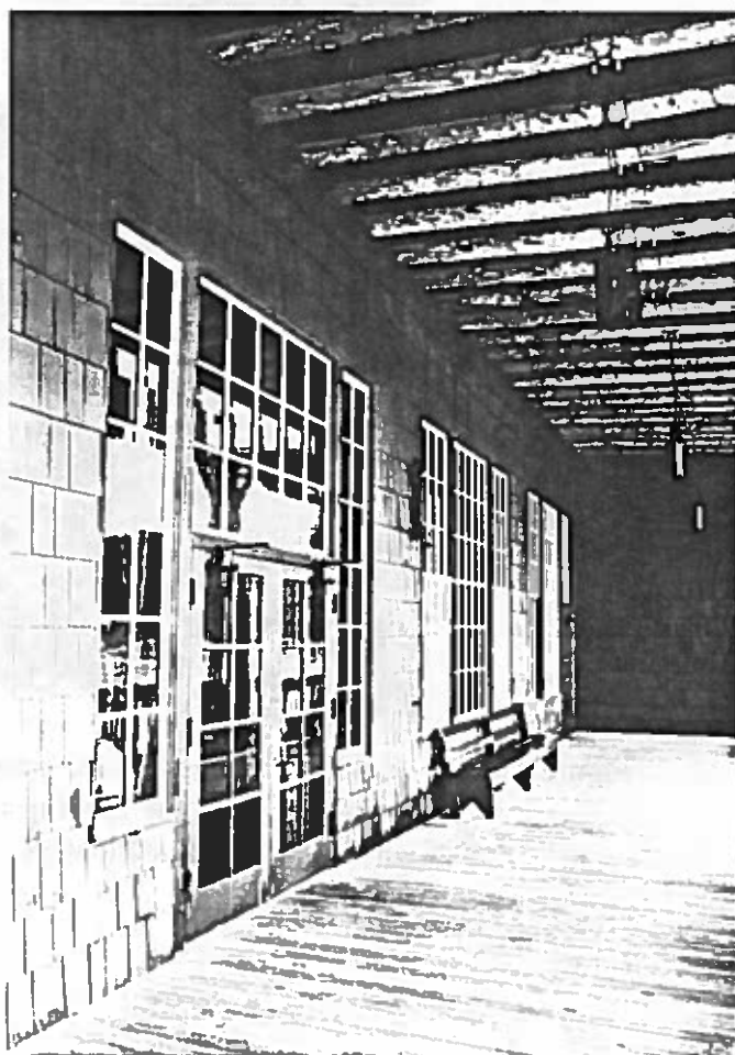
Figure 54: Looking southeast at the exit doors from the cafeteria onto the porch. Other than minor wear and tear these doors are in good condition. Note the light fixtures that appear to be original. The knob and tube wiring still exists in many areas.
