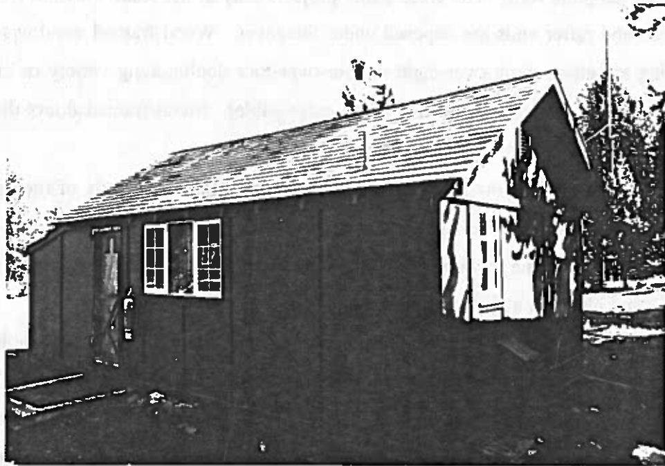
Figure 189: Looking south at the "love nest" cabin. The walls are plywood with battens over the joints. A bathroom has been added to the back.
