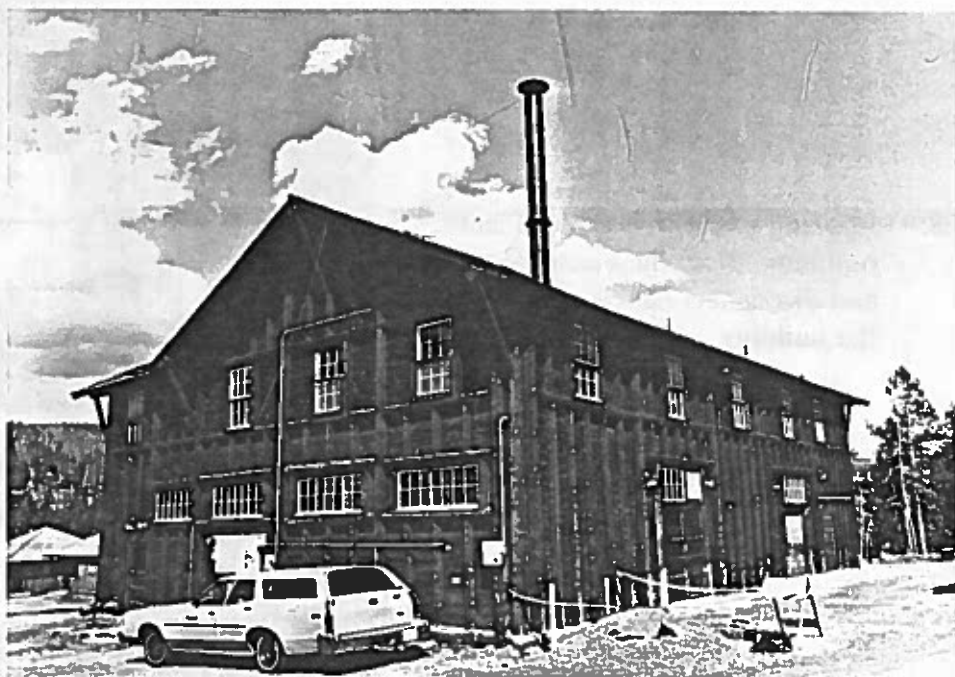
Figure 206: Looking northeast at the Boiler Plant building. The wall logs other than the bases appear to be in good condition.
