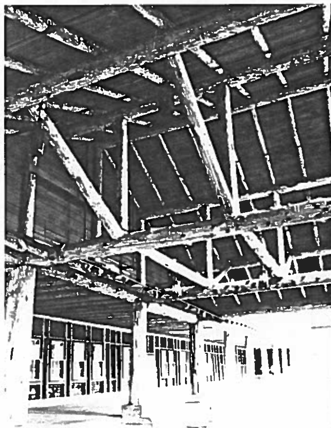
Figure 106: Looking east at the structure logwork of the porte-cochere. The logs are in good condition. There are original light fixtures up in the ridge.
