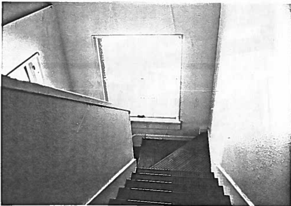
Figure 199: Looking at the interior of the stairway on the Dormitory building. Note the white painted sheetrock walls.
