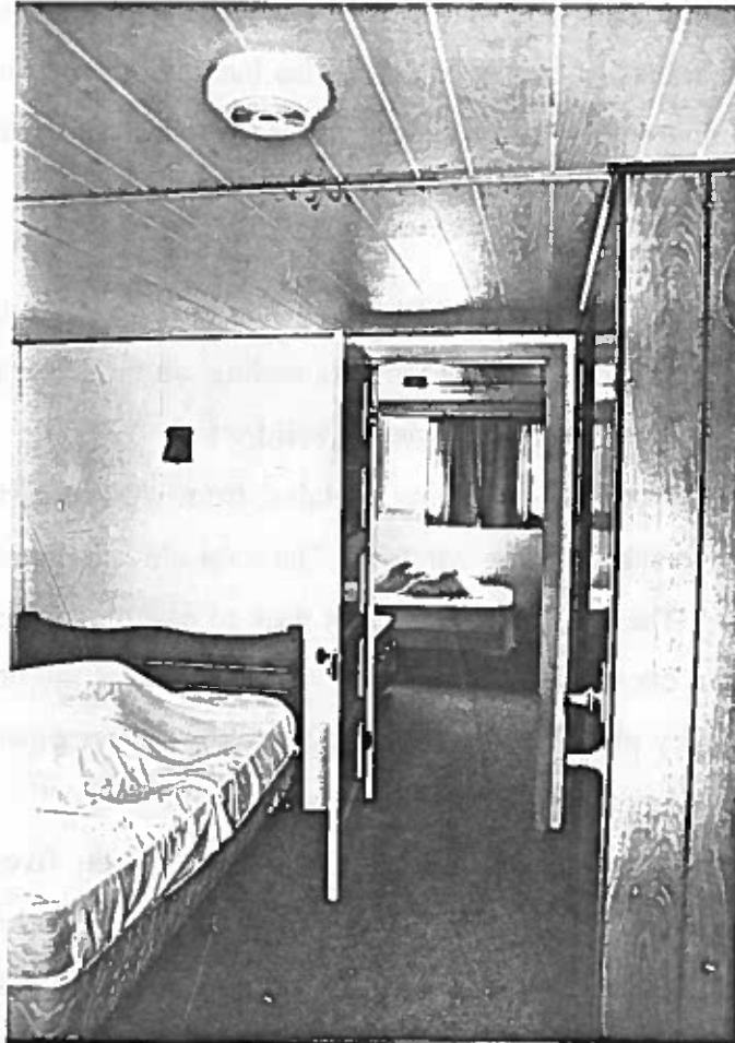
Figure 184: Looking at a typical log-out duplex cabin, (#234), interior. Note the wood paneling on the walls and ceiling with some of the paneling painted white.
