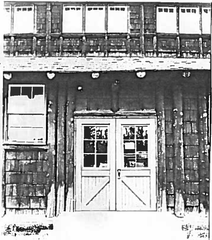
Figure 81: Looking west at the exit doors on the east side of the Rec Hall. The doors have been damaged by loading and unloading of materials to the Rec Hall. The base panels are coming apart. Note the weathered base logs and bottoms of the vertical logs.
