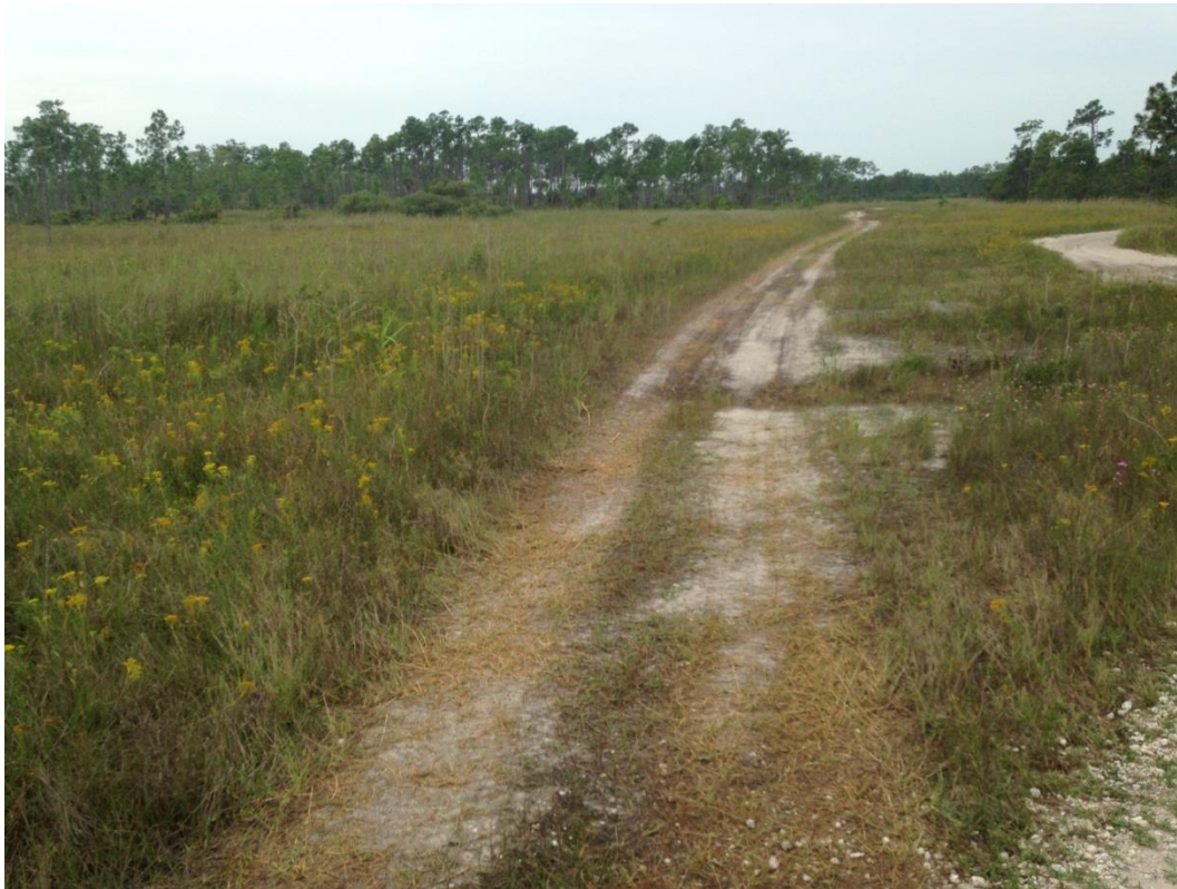
Buckskin Trail, braiding and fresh material pushed outside of tread
