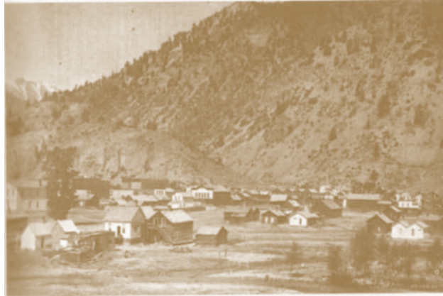
Cristobal. The Red Mountain Gulch Day Area did not exist at that time.
