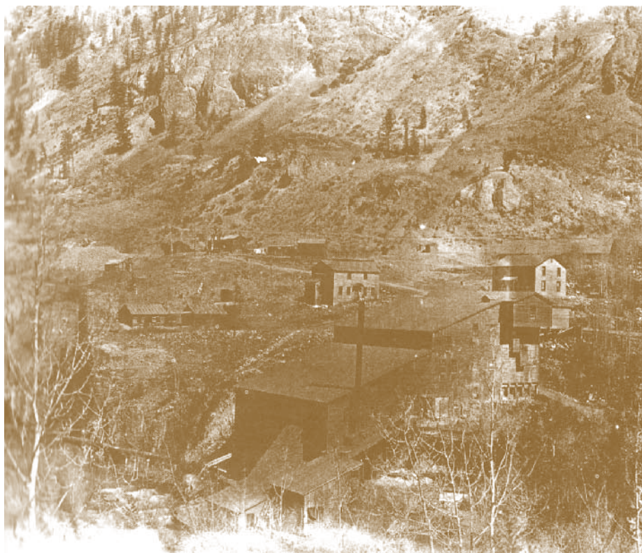
Hidden Treasure Mill, Office, and Bunkhouse. Courtesy of Tiny Hinsdale of The Silvery San Juan by Carolyn and Clarence Wright
