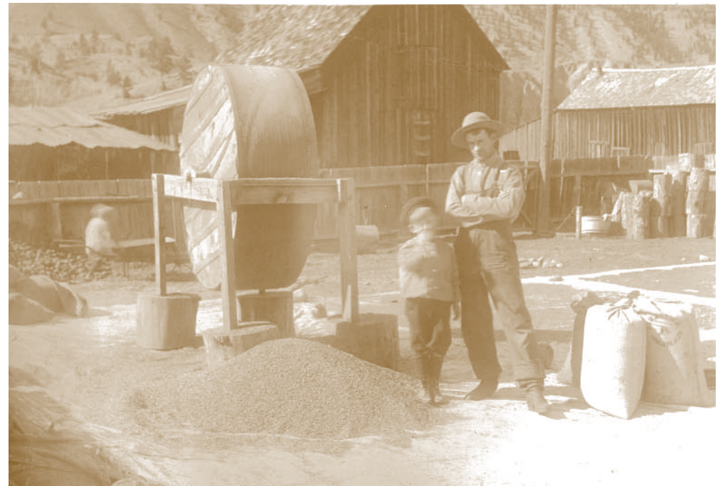
Seed extractor or cone tumbler. Open cones are placed into the extractor; then the drum is turned over, shaking the remaining seed out of the cones. There may be paddles inside the drum to knock the cones around more. The seed being smaller in size than cones will fall to the bottom of the drum. Most seed extractors should have a screen on the outside of the drum which allows the seed to fall through and out while keeping the cones and larger debris in. On the photographs, the detail of the screens and fill/empty hatches is not readily apparent. Bushel bags are the common unit of measure for cones. Contractors were paid by the bushel for collected cones. Extracted seed is usually measured by the pound. Bags on the right appear to be filled with clean seed, which is the end product of the process.
