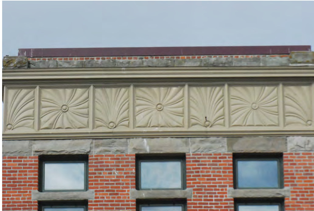
CITY HALL CORNICE PANELS
