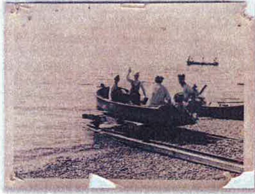
Launching a Cama Beach 40/50 Series with marine railway ca. 1950. Cama Beach 20 Series type boats visible in the background. Courtesy of the Stanwood Area Historical Society
