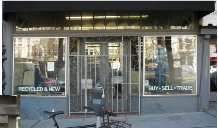
Figure 1: Eastern storefront: 2117 Market Street
