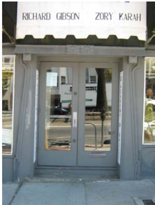
Figure 11: Entry doors to New Era Hall rooms from Market Street
