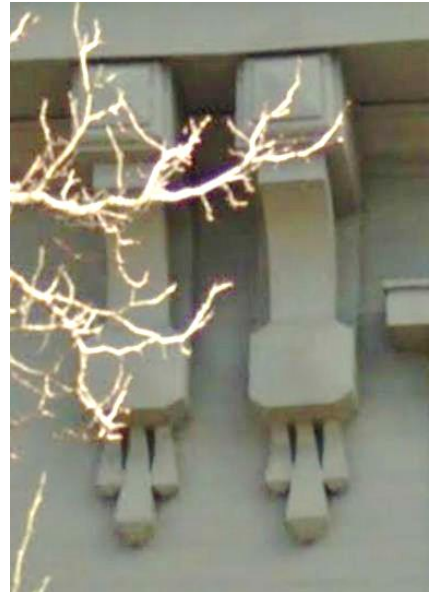
Figure 12: Secessionist pendants below brackets
