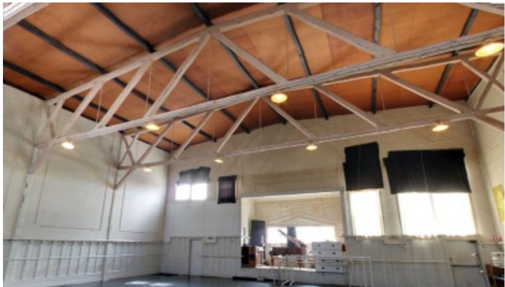
Figure 7: Interior of Lodge Room No. 1 with exposed Howe Trusses. (Google Maps)
