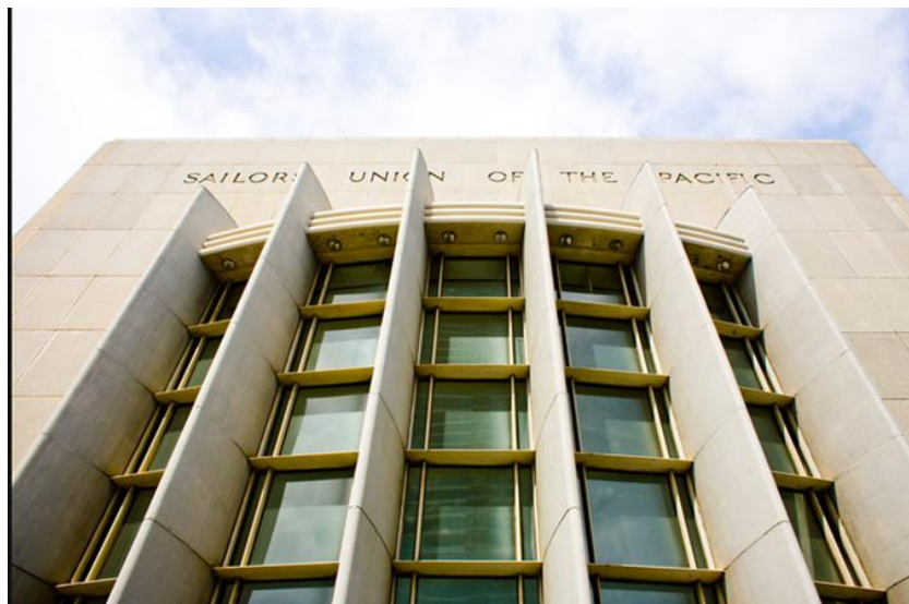
Above: Detail of window wall entrance. Source: Thomas Hawk, Flickr.com
