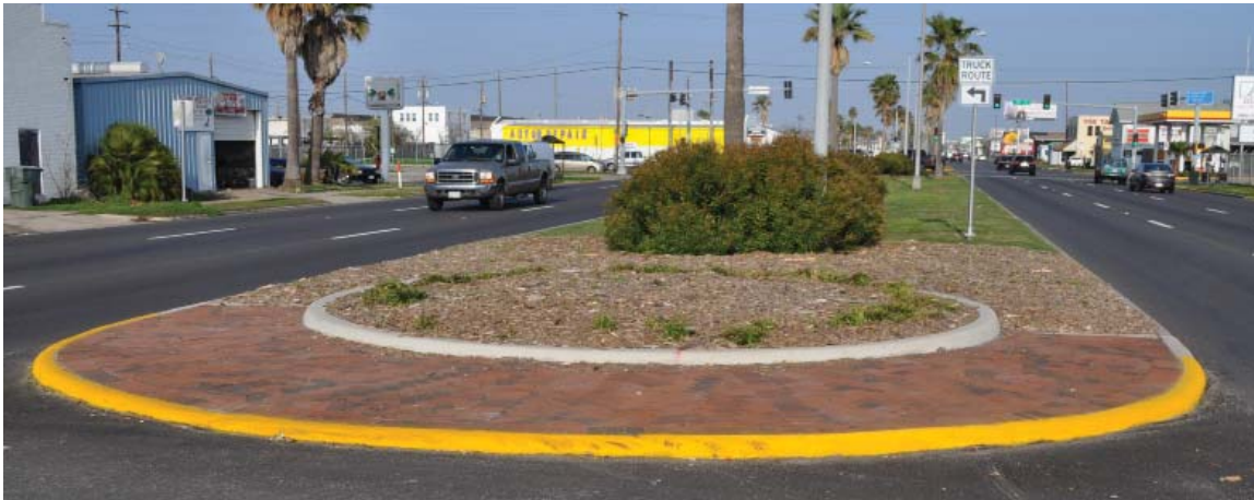
This circular, curbed planting bed is typical of every segment of the median.
