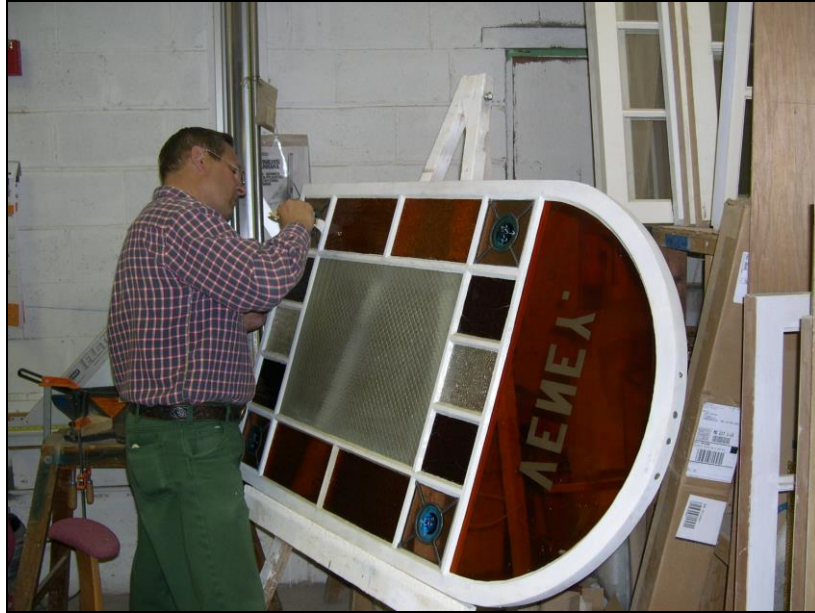
Photo 7: Painting the sash
