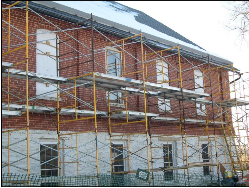
Photo 1: First floor sash were removed and temporary enclosures were installed
