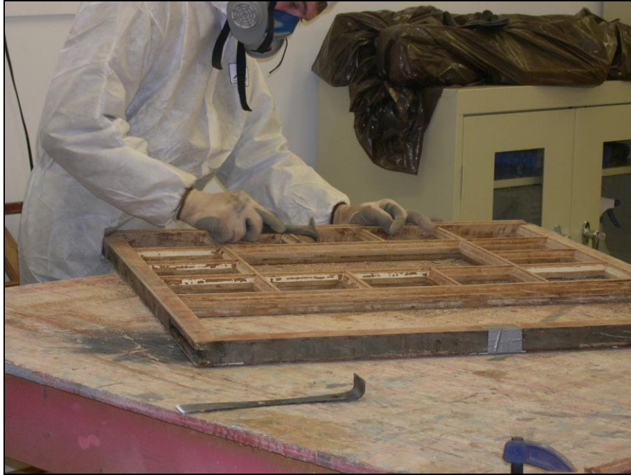
Photo 3: Lead paint being scraped from the sash at our Jenkins facility
