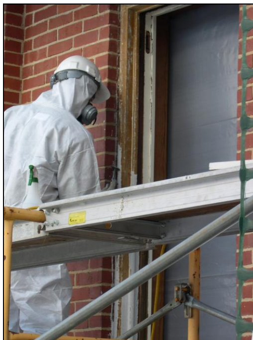
Photo 6: Scraping paint from the window jambs
