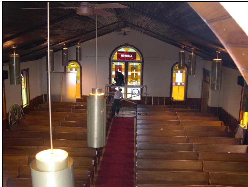
Photo 8: Installing the east elevation windows
