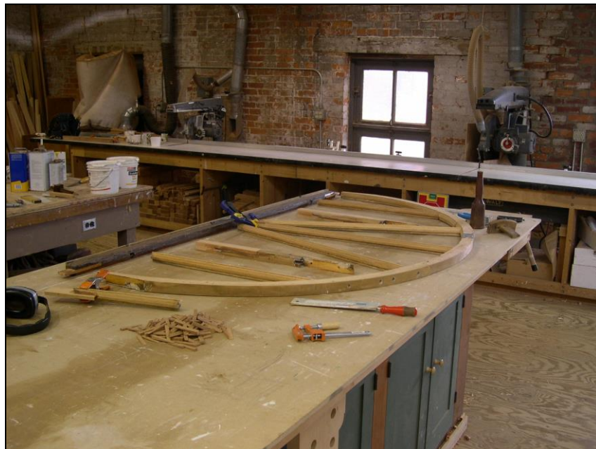
Photo 4: Carpentry repairs to the west elevation lunette
