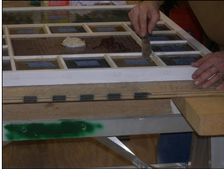
Photo 5: Glazing the sash
