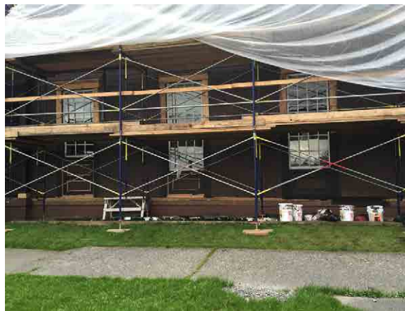
The bottom section of the building about to be painted.
