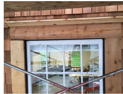
New header installed over the windows.
