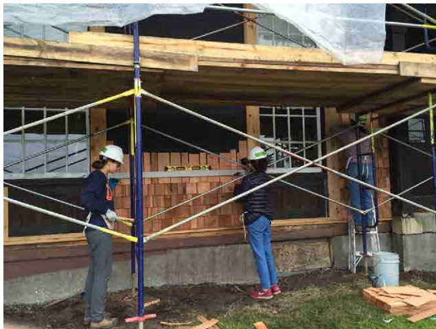
Interns putting on new cedar shingles.
