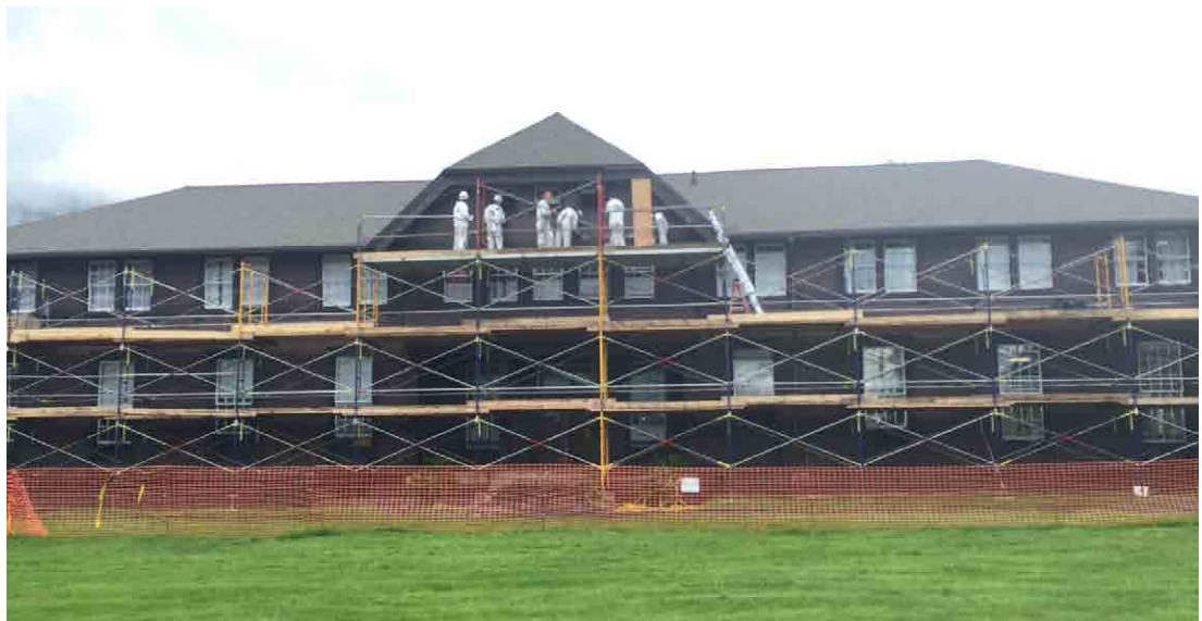
Interns painting the last few spots on the top floor of the scaffolding.
