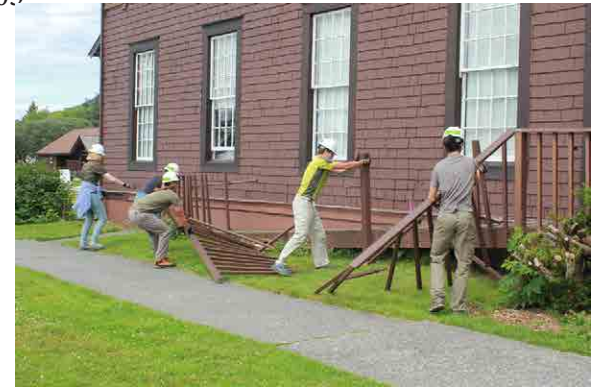
Interns removing the ramp that was on the left side of the porch.
