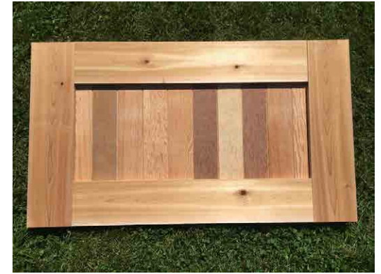
The panel that was fabricated to be installed under window G as the original was missing.
