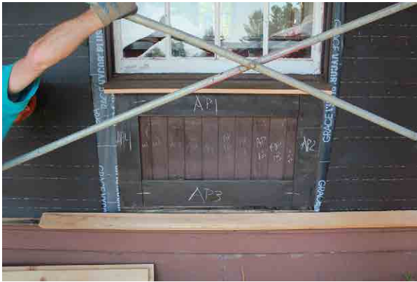
Vycor and 15 lbs Felt have been installed around Window A.
