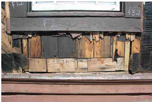
Boards that covered many hidden panels underneath all windows. [Window F]
