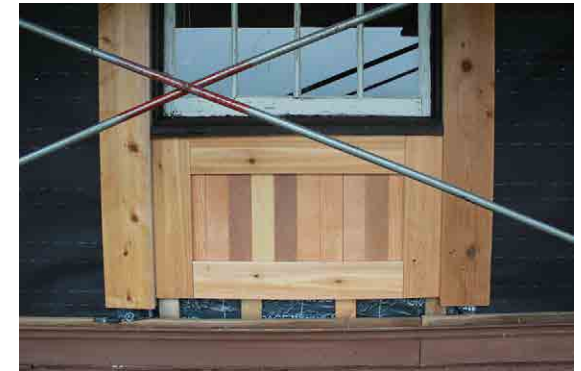
The new panel and casings have been installed for Window G with Vycor and 15 lbs Felt.
