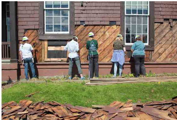
Interns removing old cedar shingles and nails.
