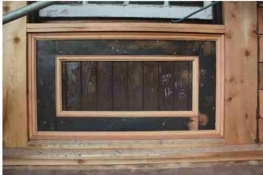
Window panel with new moulding.
