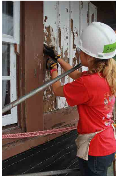
Intern Avery scraping old paint.
