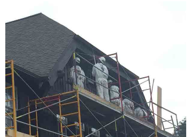
Interns painting the very top of the building.
