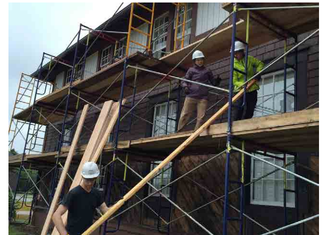
Interns erecting the scaffolding.
