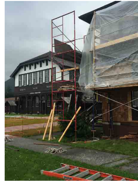
Scaffolding that was erected on the west side of the building.
