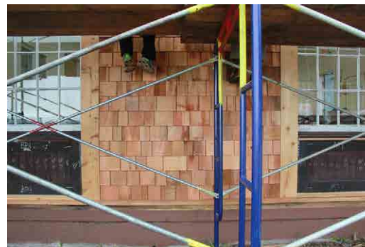
Interns putting on new shingles on the second level of scaffolding.
