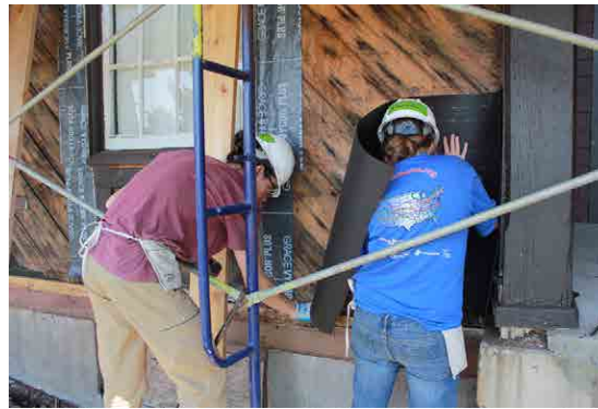
Interns installing a section of 15 lbs Felt.
