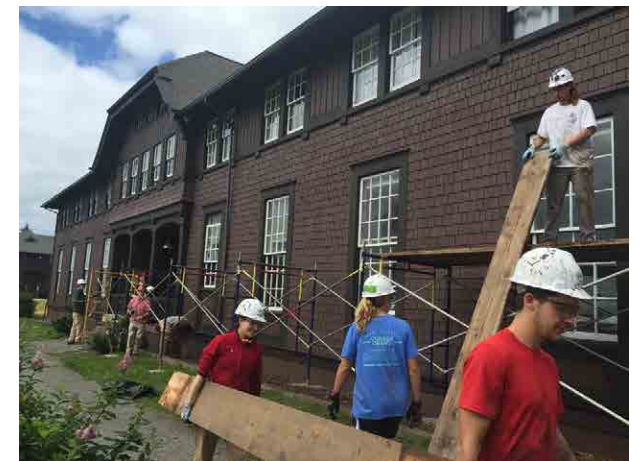
Interns disassembling the scaffolding.
