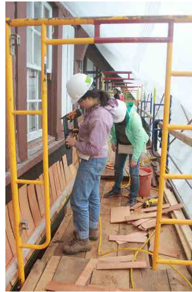
Interns Minah and Amanda shingling a section above the porch.
