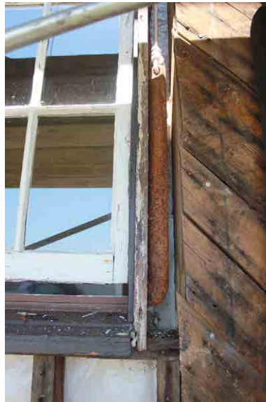
A window sash that was hidden beneath a casing.
