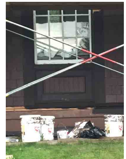
Paint supplies and a partially completed paint job.
