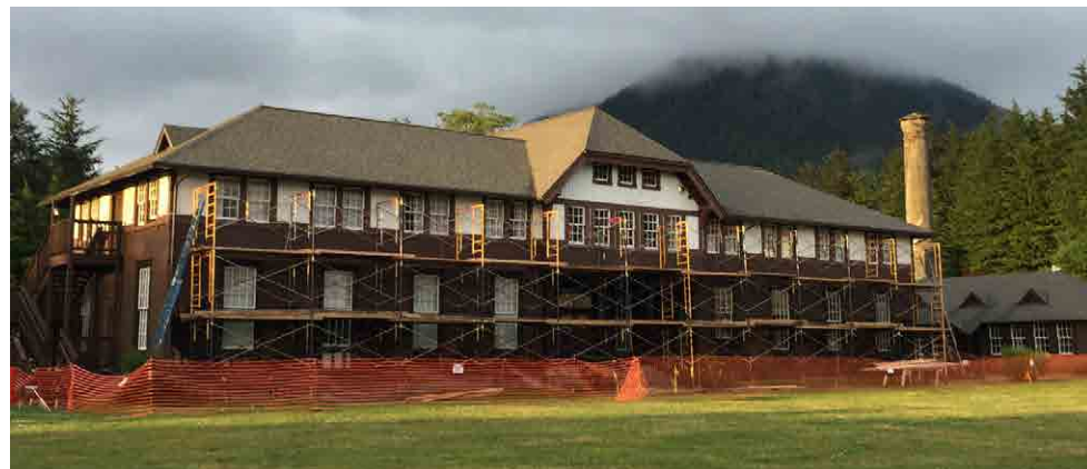
Scaffolding completely erected.
