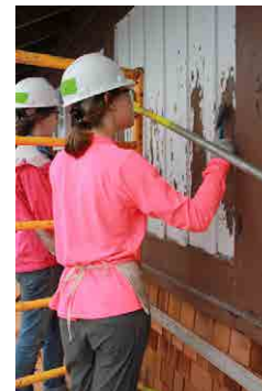
Interns Emily and Eve scraping old paint.
