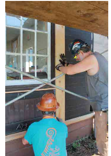
Larry and Pete raising the drip-cap and making sure the casing fits correctly.
