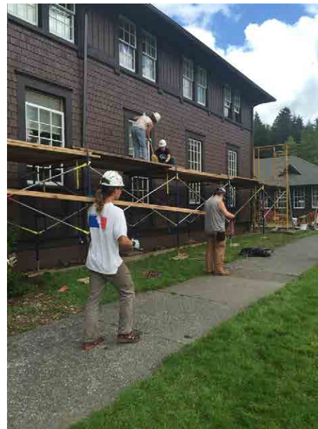
Interns disassembling the scaffolding.
