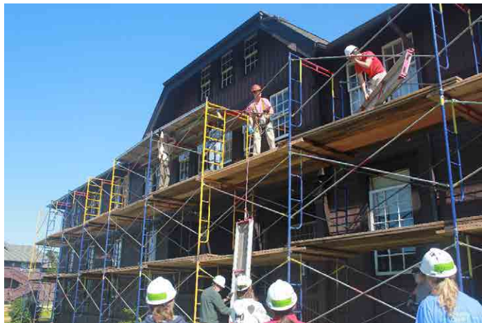
Interns disassembling the scaffolding.
