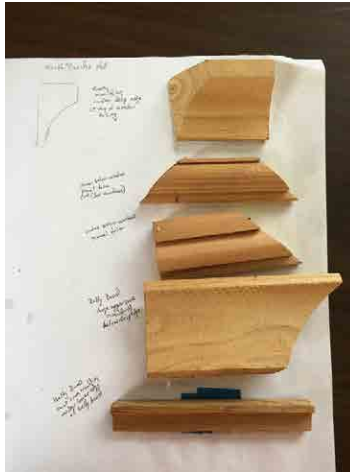
Samples of moulding from North Pacific Hall. The moulding created for under the drip-cap is the second from the bottom.
