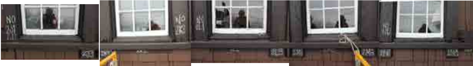
SECOND STORY WINDOWS, LABELLED, PRE SHINGLE REMOVAL
