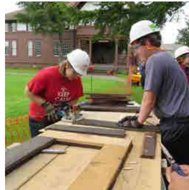
ANNA PIWOWAR AND NATHAN HENRY CUT HOLES INTO THE PANEL FRAMES TO PREPARE FOR ASSEMBLY
