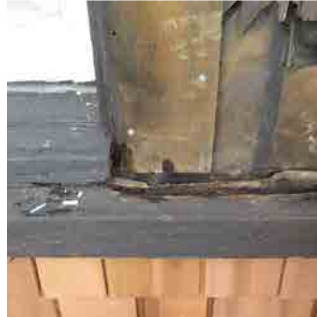
EPOXY IS APPLIED TO ROT-DAMAGED ORIGINAL WOOD PIECES
