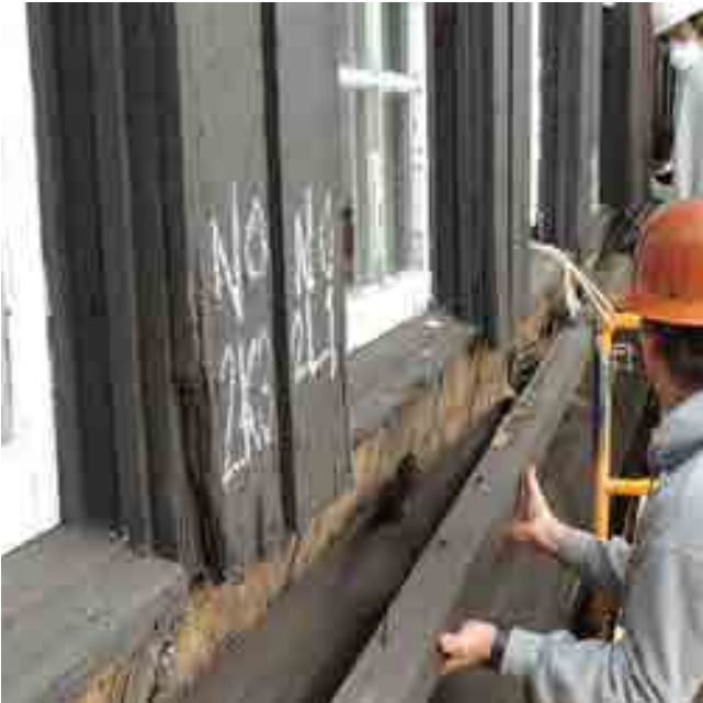
REPLACING WOOD TRIM
