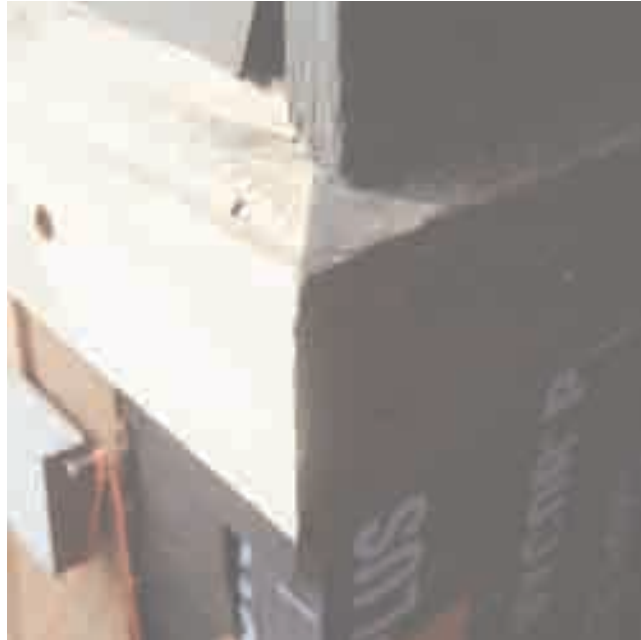
(DAY 13) A NEWLY FABRICATED PIECE OF TRIM MEETS AN ORIGINAL THAT DID NOT REQUIRE REPLACEMENT
