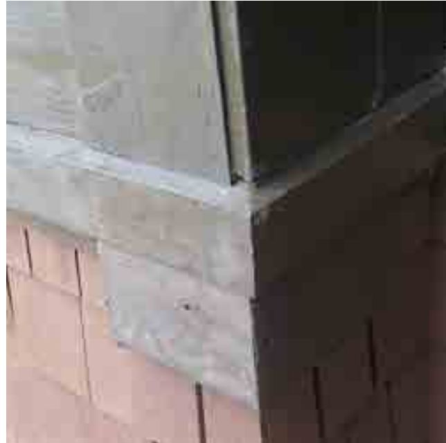
FRESHLY PAINTED, WITH NEWLY FABRICATED BLOCKS BENEATH, THE OLD AND NEW TRIM ARE SEAMLESSLY CONSTRUCTED TOGETHER
