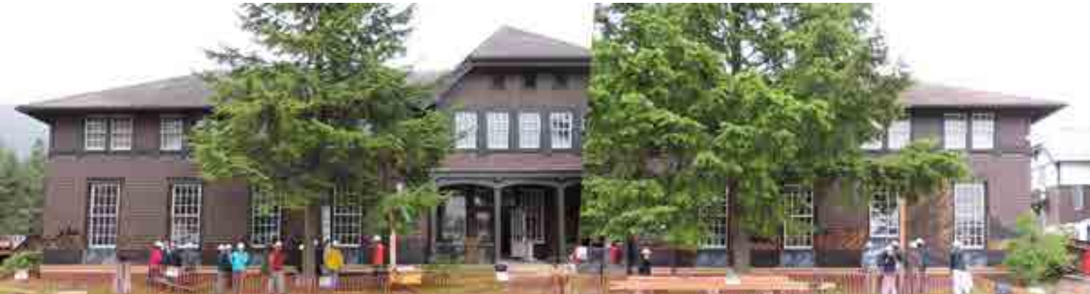
WATERPROOFING INSTALLED AT FIRST LEVEL
