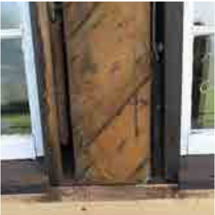
6X1S REMOVED TO WATERPROOF AROUND WINDOWS
