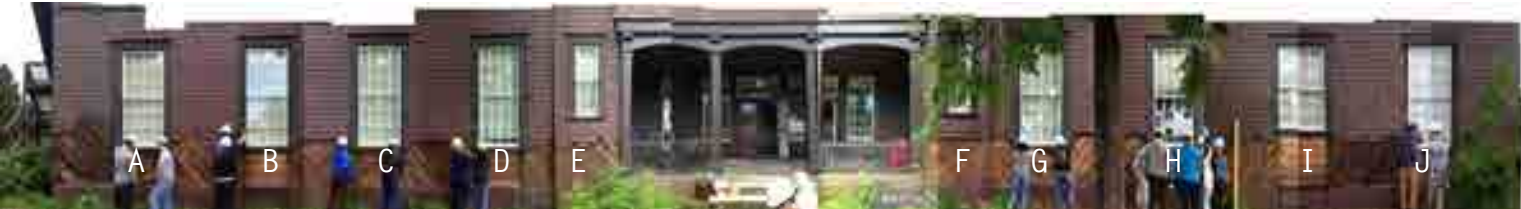
FRONT ELEVATION WITH ORIGINAL SHINGLES AND WATERPROOFING REMOVED.
