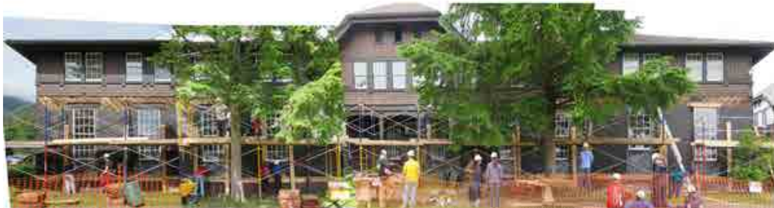
SHINGLES AND CASINGS REMOVED, TAR PAPER CUT AND STAPLED INTO PLACE UP TO MOLDINGS
