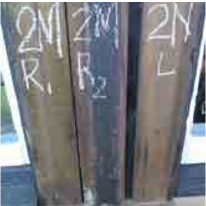
DAMAGED CASINGS REMOVED TO REVEAL 6X1 BOARDS, 61” LENGTH, WHICH WERE THEN LABELLED
