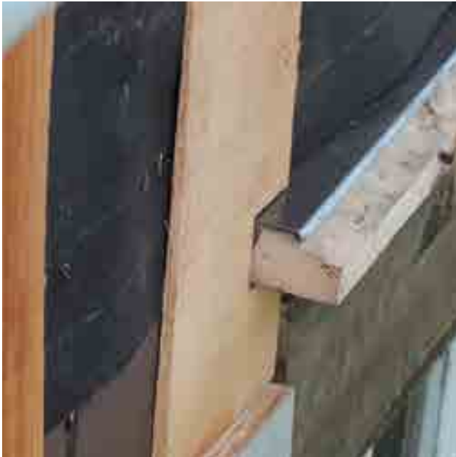
SHINGLES CUT TO FIT AROUND 2ST STORY WINDOW AND DRIP CAP. WATERPROOF TAR PAPER BELOW.
