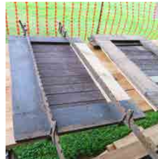
CLOCKWISE FROM TOP LEFT: PANEL REASSEMBLY ONSITE; HOLES ARE CUT INTO THE FRAMES FOR BISCUIT AND GLUE ASSEMBLY; PANELS ARE PIN NAILED TO THE FRAME; PANELS ARE FLIPPED AND CLAMPED IN PLACE DURING DRYING
