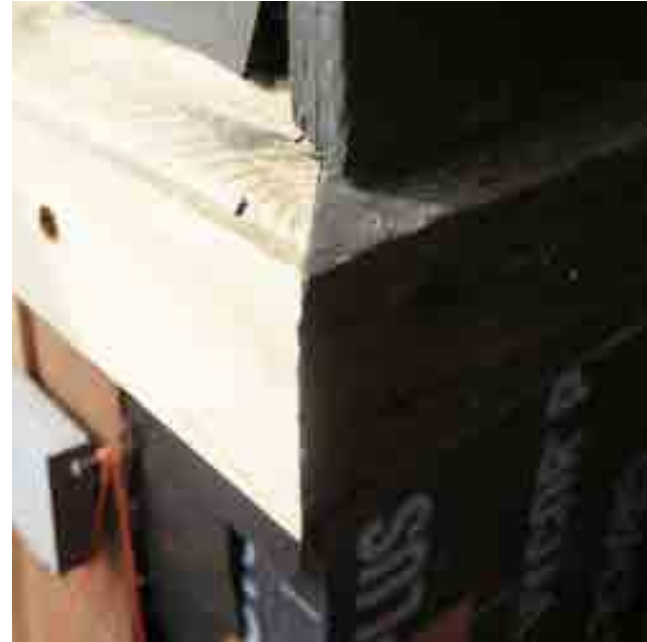
A NEWLY FABRICATED PIECE OF TRIM MEETS AN ORIGINAL THAT DID NOT REQUIRE REPLACEMENT
