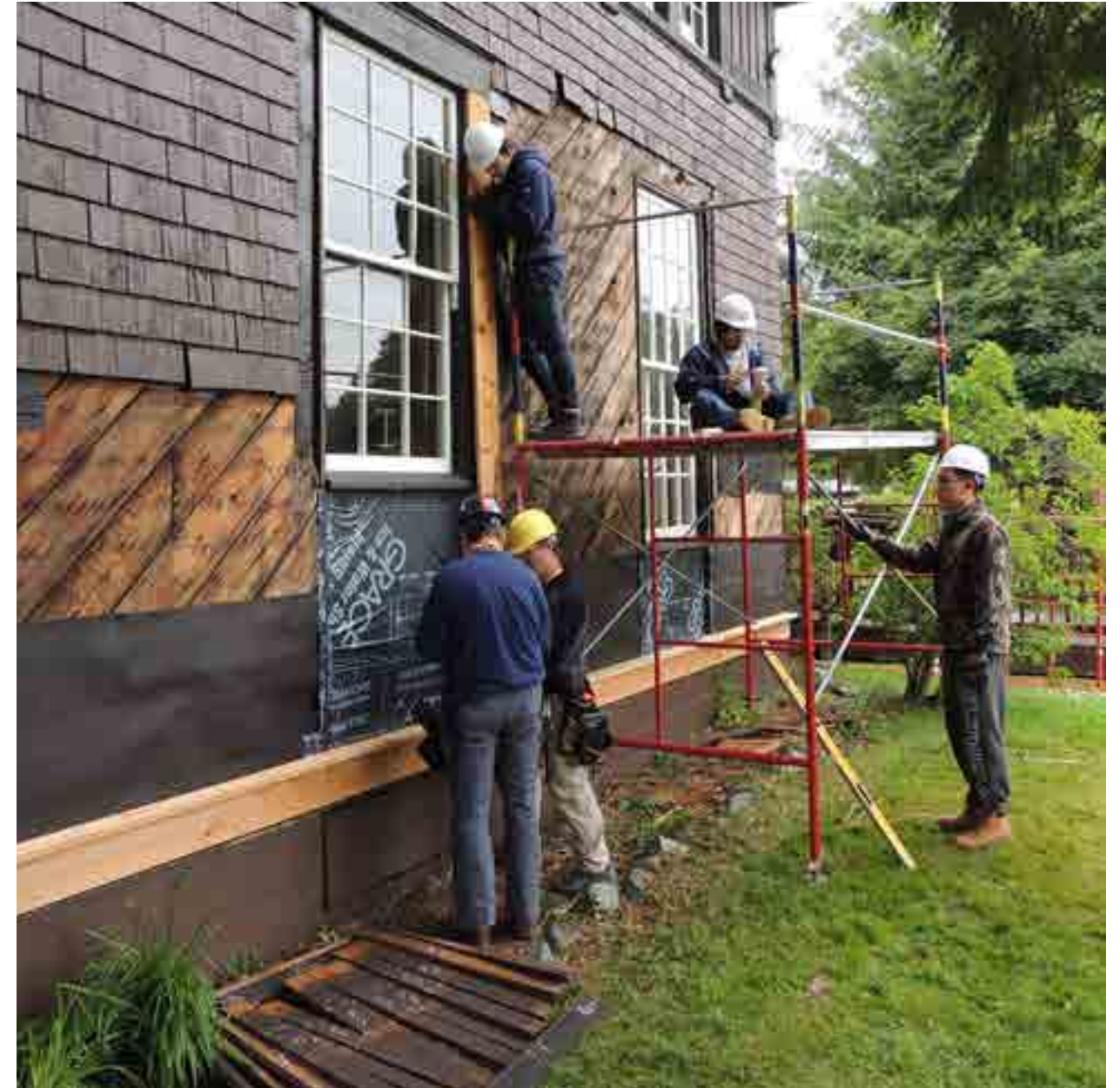
HRT MEMBERS ETIENNE DESBOIS, SAMIR WADHWANI, AND MIKE MCDONNELL WORK WITH LARRY JACKSON AND PETE WEILAND TO INSTALL WINDOW CASINGS.
