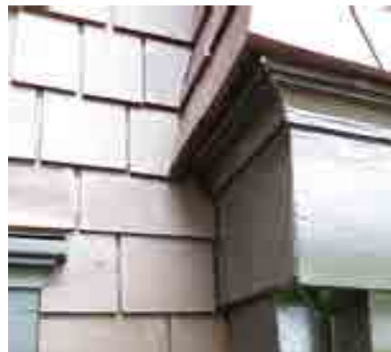
NEW SHINGLES MEET PORCH MOLDING
