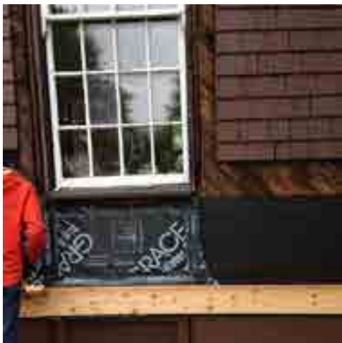
BELLY BAND INSTALLATION
