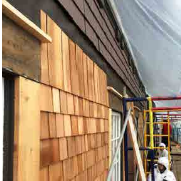
SHINGLE INSTALLATION REACHES TO TOP OF SECOND STORY WINDOW SILLS
