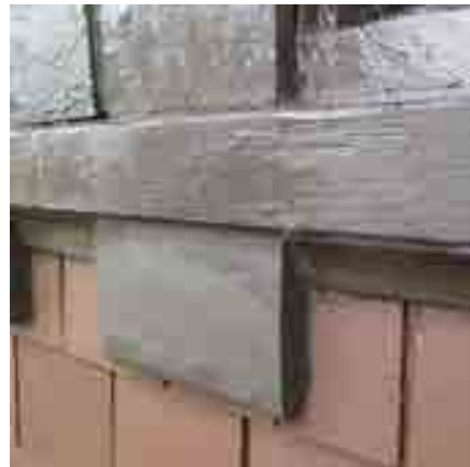
NEWLY FABRICATED BLOCKS BENEATH CASINGS
