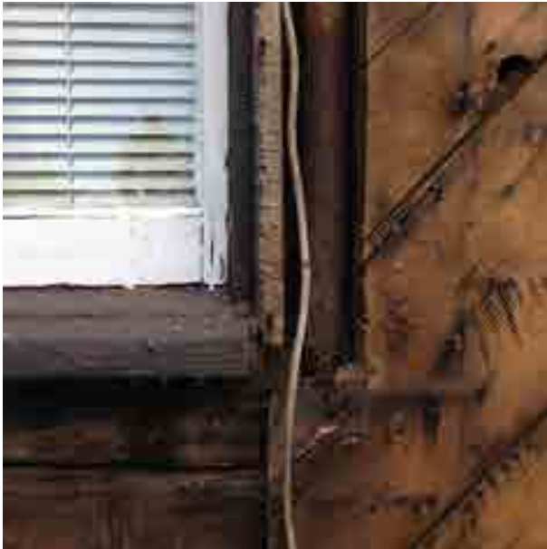
WINDOW SASH WEIGHT REPAIR: SASH WEIGHTS AND CASINGS REMOVED
