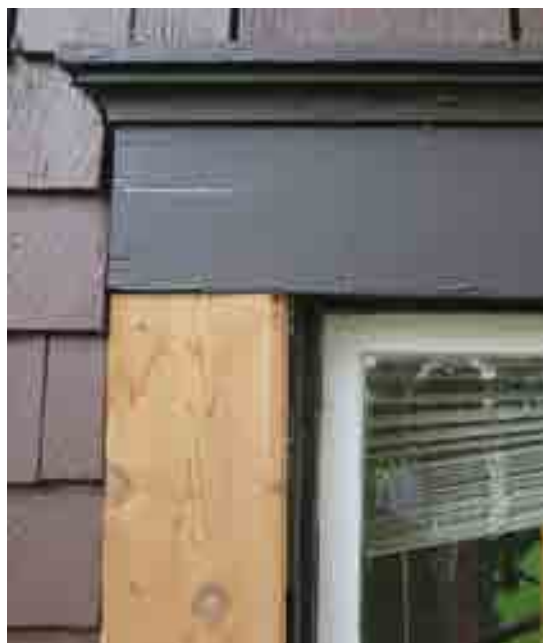
CHALK MARKERS ON THE WINDOW HEADERS TO NOTATE SHINGLE PLACEMENT BEFORE REMOVAL
