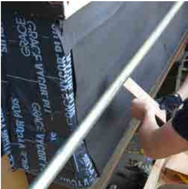
BEGINNING SHINGLE INSTALLATION ABOVE PORCH
