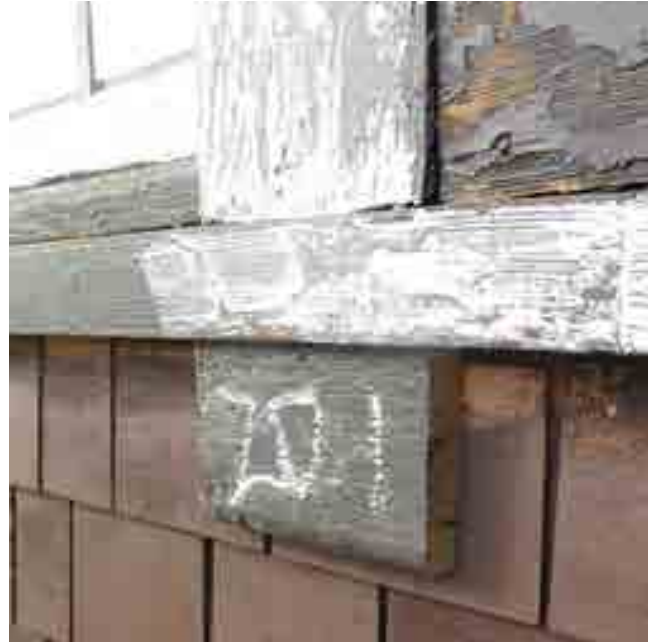
ORIGINAL BLOCKS WERE TRIMMED TO MATCH THE DIMENSIONS OF THE CASINGS ABOVE
