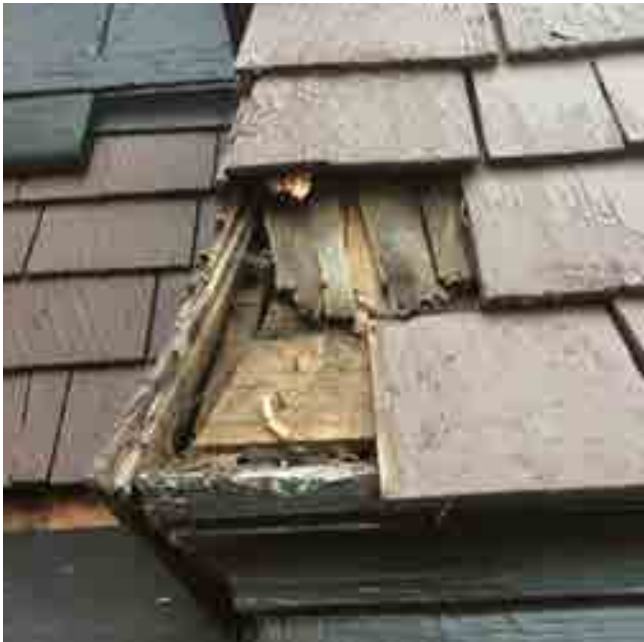
SHINGLE REMOVAL ABOVE PORCH
