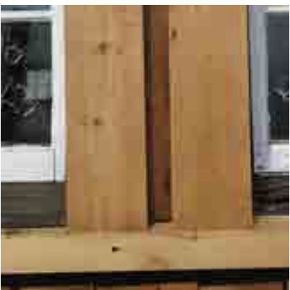
CASINGS FABRICATED AND INSTALLED ABOVE THE SILL WITH GALVANIZED FINISH NAILS
