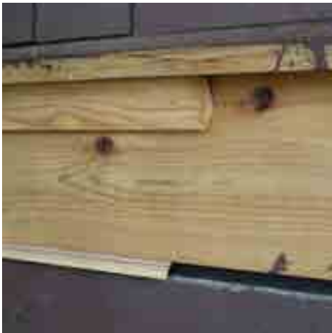
BELLY BEAM AND SILL PLATE TRIM DETAILS
