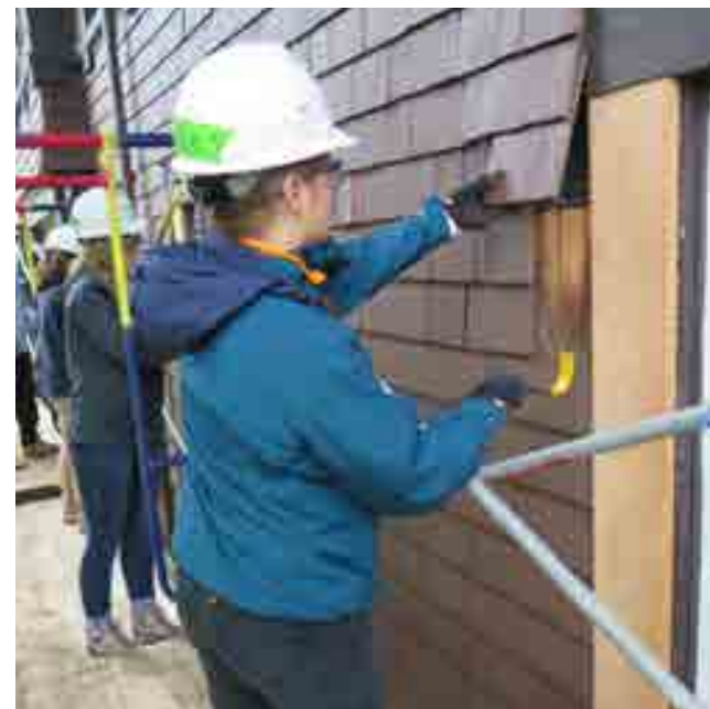
SHINGLE REMOVAL CONTINUATION
