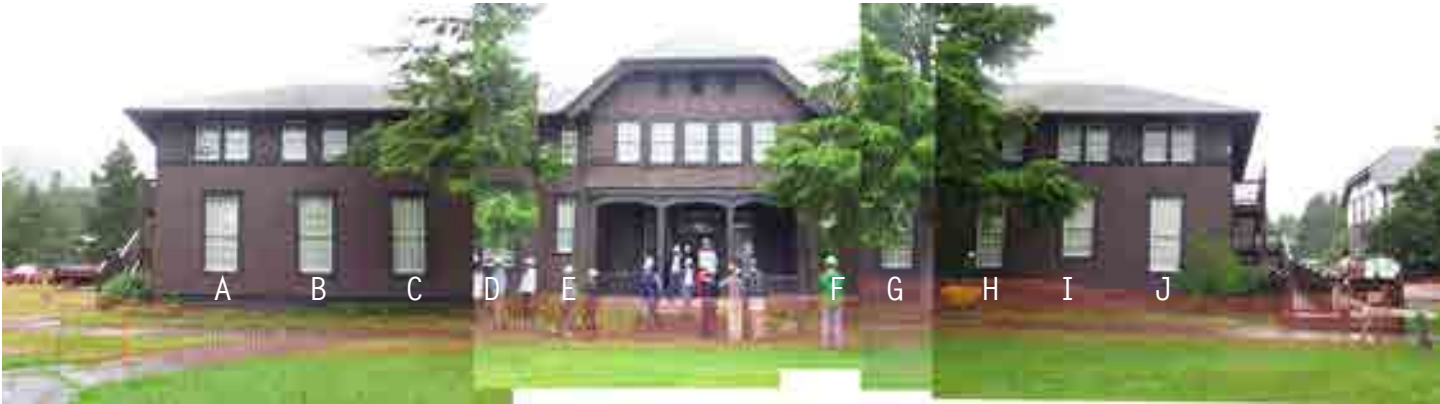
PRE FACADE REMOVAL
