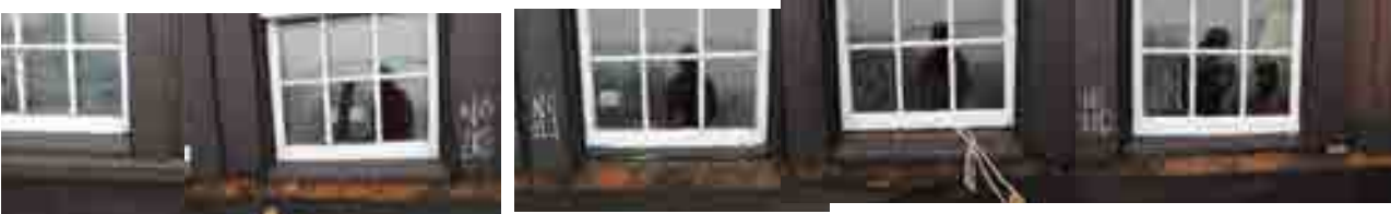
SECOND STORY WINDOWS, SHINGLES REMOVED AND TAR PAPER STAPLED ON
