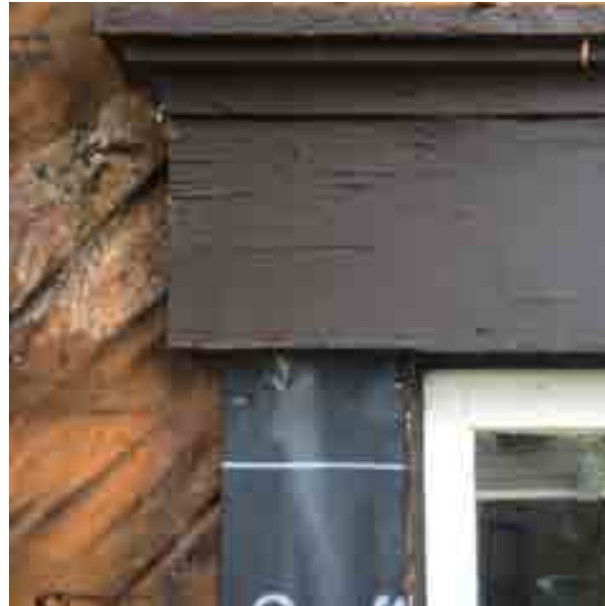
WATERPROOFING: VYCOR WATERPROOFING BENEATH CASINGS
