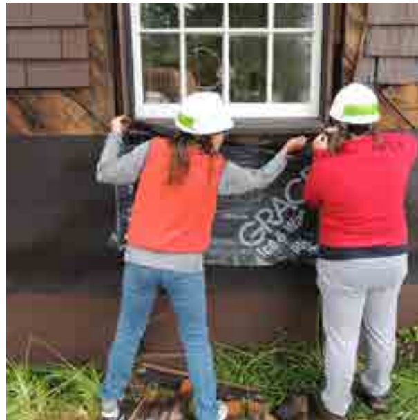
WATERPROOFING: RACHEL JONES AND ANNA PIOWAR APPLY TAR PAPER AND VYCOR TO THE PANEL AREA BENEATH THE WINDOW
