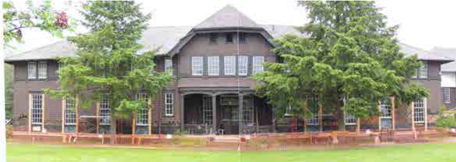
SCAFFOLDING ERECTION BEGINS
