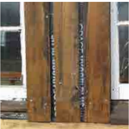
WATERPROOFING INSTALLED, 6X1S REINSTALLED WITH GALVANIZED NAILS, TURNED AROUND TO MINIMIZE DAMAGE EXPOSURE
