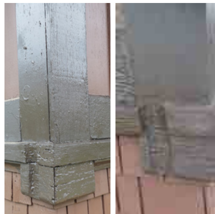
THE ORIGINAL EAST AND WEST CORNER BLOCKS HAVE CIR- CULAR CUT OUTS FOR WATER DRAINAGE PIPES WHICH NO LONGER EXIST. THE BLOCKS, HOWEVER, REMAIN.
