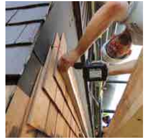
ANDY WILSON WORKS ON SHINGLE INSTALLATION NEAR THE CORNERS
