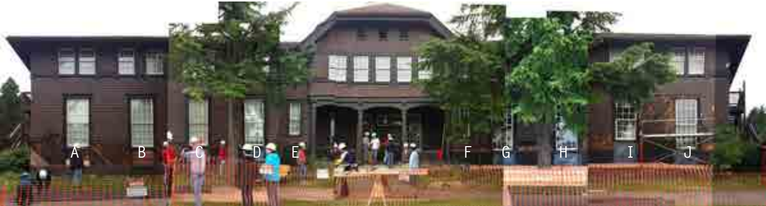
SIDING REMOVED AT FIRST LEVEL, WATERPROOFING TAR PAPER BEING STAPLED ON
