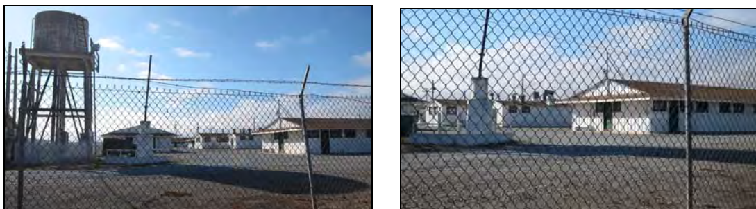
Views of Toro Labor Camp at 266 Hitchcock Road, Salinas (PAST photos).
