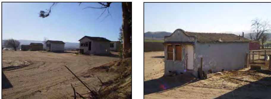
Views of labor camp housing at 56490 Cattlemen Road, San Lucas (Galvin Photos).
