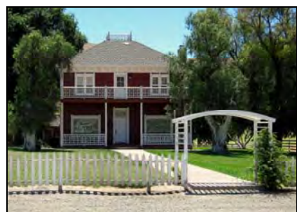
Primary residence and tank house (left) at Eade/ Cooper Ranch, 57440 Highway 198, San Lucas.
