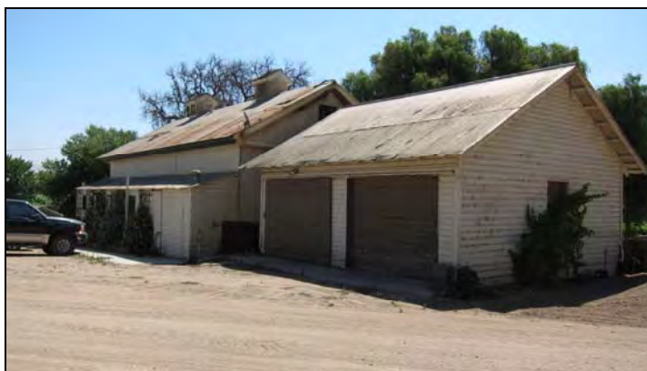
Locational cheese processing facility on River Road near the intersection of Chualar River Road (PAST photo).
