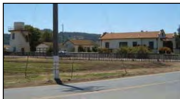
Cluster at 1660 San Juan Rd. Note early housing between the main house and tank house.
