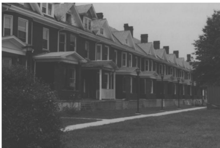
Maple Terrace Court before renovation
