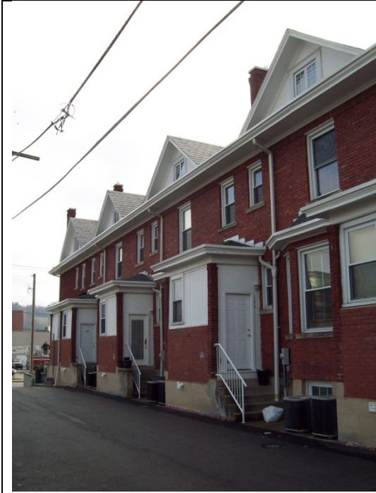
Maple Terrace Court after renovation
