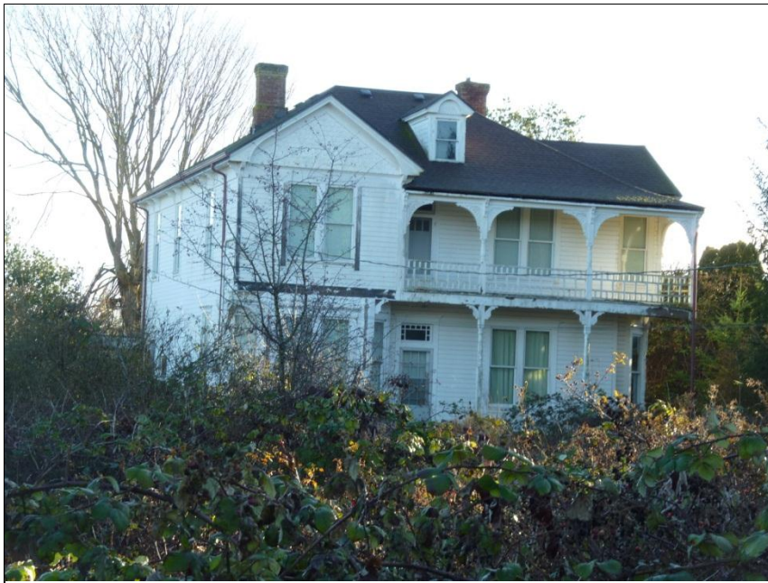
Figure 3: House at 3903 H Avenue
