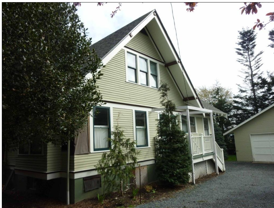
Figure 8: House at 3601 Commercial Avenue
