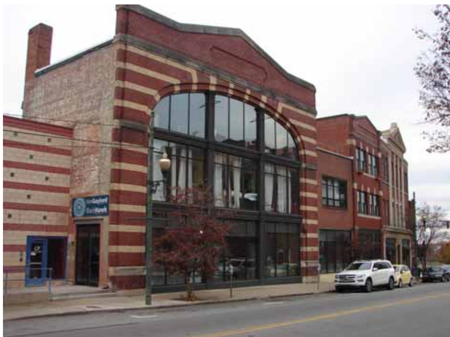
The Enterprise Machine Company Building, constructed in 1912 by J. B. Rumbough as a fireproof garage and machine shop. (Photo courtesy Heritage Strategies, LLC)
