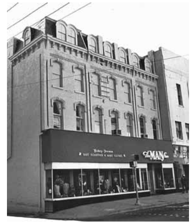
22 Patton Avenue, demolished.
