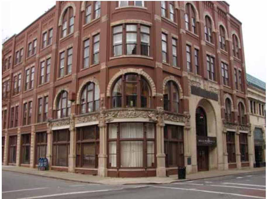
The Drhumor Building, designed by A. L. Melton in the Romanesque Revival style, was constructed in 1895 and is one of the oldest commercial buildings in downtown Asheville. (Photo courtesy Heritage Strategies, LLC)
