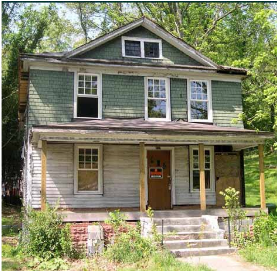
Photos, facing pages: Flint Street home in Montford, before and after rehabilitation. (Photos courtesy North Carolina State Historic Preservation Office)
