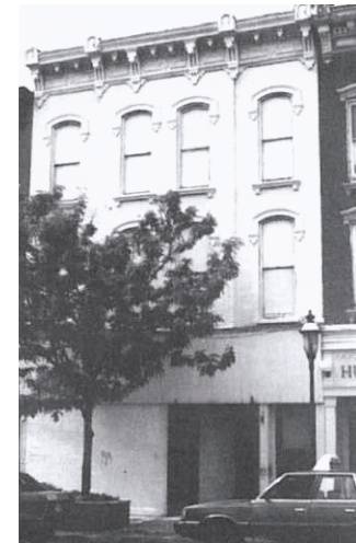
No: Windows boarded
