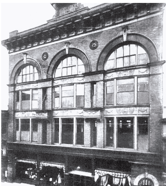
The Rosenbaum building, located at 118 Baltimore Street, was built in 1899
