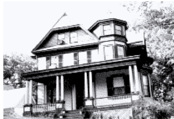
Typical example of historic porch
