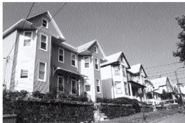
Typical example of a stone retaining wall
