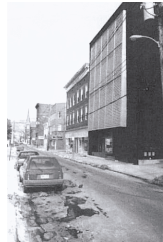
No: Exterior screen over windows
