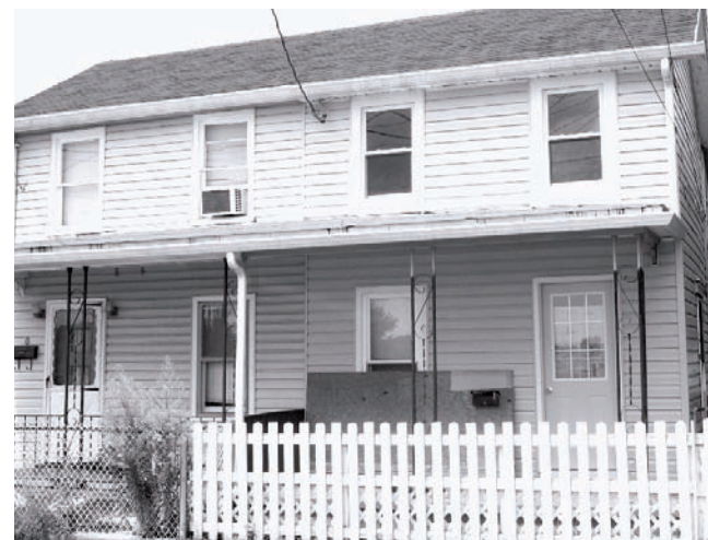
No flat iron replacement posts
