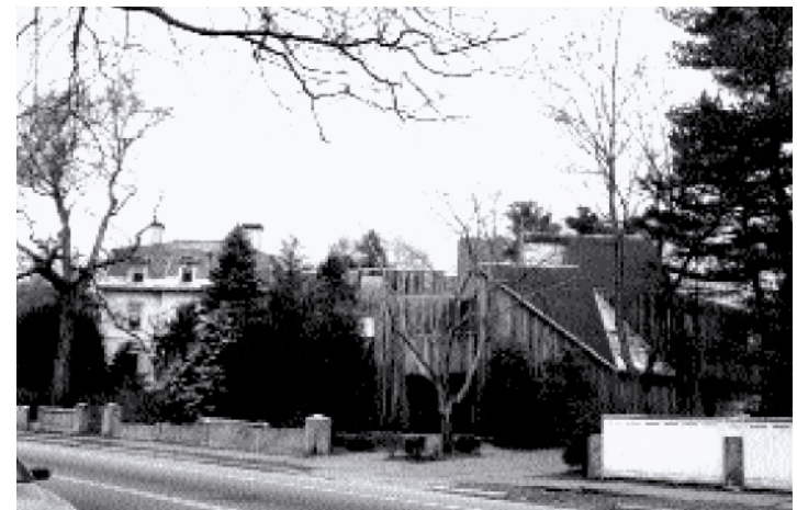
No: Modern roof inappropriate to neighborhood
