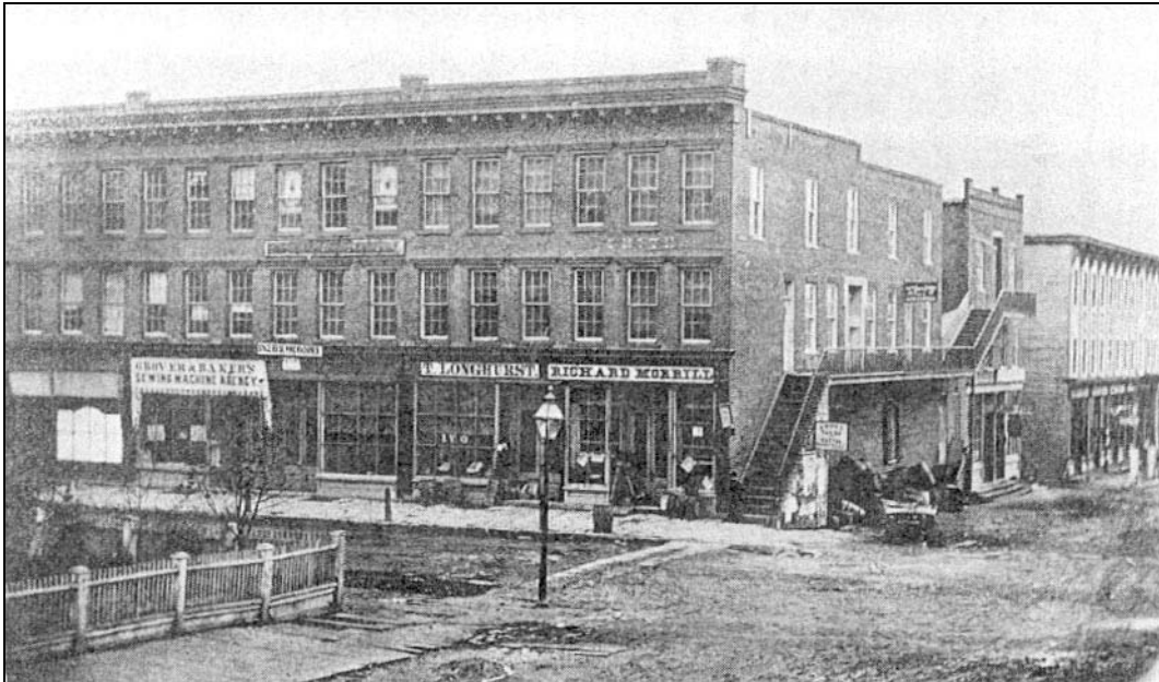
Figure 41: Sanford Block, northeast corner 8 th and Main, view northeast, c.1857 (Wilkie, p. 161)
