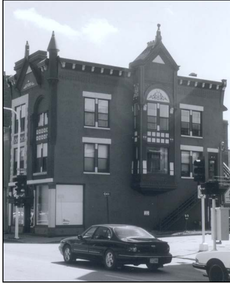
Figure 65: 1497 Central, c.late 1890s, (photo by Jacobsen, 2002) (Two-part commercial block type)
