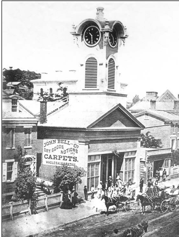
Figure 35: First Clock Tower Building, a former Congregational church (built 1845, collapsed 1872), west side Main north of 8 th , c.1872. This was a temple front converted for store use and any Italianate style linkage is derived from the addition of the clock tower.
