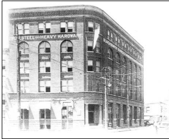
Figure 92: John Ernsdorff Iron Company five-story block, 250 Jones, c.1890s, photo c.1905 (Center For Dubuque History, Loras College, Photograph, Hoffman #01016)
