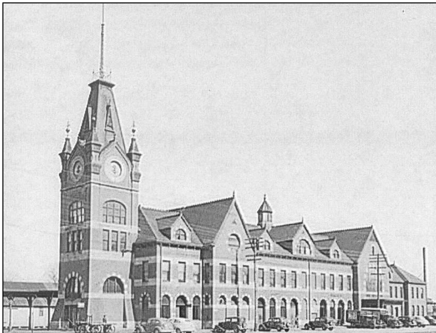
Figure72: Illinois Central Railroad Passenger Depot (John Vachon photo, c.1940, American Memory, Library of Congress) (Two-part commercial block type)
