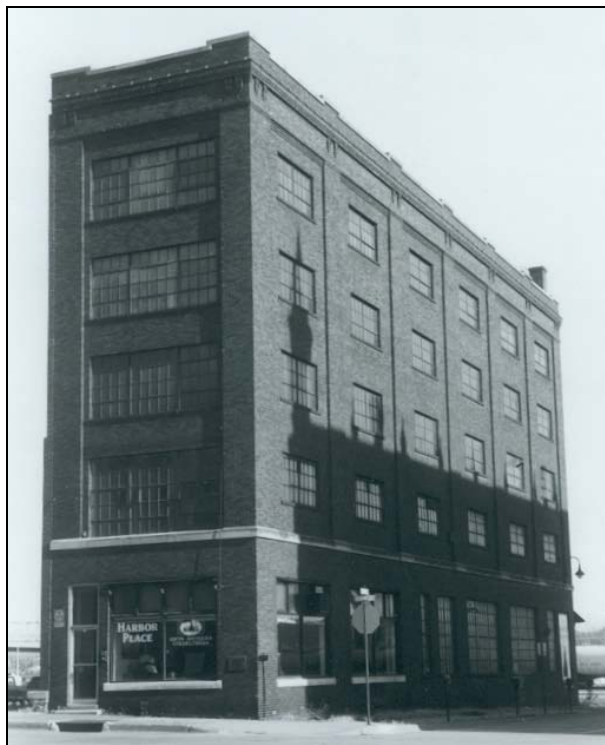
Figure 86: 104 Main, Harbor Place, 1926 (photo by Jacobsen, 2002) (Two-part Commercial Block type)
