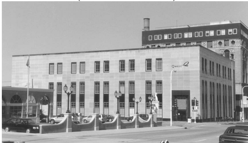
Figure 88: US West Building, Locust and 9 th streets (photo by Jacobsen, 2002) (Vault Block Type)
