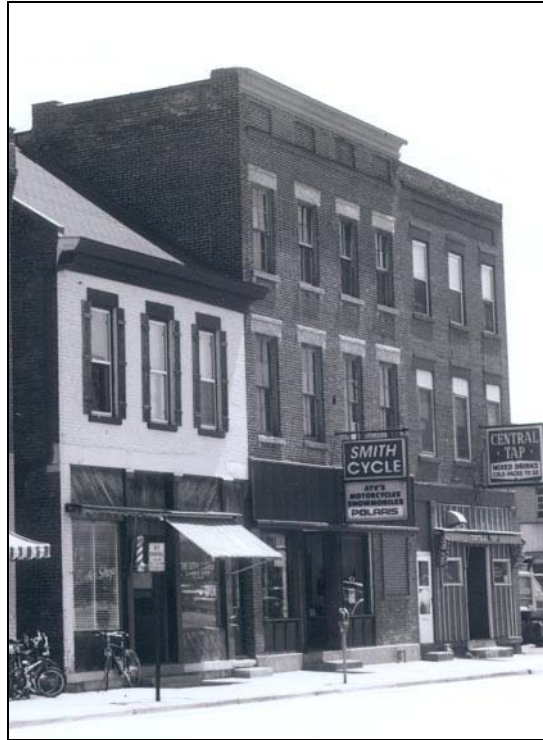
Figure 44: 1056 Central Avenue (center, view southeast) (Photo by J. Jacobsen, May 2003)
