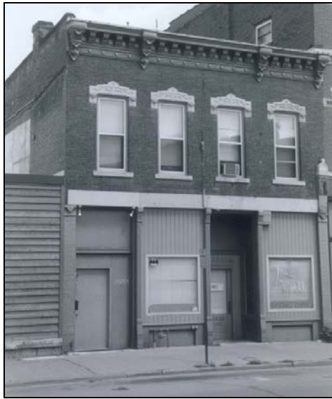
Figure 51: 1626 Central Avenue, 1880 (photo by Jacobsen, 2002) Later example of the solid stone lintel element.
