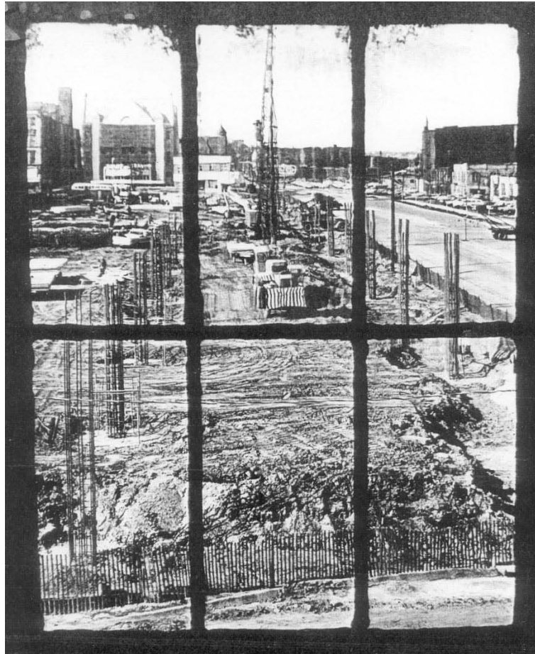
Figure 17: Urban renewal demolition along Iowa Avenue, parking ramp construction, viewed north from 5 th Street (Center for Dubuque History, Loras College, Photographs, Urban Renewal) Note the Grand Theater at upper left.
