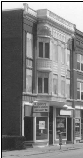
Figure 63: Fred A. Nesler Block, 1732-36 Central Avenue, 1892, view southeast (photo by J. Jacobsen, November 2002)
