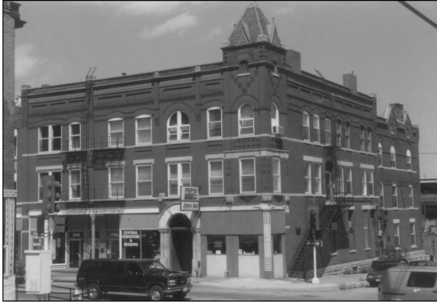
Figure 62: Rider & Lacy Block, 1702-22 Central Avenue, 1891, view northeast (photo by J. Jacobsen, November 2002)
