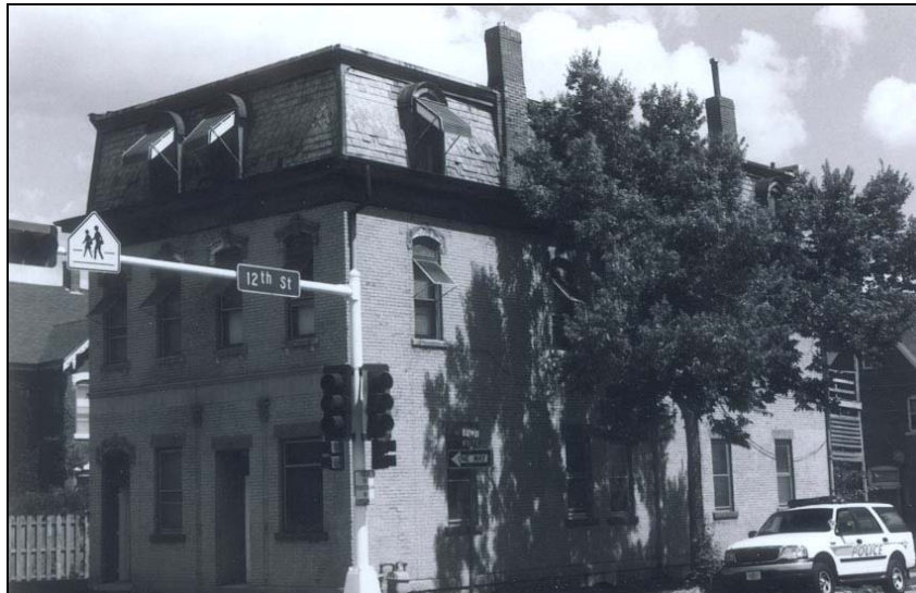
Figure 59: 1200-02 White Street, c.1879-80 (photo by Jim Jacobsen, November 2002)
