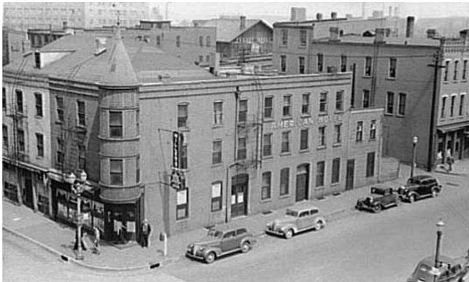
Figure 61: American Hotel, northeast corner Clay and 4 th , non-extant, view northeast (John Vachon photo. 1940)
