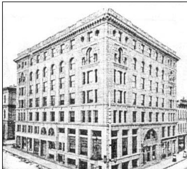
Figure 78: Bank and Insurance Building, 9 th and Main, 1894, original photo (photo, Sommer, p. 127) (Stacked Vertical Block type)
