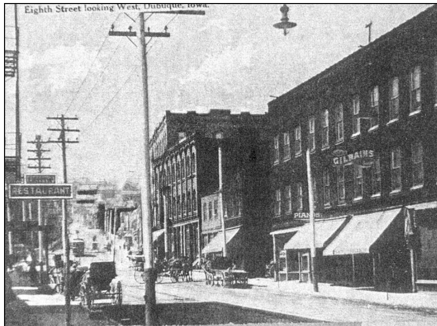
Figure 9: West Eighth/Julien Avenue, viewed west from Locust Street, c.1905 (Center For Dubuque History, Loras College, Photo FBL #3805) Lorimer House is the tall building in the distant center.
