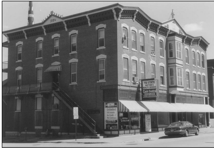
Figure 56: J. Simones Block, 1570-98 Central Avenue, 1884, view southeast (photo by J. Jacobsen, November 2002)
