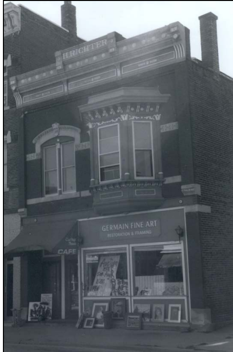
Figure 64: H. Richter Block, 1543 Central Avenue, c.1894, view southwest view southwest (photo by J. Jacobsen, November 2002)
