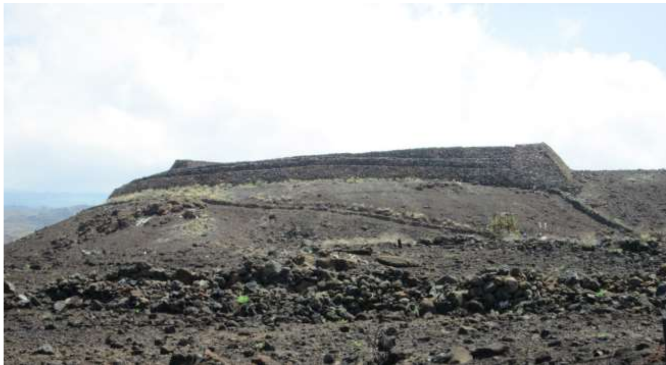
Pu’ukohola Heiau following the Kawaihae Fire.
