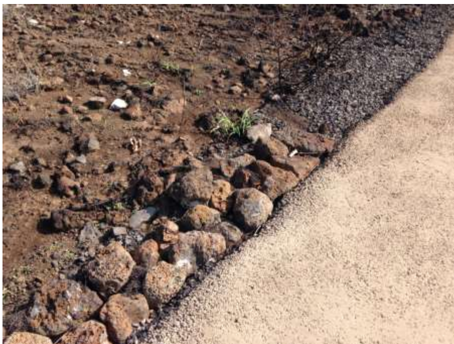
Example of an appropriate trail edge treatment below; blue gravel above.
