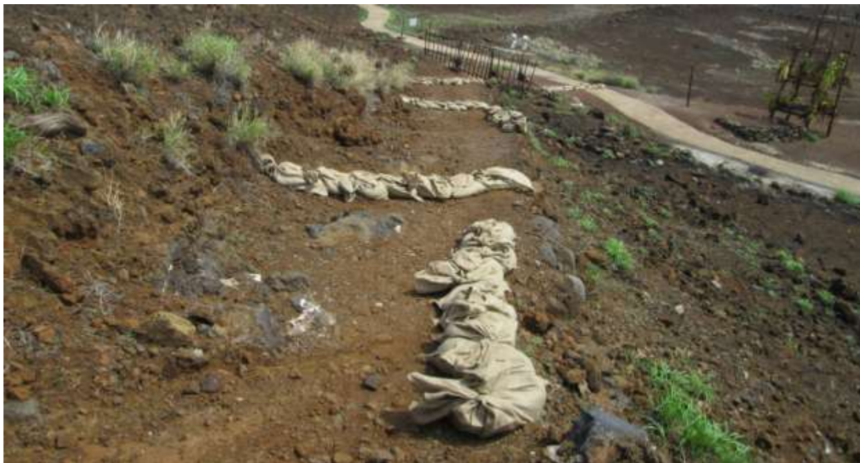
Sandbag treatment along the Pu'ukohola Heiau access trail.
