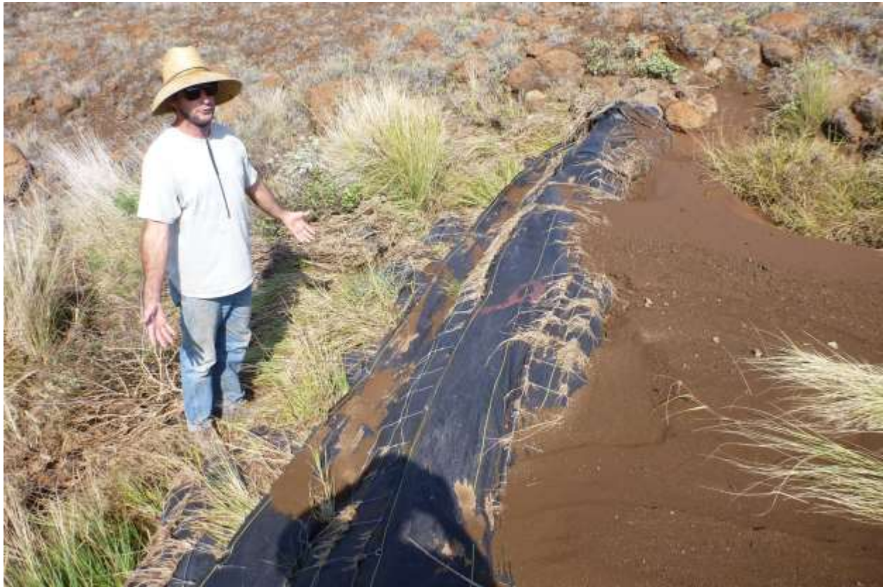
Figure W-5. Example of filled sediment dam on private lands.
