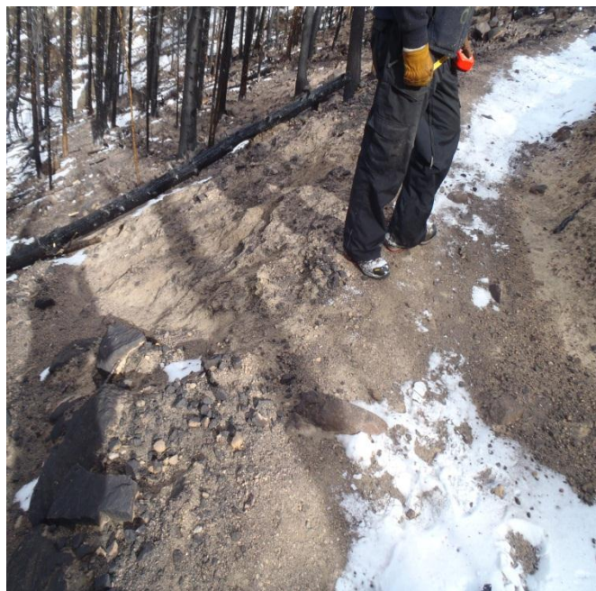
Photo 4 - Eroding trail edge
