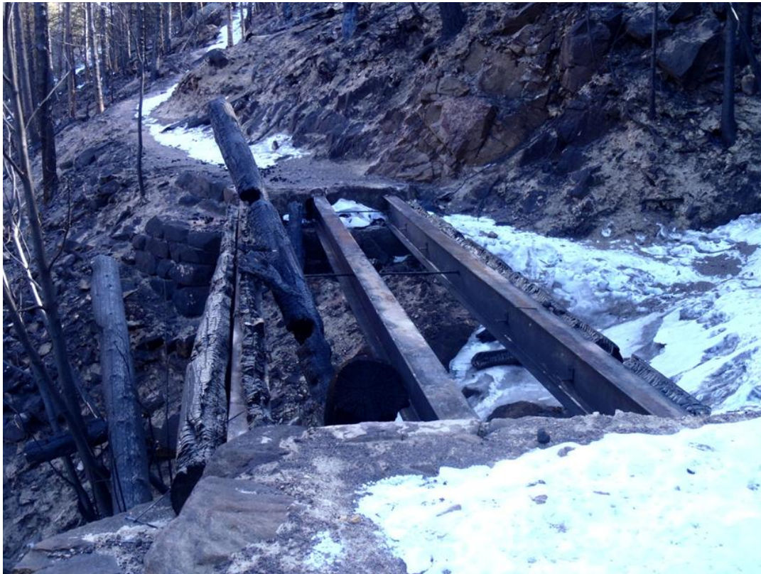
Photo 9 - B1-24-5 Wuh Creek Bridge After
