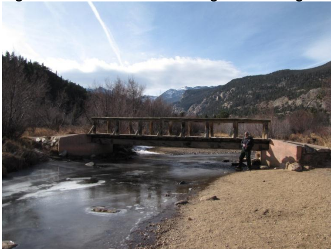
Figure 7: Cub Creek Trail Bridge across Big Thompson River below Burned Area
