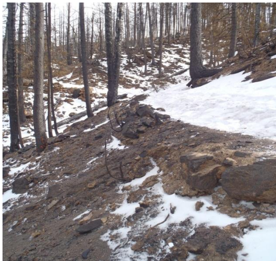
Photo 1 - Damaged Rock Walls
