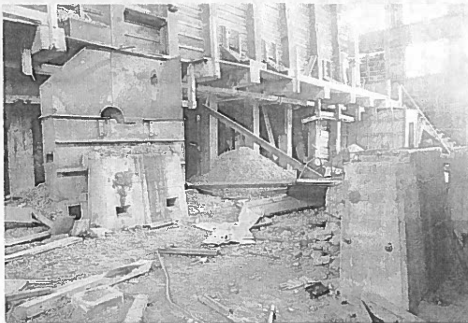
Figure 34: Looking southeast at the stamp and ball mill area in this 1982 photograph. Note the ore bins and the concrete foundation piers for the machinery.
