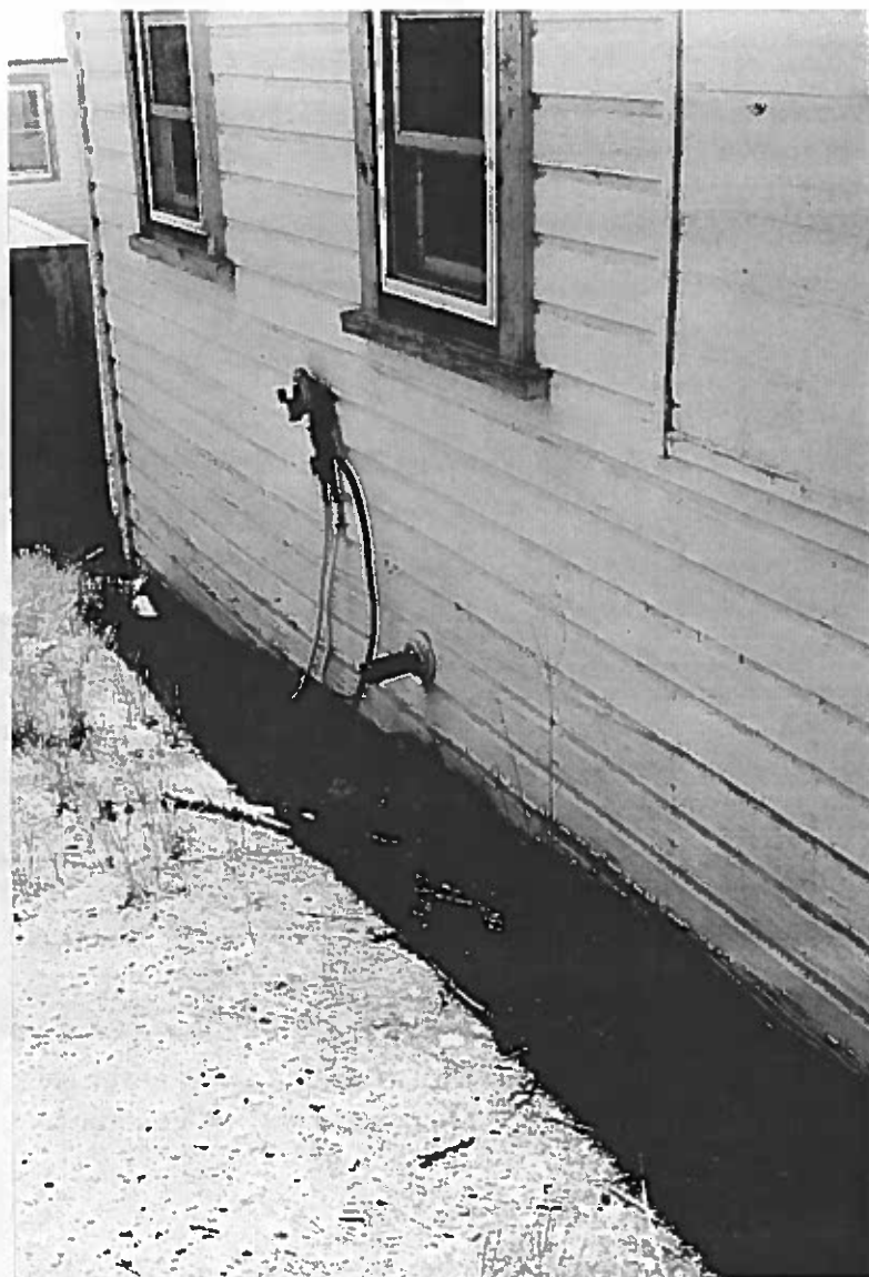
Figure 78: Looking southwest at the back of the building. Note the high grade around the bottom siding and sill plate.
