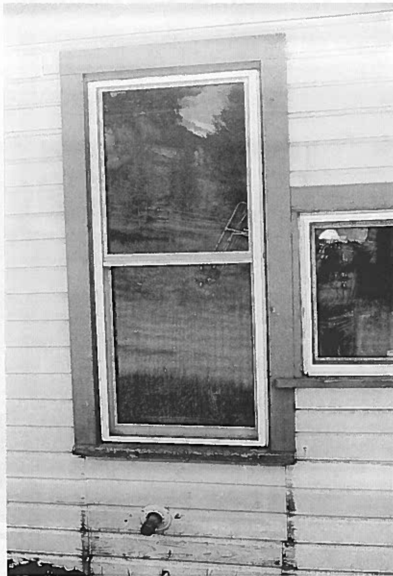
Figure 75: Looking at the vinyl windows covered windows that have replaced the original wood double-hung windows. They are in good condition.
