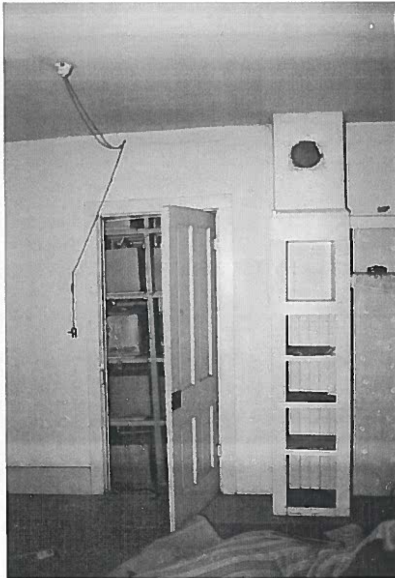
Figure 205: Looking east at the middle bedroom. The materials on the walls, ceiling, and floors are similar and in good condition.
