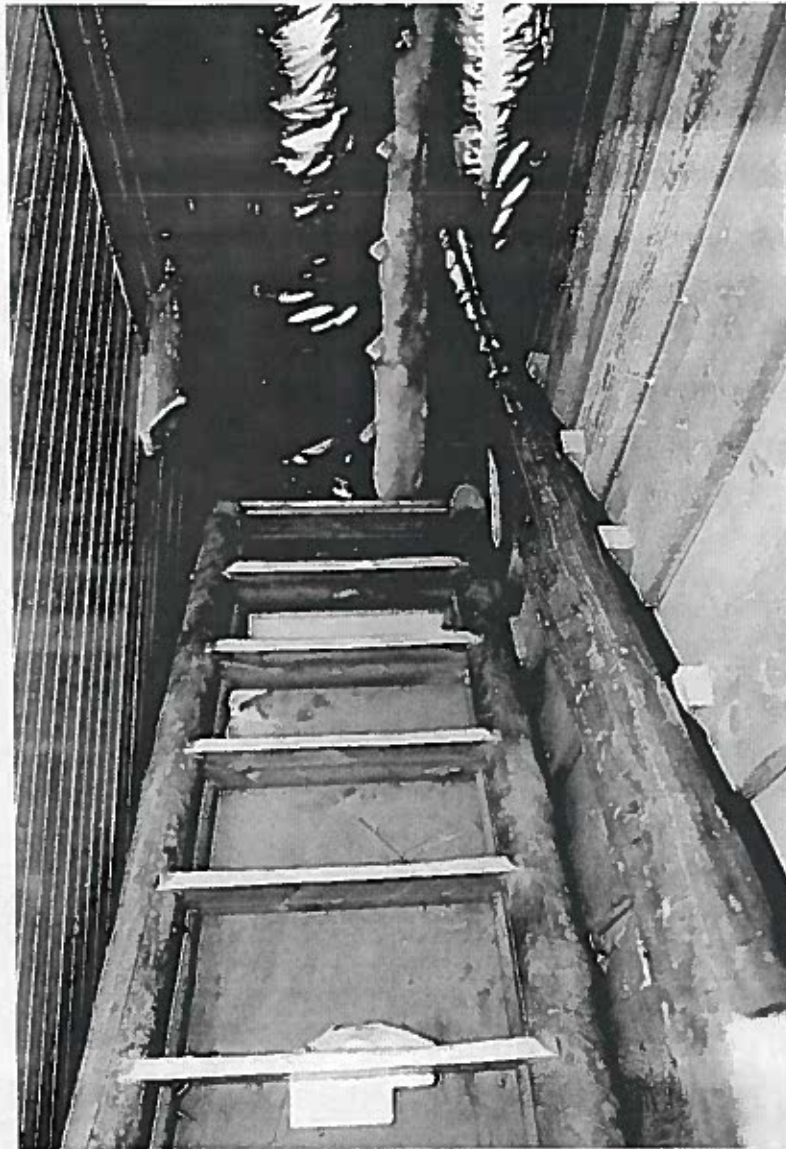
Figure 145: Looking up the stair steps to the attic space. The steps are very steep.
