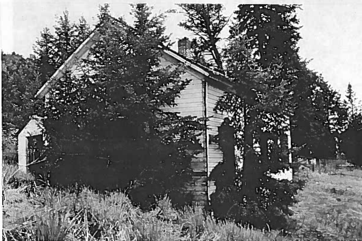
Figure 105: Looking southeast at the building. Note the trees that have grown up around the building which cause deterioration to the foundation and wall materials.
