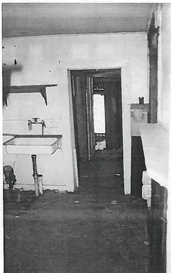
Figure 174: Looking north at the back door from the kitchen in to the back frame addition.
