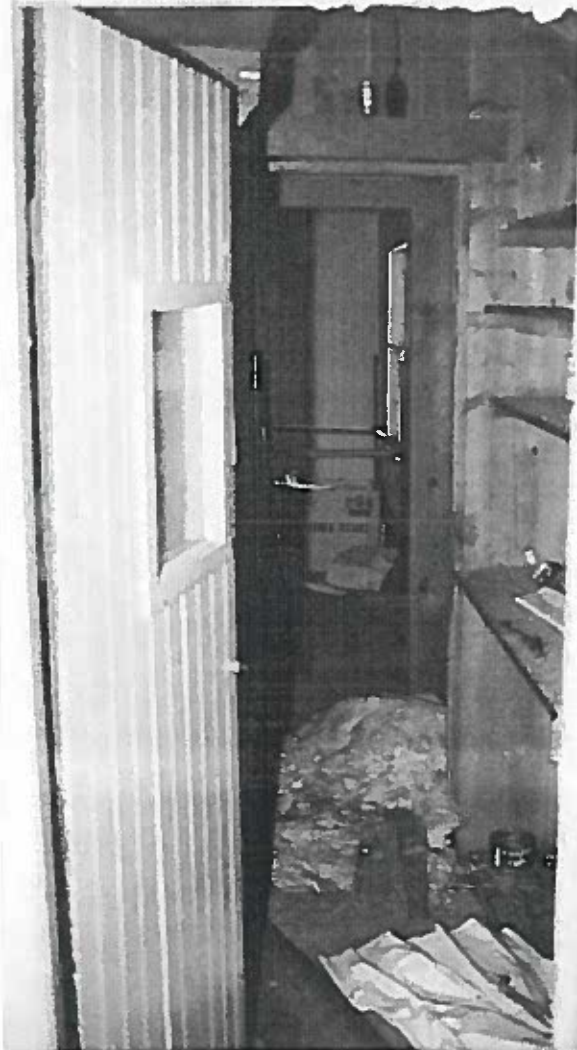
Figure 206: Looking east at the corridor between the back bedroom and the front vestibule. This appears to have been a storage area with its natural wood.
