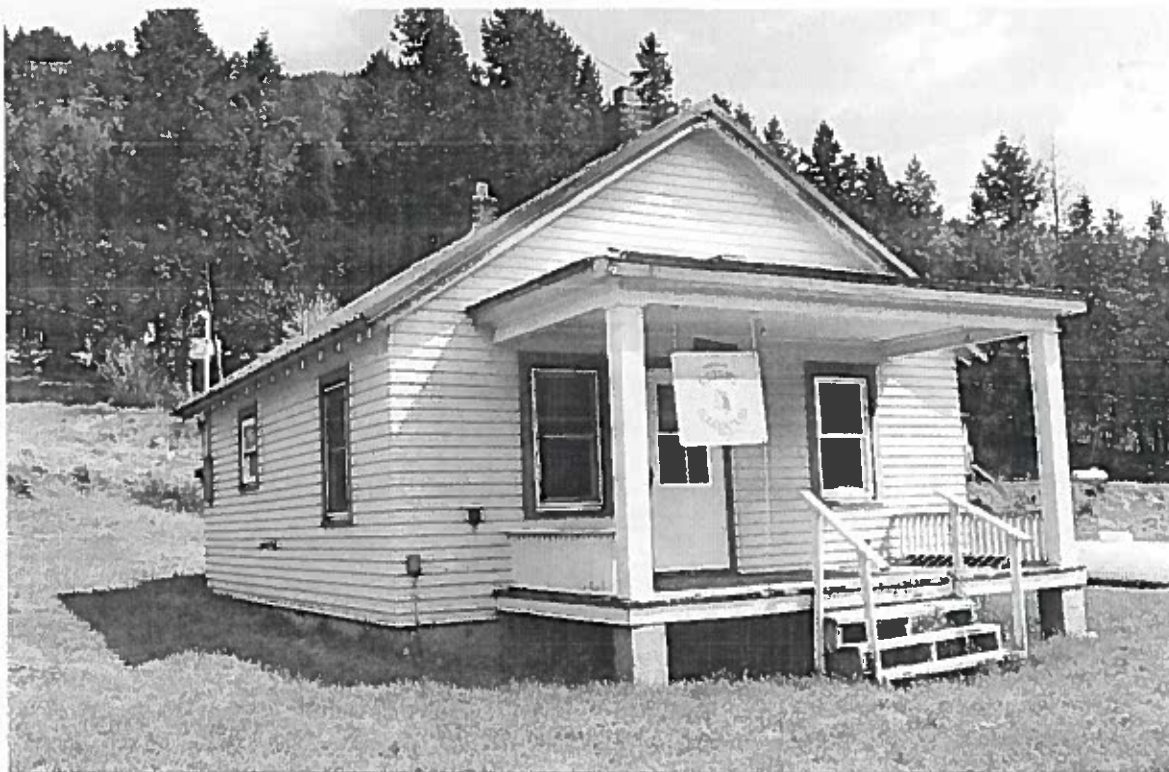
Figure 235: Looking southeast at the residence. The exterior concrete foundation, wood siding, and metal roof are in good condition.
