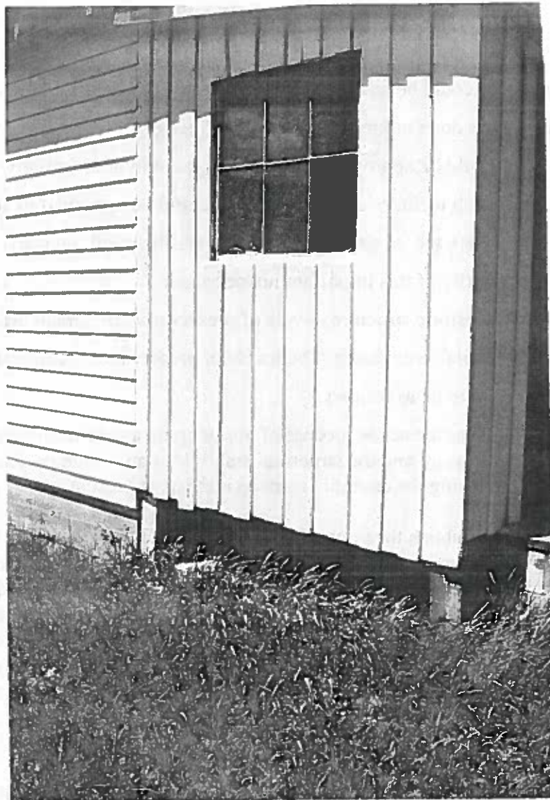
Figure 258: Looking northwest at the addition. The building sits on some wood blocking..
