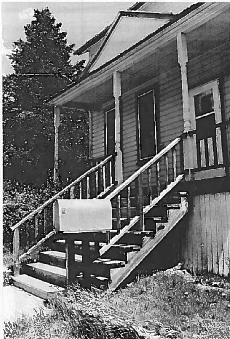
Figure 85: Looking northeast at the front steps. These steps have been rebuilt for the building.
