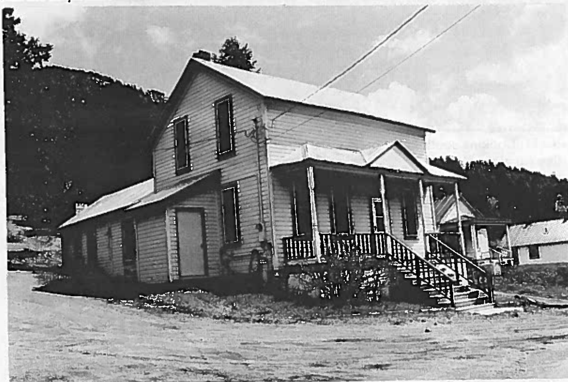
Figure 70: Looking southeast at the building. Note the shed roof addition to the building. The galvanized metal roof on the building covers the original wood shingles. The metal is in good condition.
