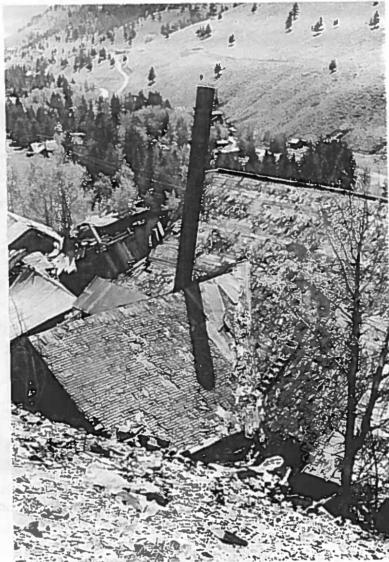
Figure 22: Looking southwest at the roof of the Mill and at the stack of the upper boiler area.
