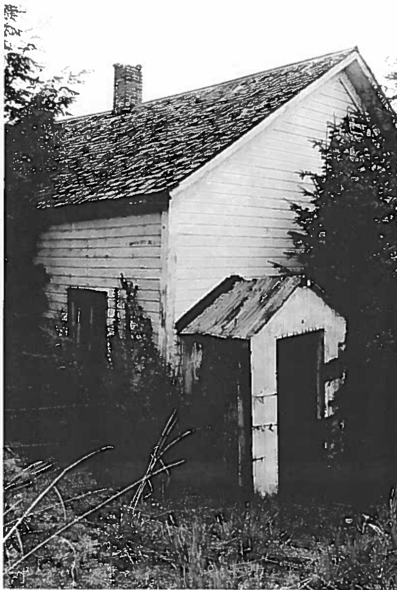
Figure 107: Looking west at the building. Note the wood shingle roof that is in fair condition. Also, note the deteriorating brick chimney on the top of the roof.
