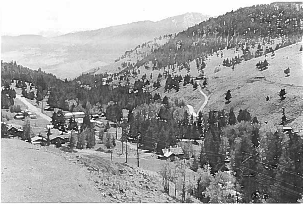
Figure 2: Looking southwest at the town of Jardine from the new mill site above the Revenue Mill.
