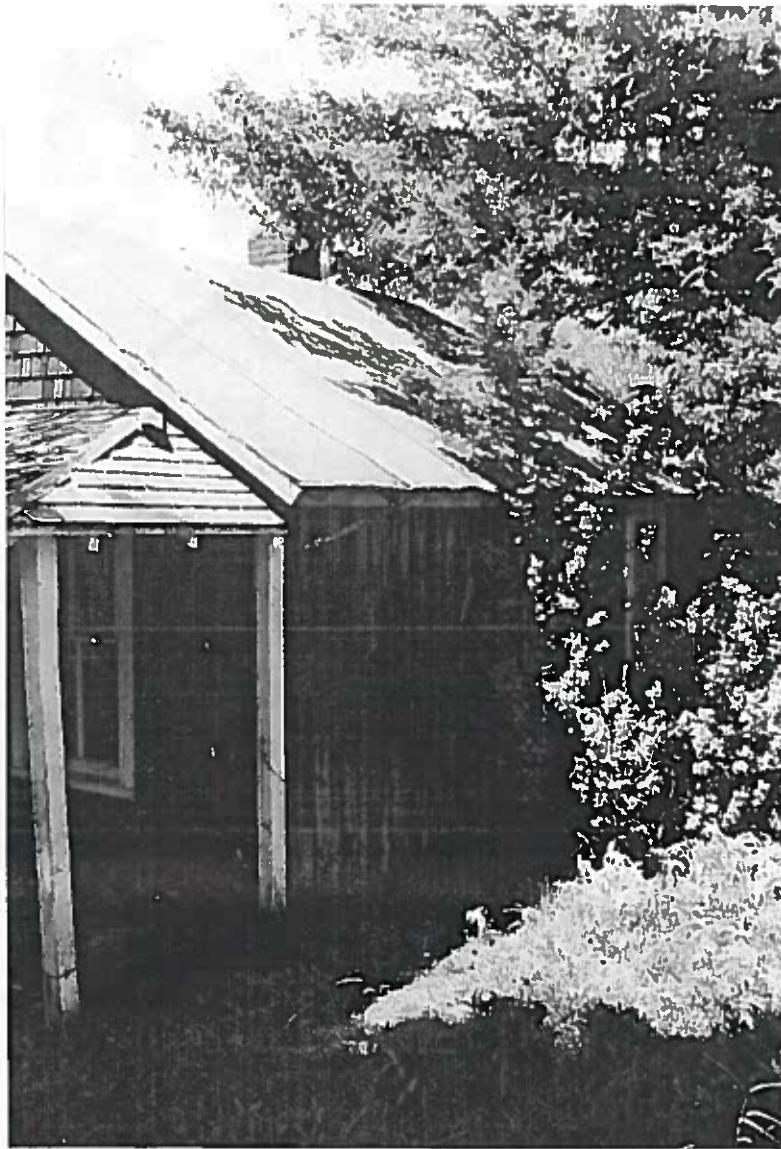
Figure 190: Looking southwest at the Cabin. The metal roof on this side of the building is in good condition. Note the brush and trees up against the building.
