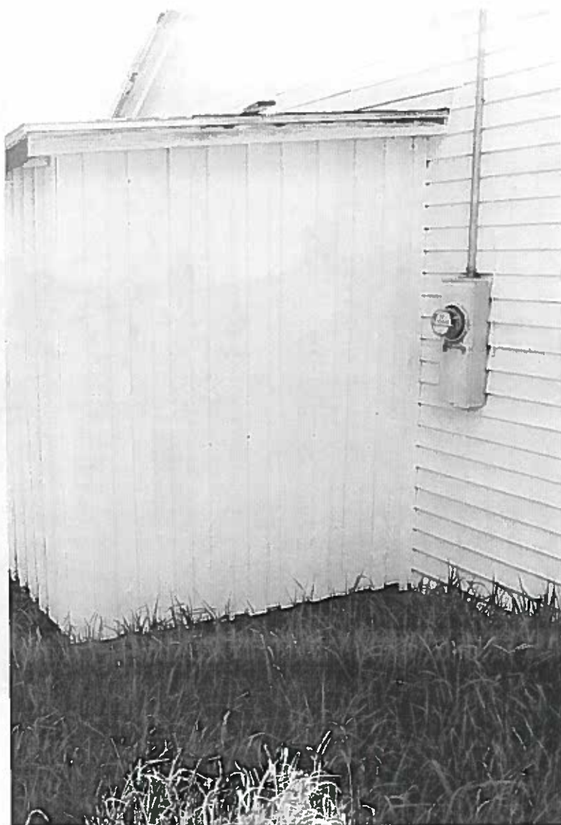
Figure 257: Looking southwest at the addition which is a frame structure with board and batten siding. It is in good condition but has no foundation under it.
