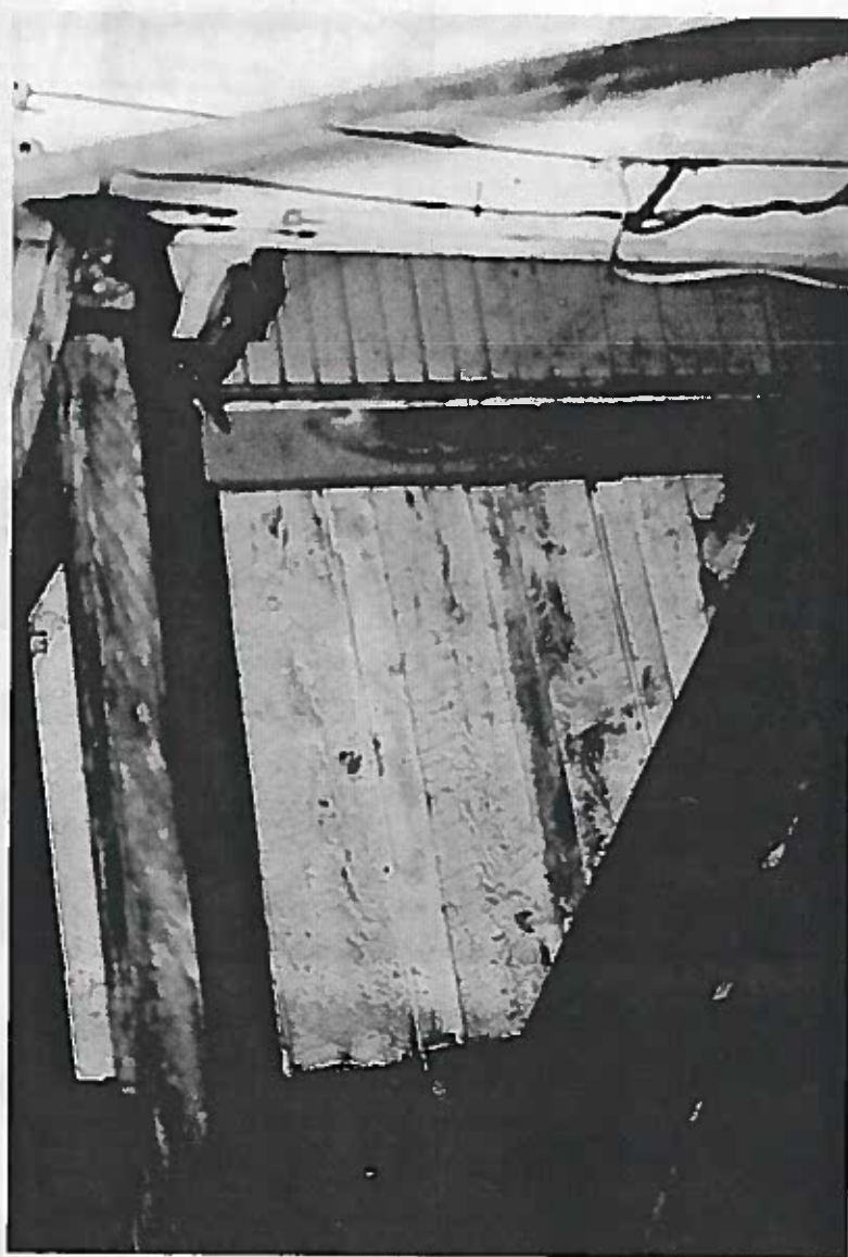
Figure 136: Looking east at the steep steps up to the first floor.
