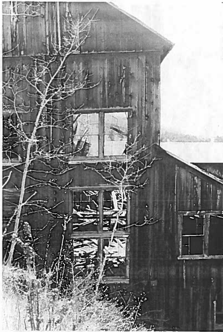
Figure 17: Looking south at the north wall of the Mill at the stamp mill and ball mill level.
