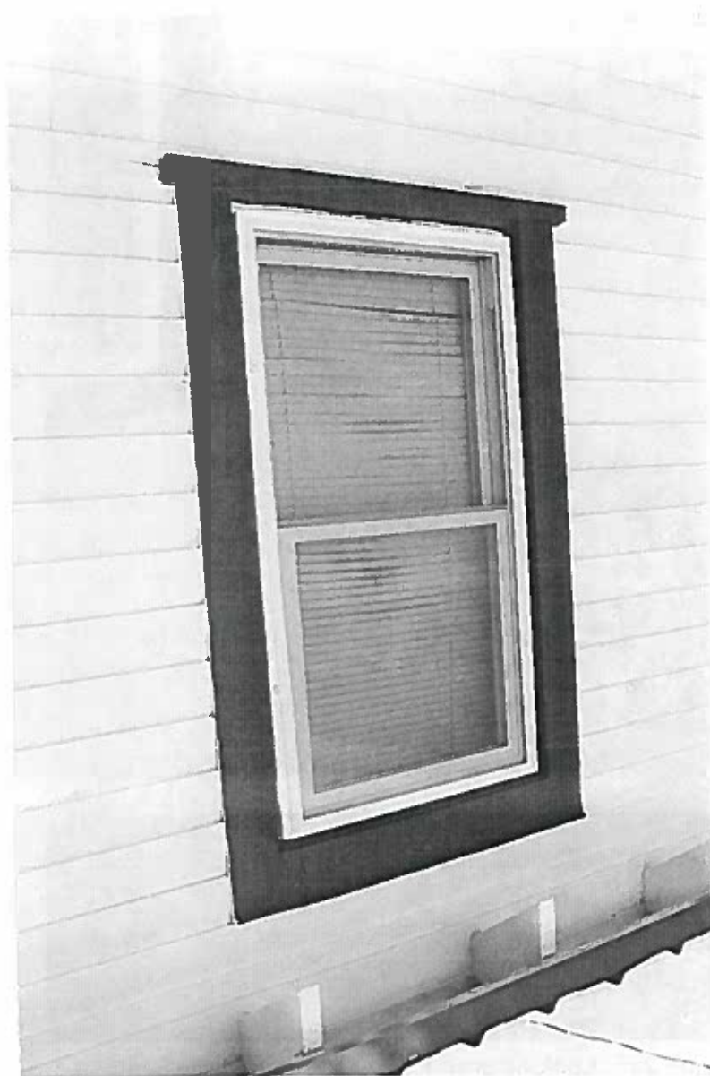
Figure 254: Looking southeast at a typical wood double-hung window. The window and adjacent materials are in good condition.
