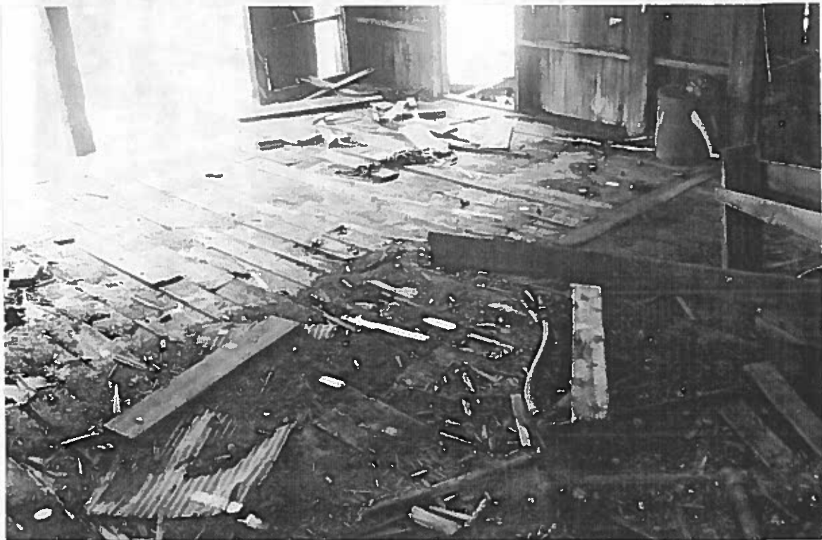
Figure 28: Looking north at the floor on the north end of the lower level.
