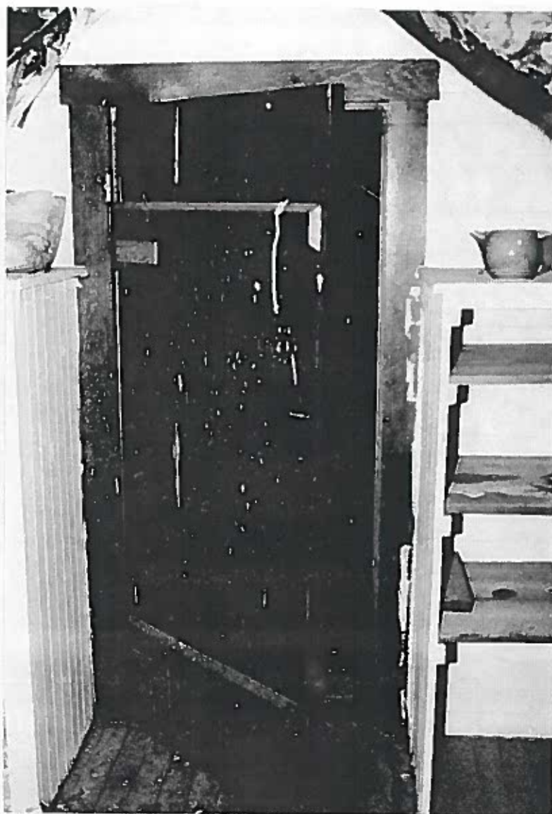
Figure 149: Looking west at the wood door leading out of the finished half of the attic.
