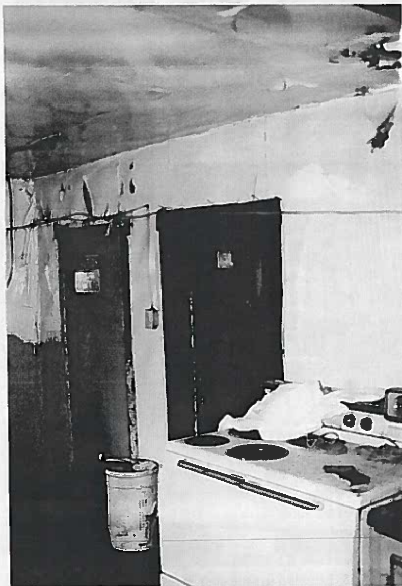
Figure 144: Looking northeast at the door to bathroom. The wall and ceiling papers have been painted.
