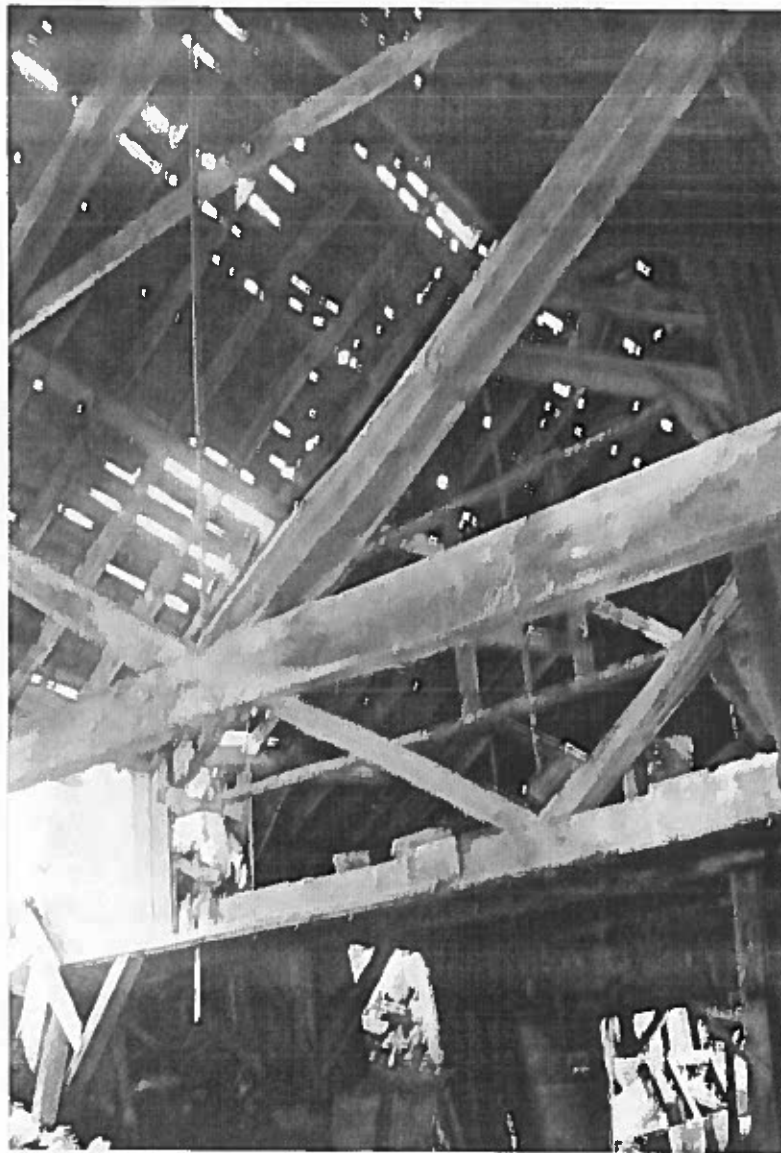
Figure 37: Looking south at the roof truss structure in the upper end of the Mill. The trusses even though not supported very well on the east end of the building, appear to be in good condition.
