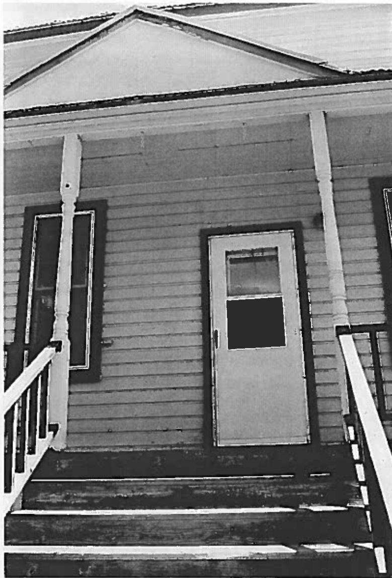
Figure 86: Looking east at the entrance door. There is a metal storm door.
