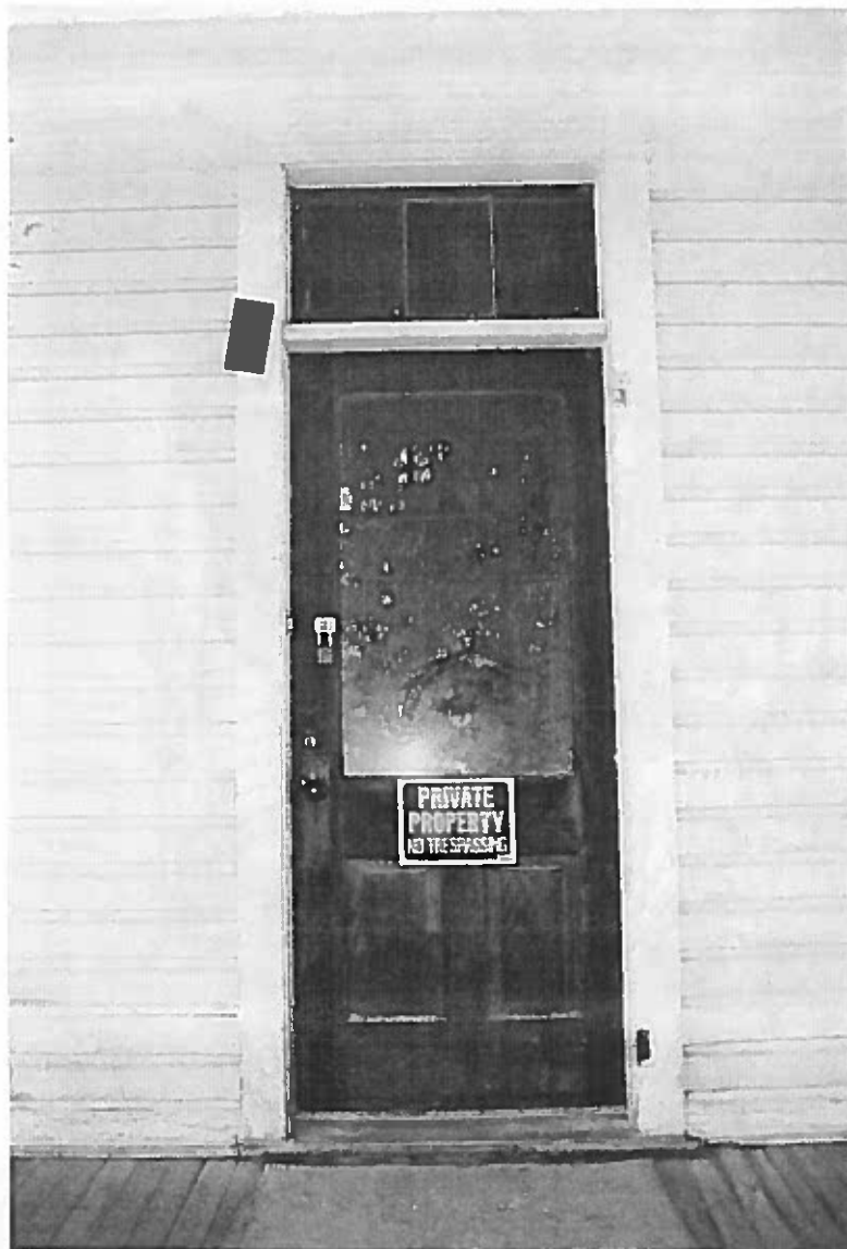
Figure 43: Looking north at the entrance door to the building. The door is worn and there is some minor deterioration at the base of the door and trim, due to moisture. Other than that the materials are in good condition.
