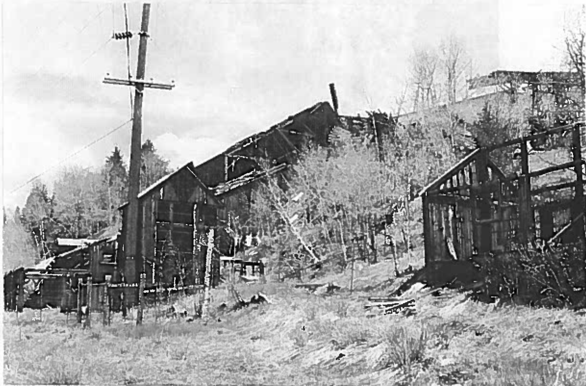
Figure 7: Looking northeast at the Revenue Mill. Note the fenced area around the mill to keep people out of the dangerous areas.
