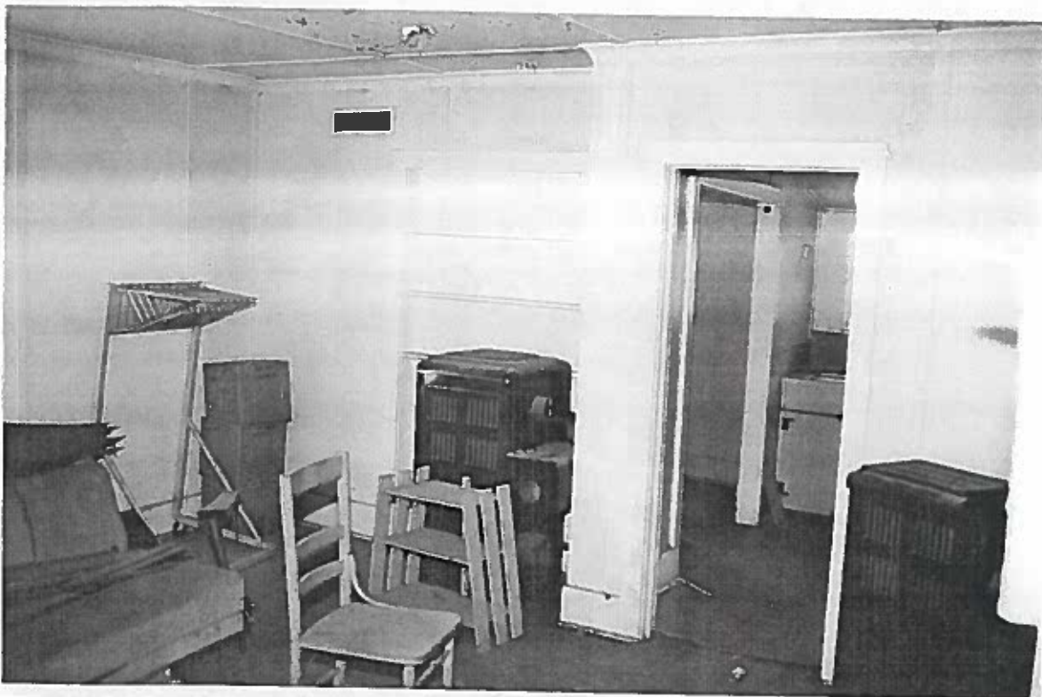
Figure 196: Looking southwest at the front room. The plaster walls and ceiling, wood floors and general woodwork appears to be in good condition.
