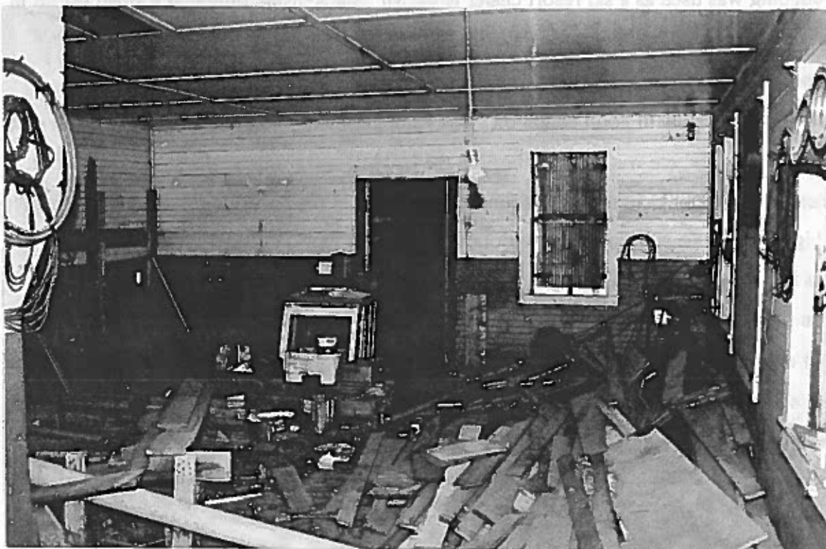
Figure 114: Looking south at the entrance to the room. Note the window sash on the floor. Most of the interior materials are in good condition with some minor wear.
