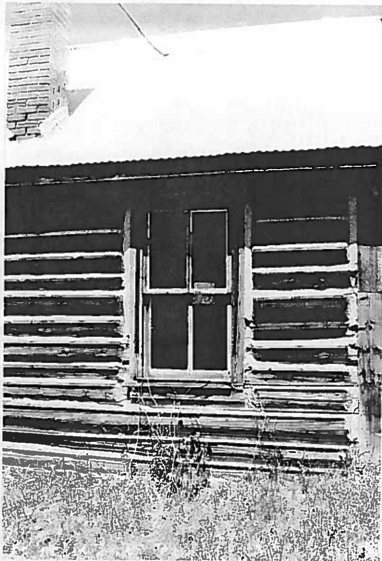
Figure 120: Looking north at the log work and a typical wood double-hung window on the house. The logs and wood windows are weathered but are in good condition. There is some missing putty in the windows and some rot along the base of the logs.
