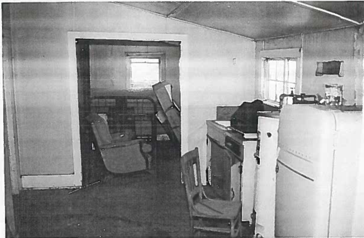
Figure 201: Looking south at the kitchen and dining room area on the back of the building. The materials are generally in good condition in these areas.
