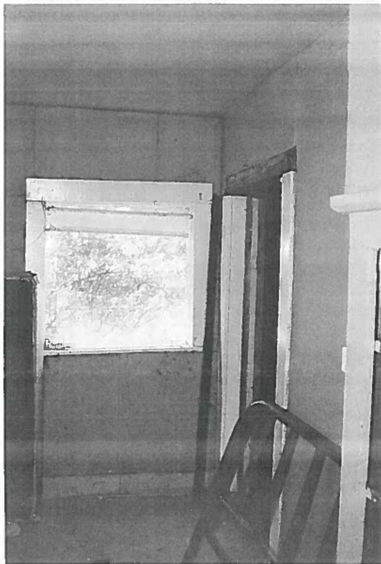
Figure 230: Looking south at the door to the living room and a single pane window that has been added to the opening.
