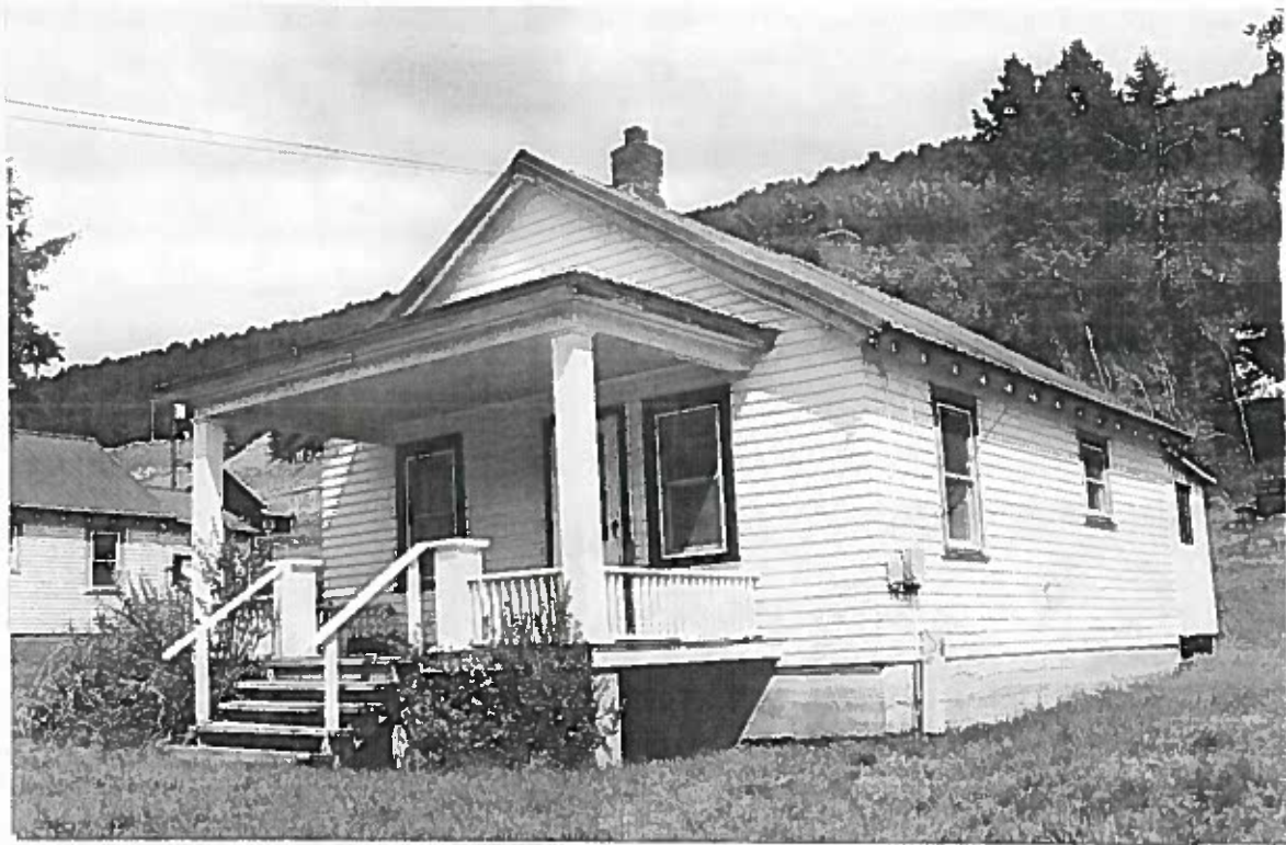
Figure 251: Looking northeast at the Residence. The foundation, walls and roof are in good condition.
