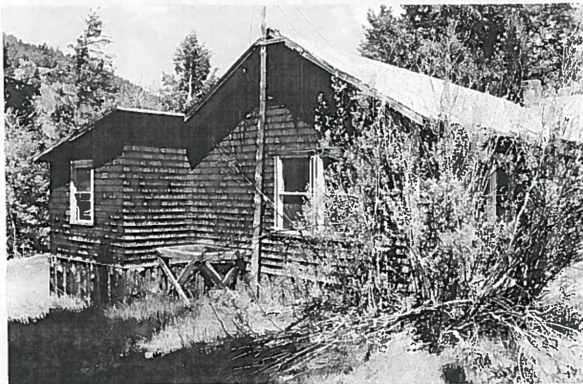
Figure 182: Looking northwest at the end of the building. Note the weathered shingles.
