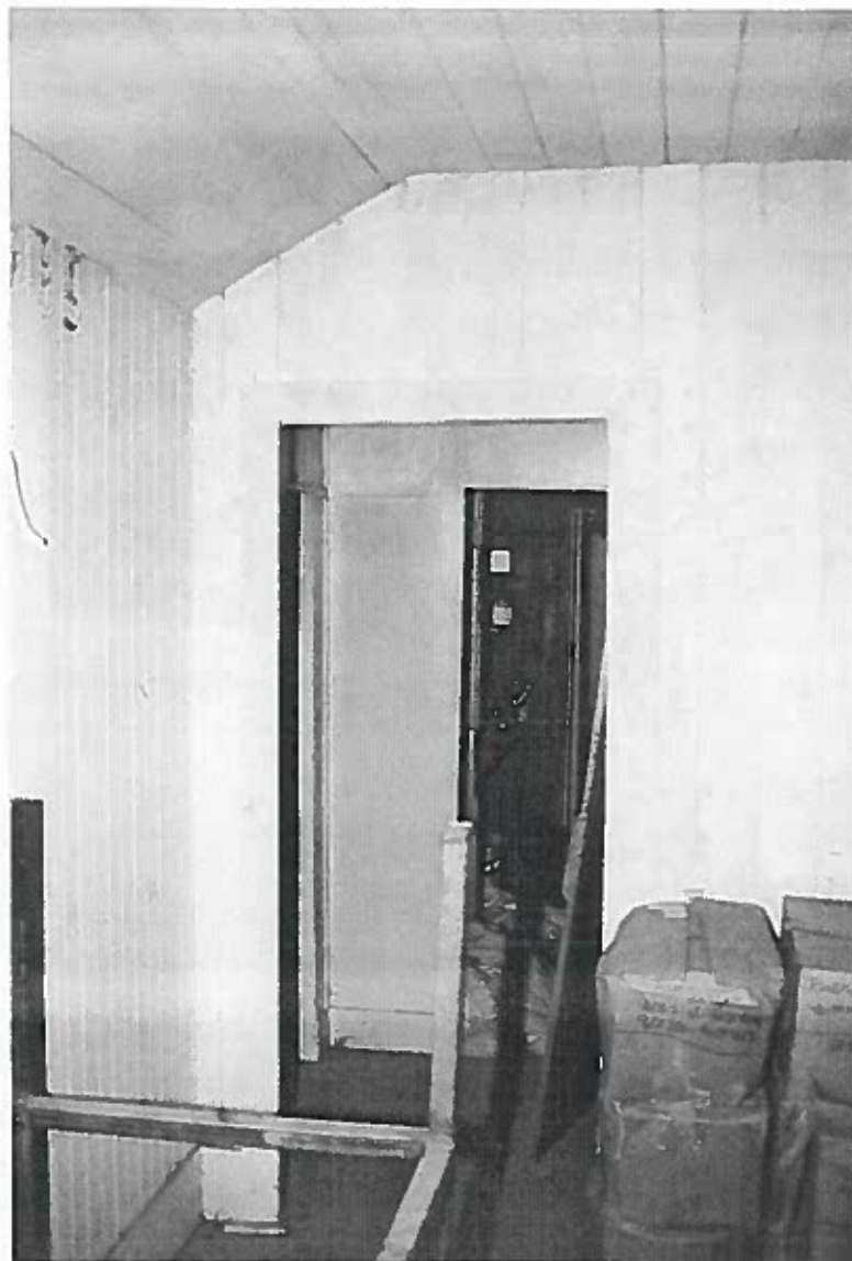
Figure 208: Looking west at the front bedroom towards the door to the front vestibule area.
