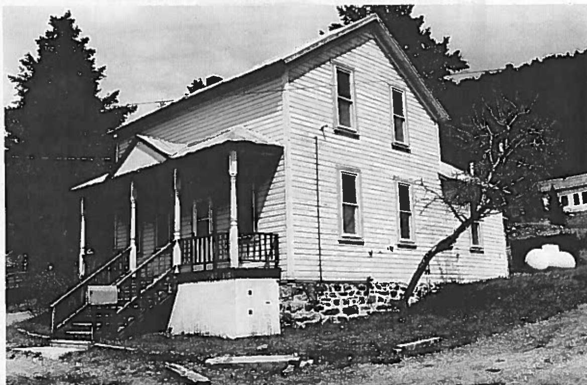
Figure 83: Looking northeast at the building. The wood siding is in good condition with some minor wear.
