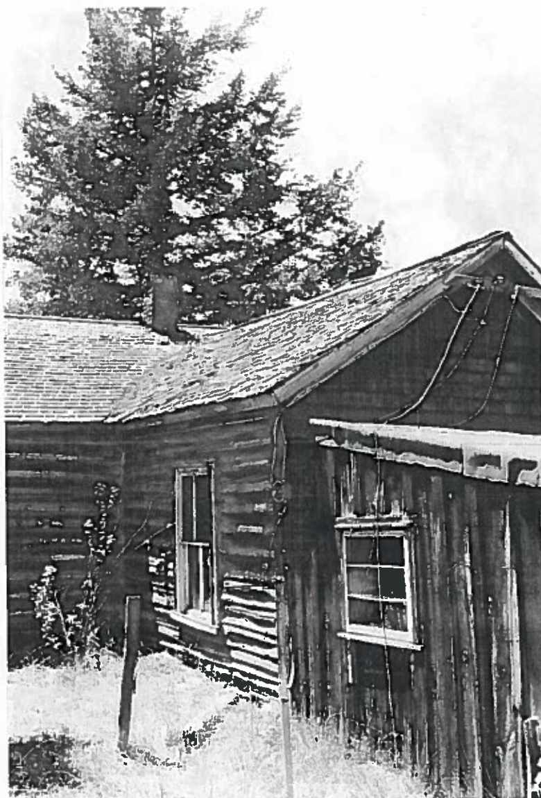
Figure 162: Looking southwest at the intersection of the frame structure and the log structure. Note the high grade around this section of the building.
