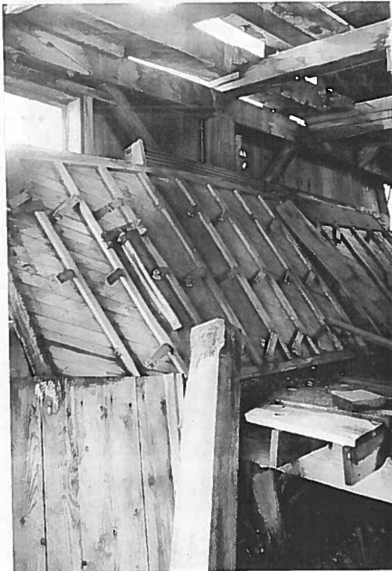
Figure 29: Looking northeast at some of the floatation equipment laying up against the outside wall.
