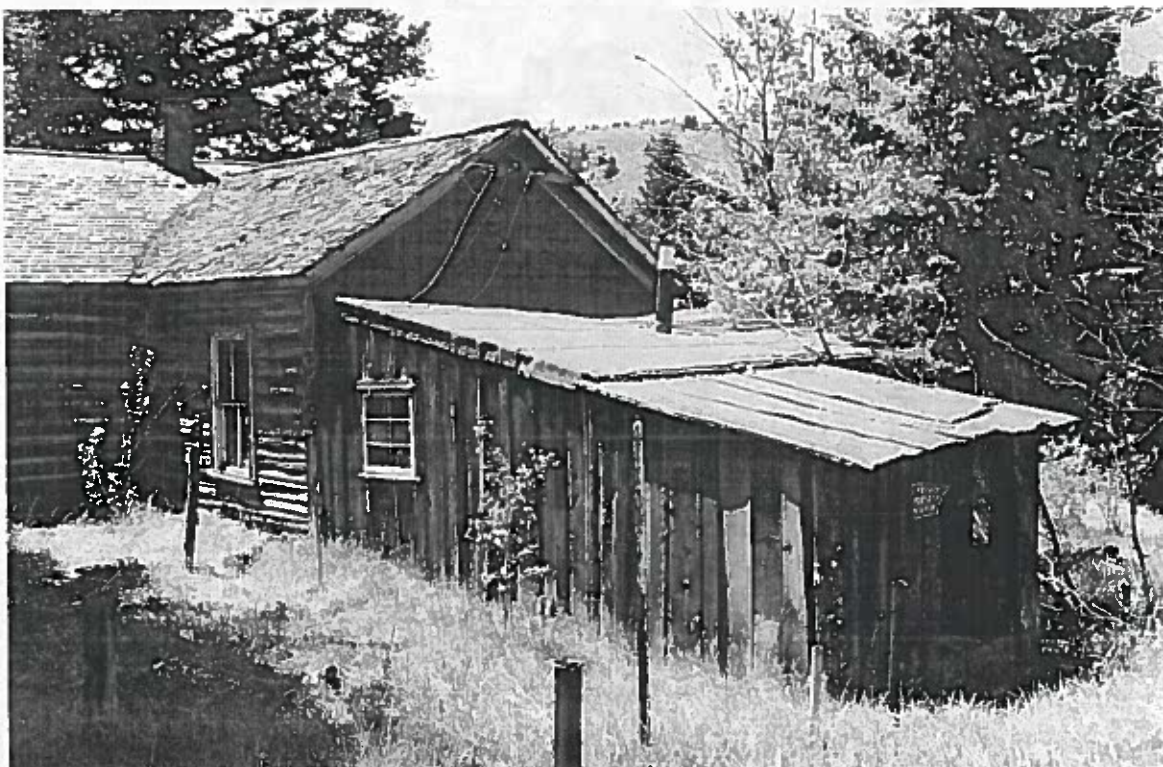
Figure 161: Looking southwest at the frame addition to the building. Note the metal and sheet asphalt roofs which are in fair condition.
