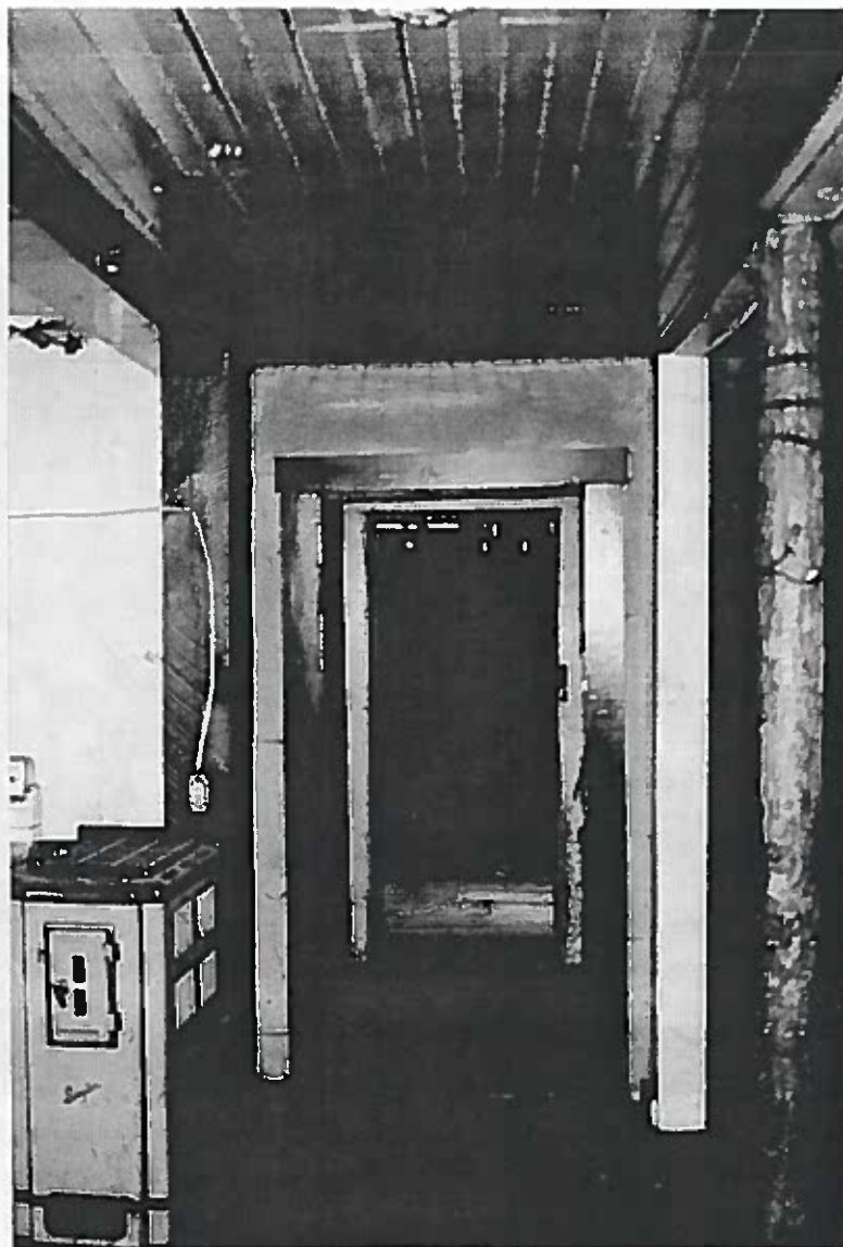
Figure 142: Looking west at the hallway from the kitchen to the dining room. Note the beaded board ceiling which appears to be original.
