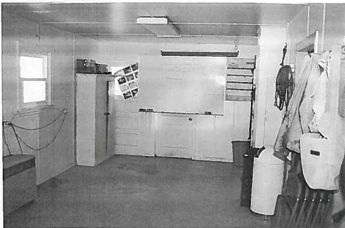
Figure 243: Looking east at the interior of the main room. The materials are in good condition with some minor wear.
