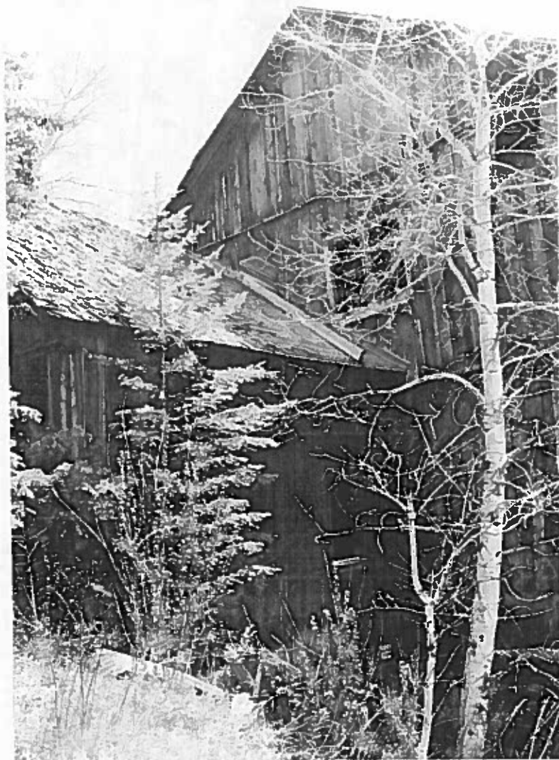
Figure 19: Looking southeast at the upper end of the Mill near the ore bins and the boiler area. The materials are very similar all around the building.
