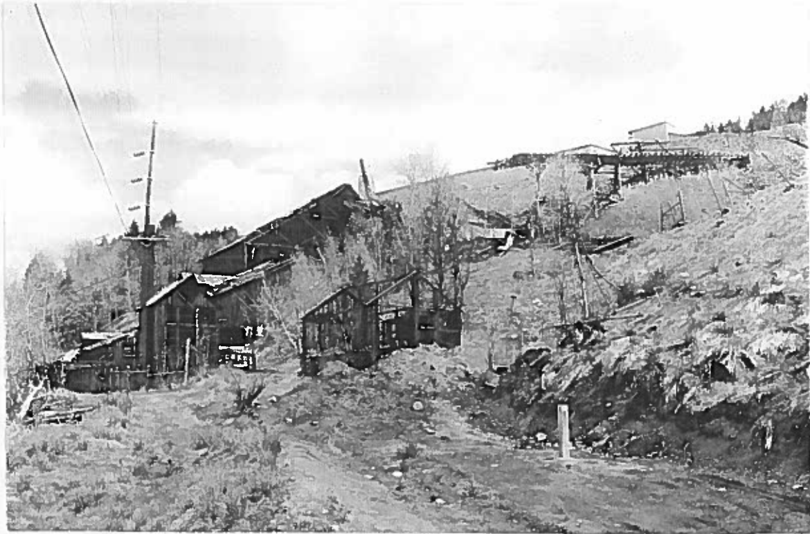
Figure 6: Looking northeast at the Revenue Mill area. Note that the upper parts of the ore bin and the connection to the tramway have collapsed.
