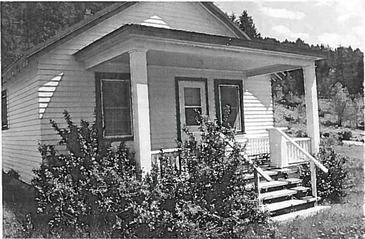
Figure 253: Looking southeast at the porch which appears to be in good condition.
