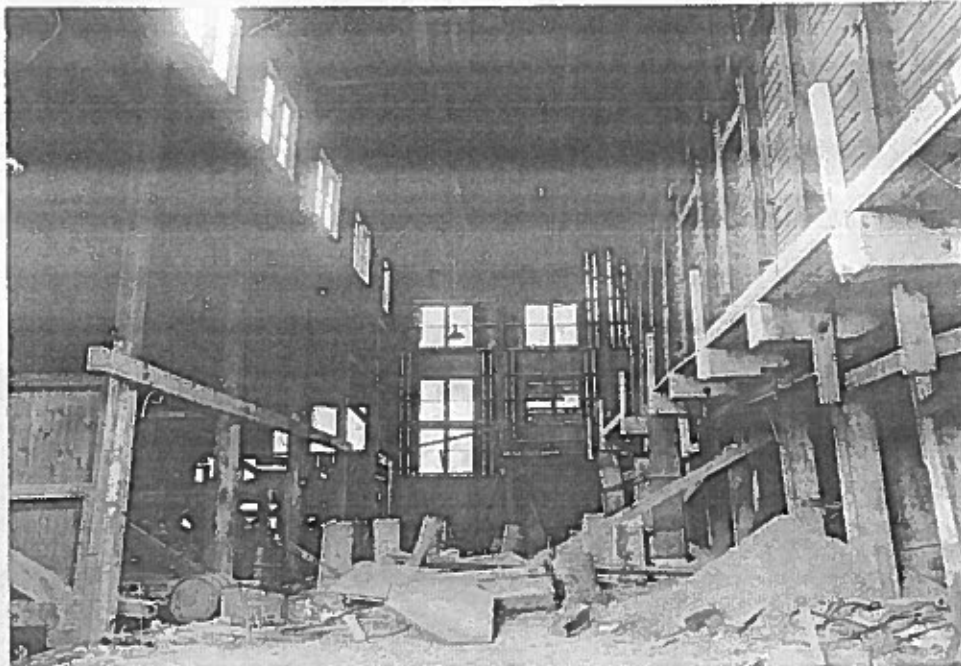
Figure 33: Looking north at the stamp and ball mill area in this 1982 photograph. Note the ore bins to the right.
