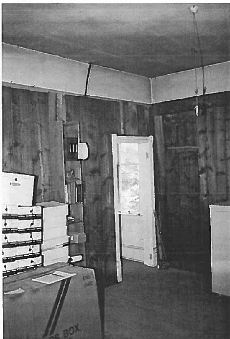
Figure 58: Looking northeast at the front room where it enters into the kitchen. The siding is from the mill and other buildings around the site. It is hard to determine the condition of the plaster behind the siding. The wood floor is worn but in good condition.
