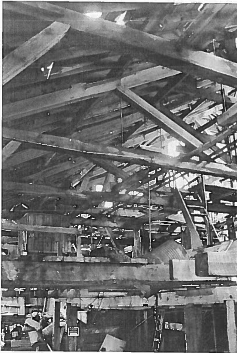
Figure 31: Looking northeast at the wood truss structure over the floatation area. The trusses appear to be intact and in good condition. There is some minor rot in the wood because of holes in the roof however it does not appear to be a problem.
