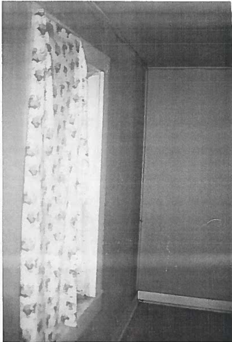
Figure 168: Looking west at the southwest bedroom. Note the good plaster on the walls and ceilings.
