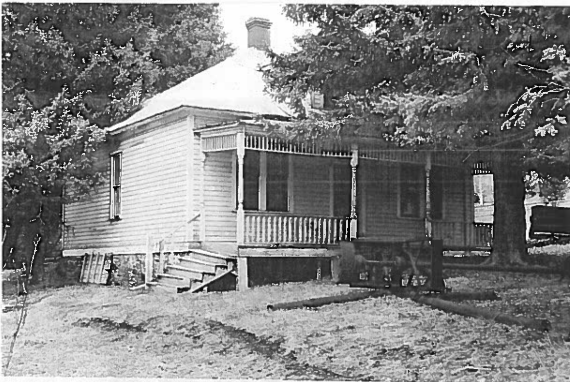
Figure 45: Looking northeast at the Bush Guest House. The materials are generally in good condition.
