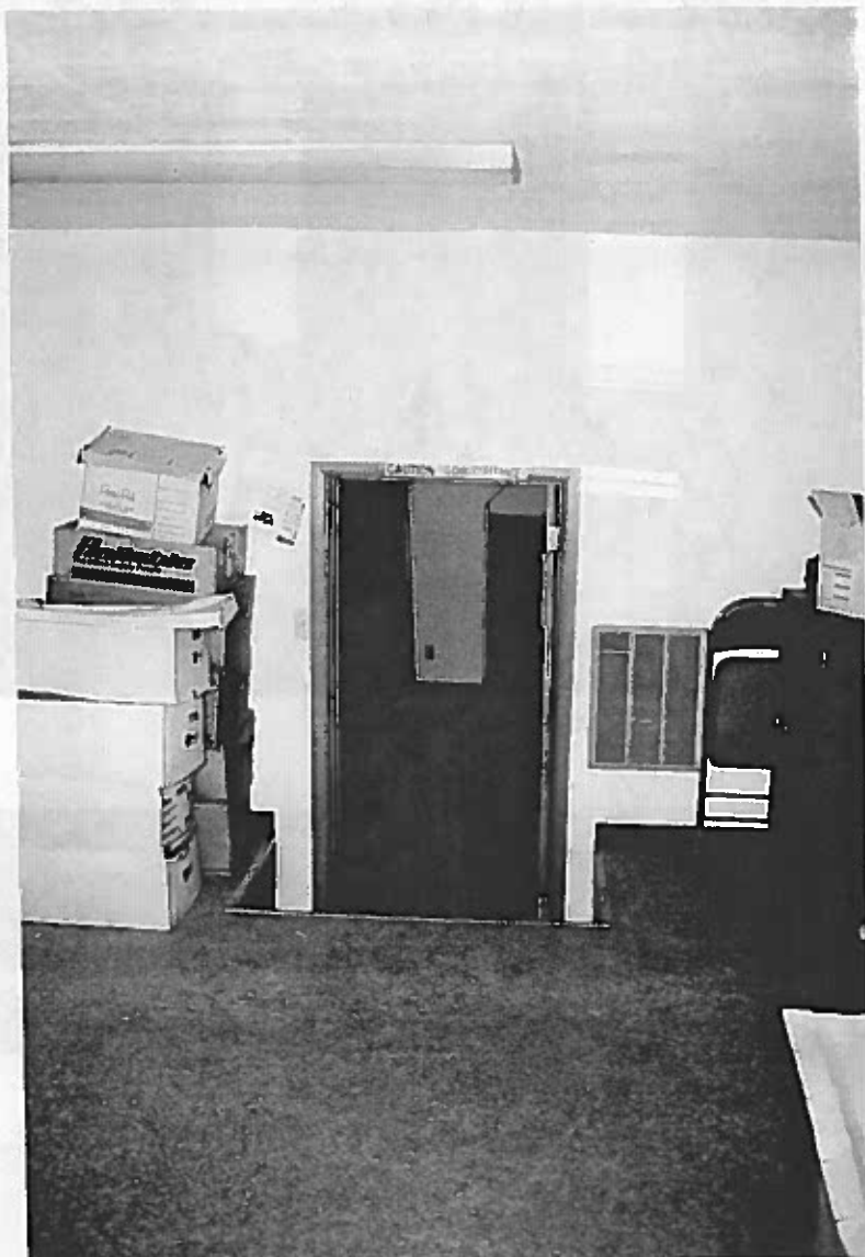
Figure 96: Looking west at the steps and doorway to the original building.
