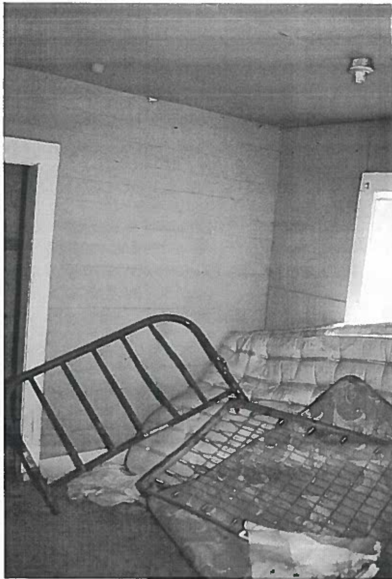
Figure 229: Looking northeast at the bedroom area. The celotex materials on the walls and ceiling are in good condition although they are later materials.
