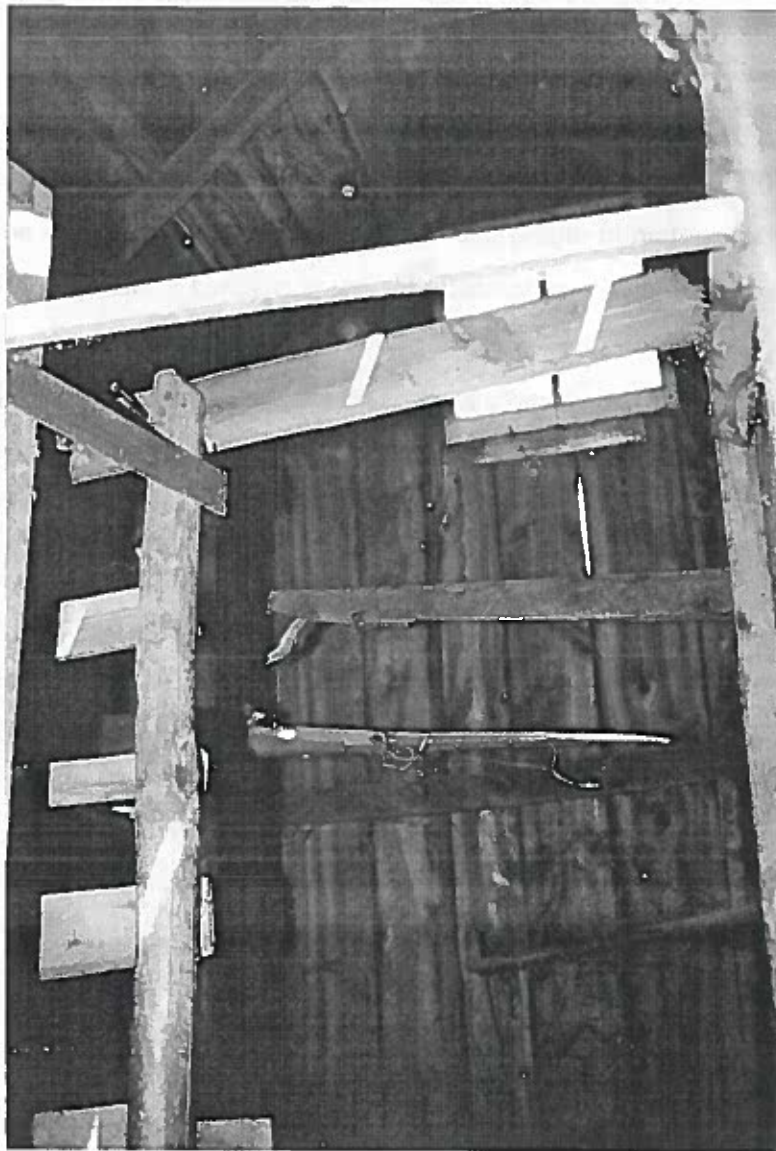
Figure 233: Looking north at the wood frame wall with wood boards on the exterior wall.
