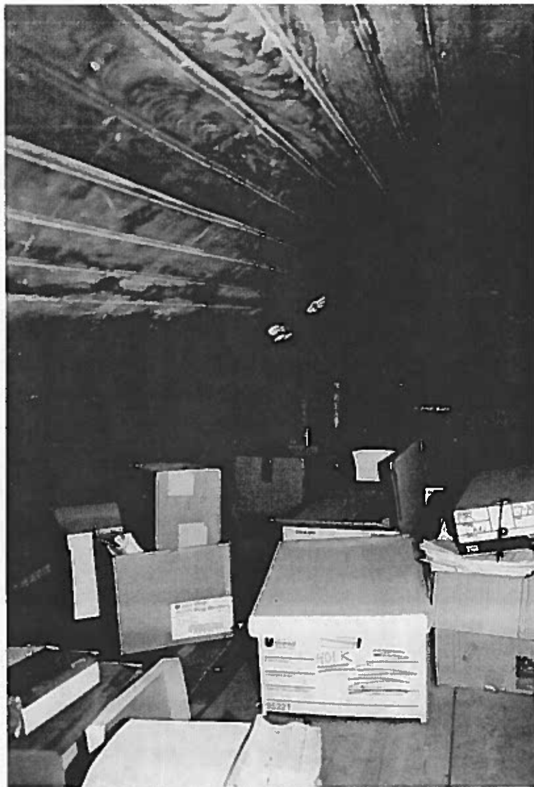
Figure 99: Looking east at the unfinished attic space used as storage.
