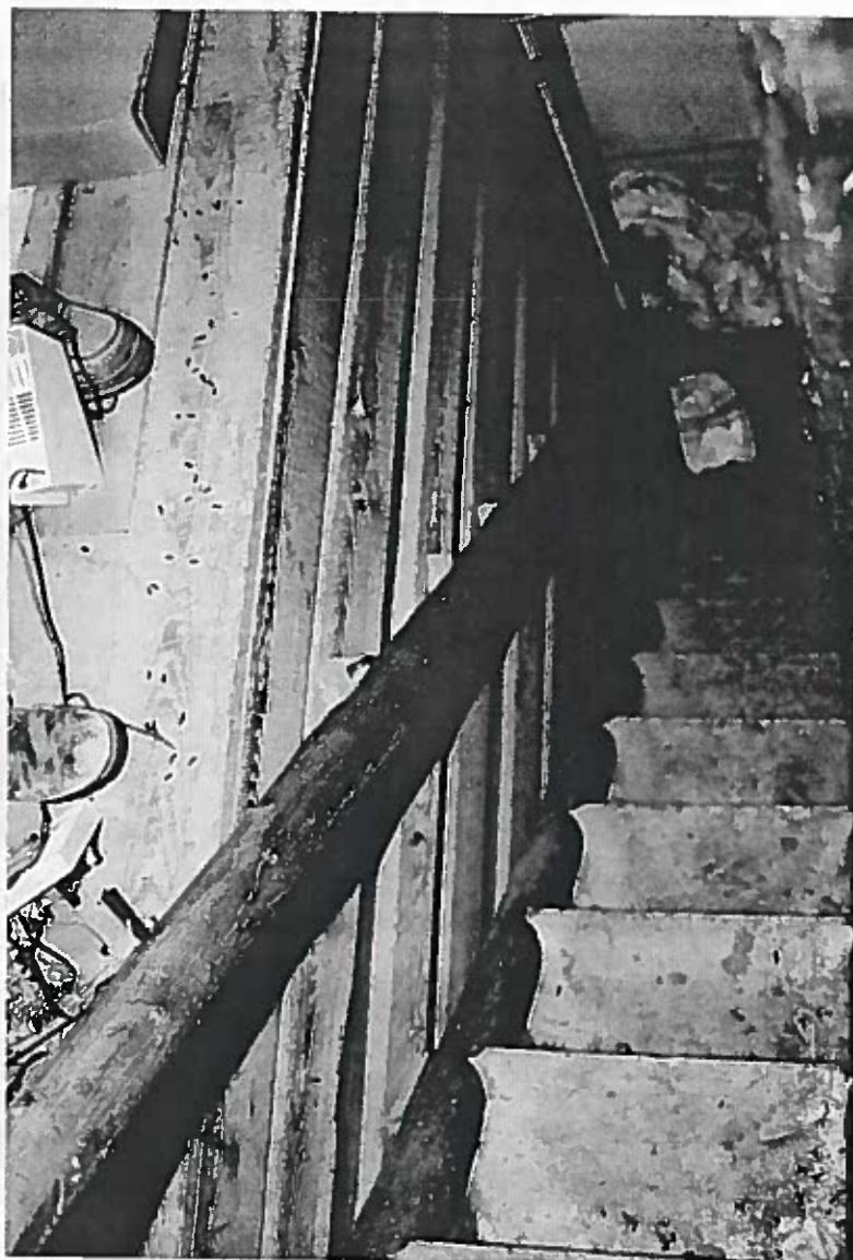
Figure 150: Looking down the stair to the first floor from the attic.
