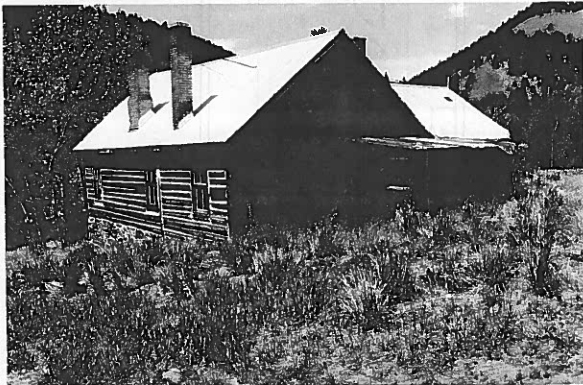
Figure 119: Looking northwest at the house. Note the galvanized metal roof which is covering the original wood shingle roof. The brick chimneys have some brick and mortar deterioration at the tops. The materials are generally in good condition.
