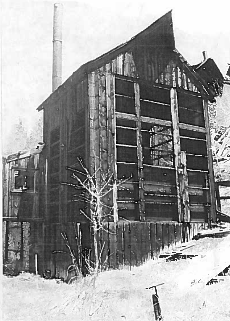
Figure 8: Looking northeast at the coal bin for the lower boiler. Note the wood structure and siding which is in good condition. There is some rot at the bottom of the structure where the grade is against the building.
