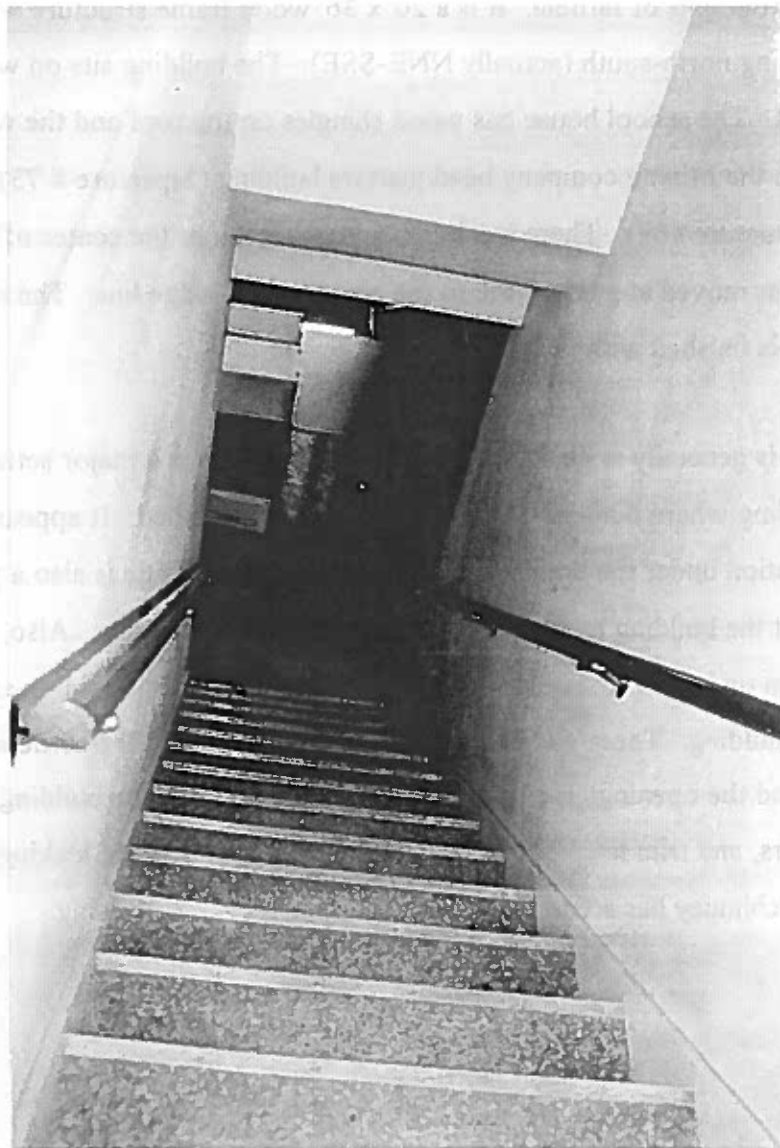
Figure 101: Looking south down the stairway to the first floor from the attic.
