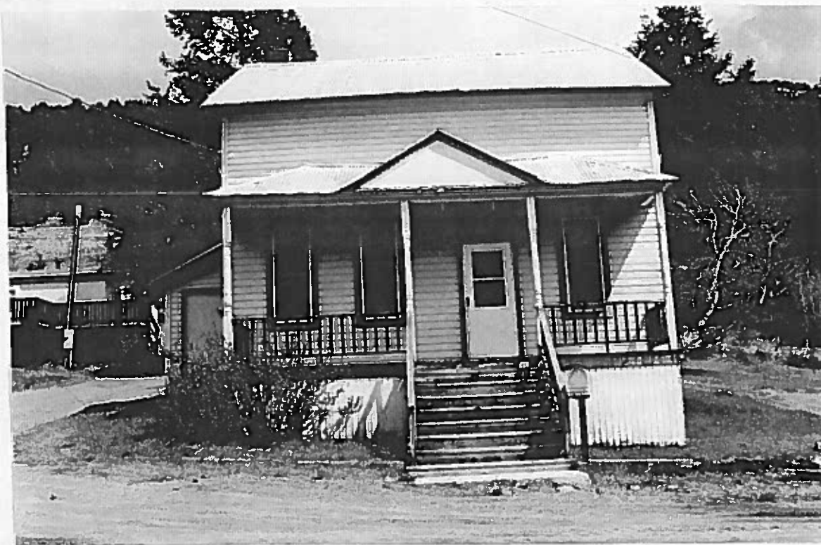
Figure 69: Looking east at the front of the Company Headquarters building. Note that the front porch steps are offset thus the columns are offset. It appears that the porch was rebuilt and the steps moved over.
