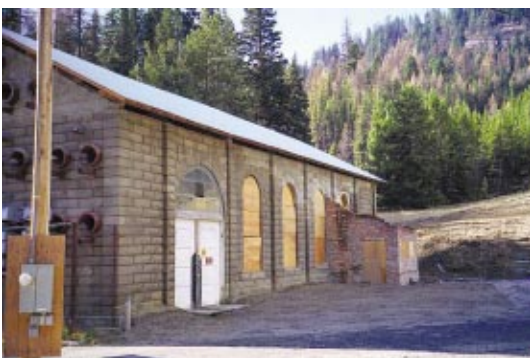
Fremont Powerhouse before and after restoration, Grant County, 1908
