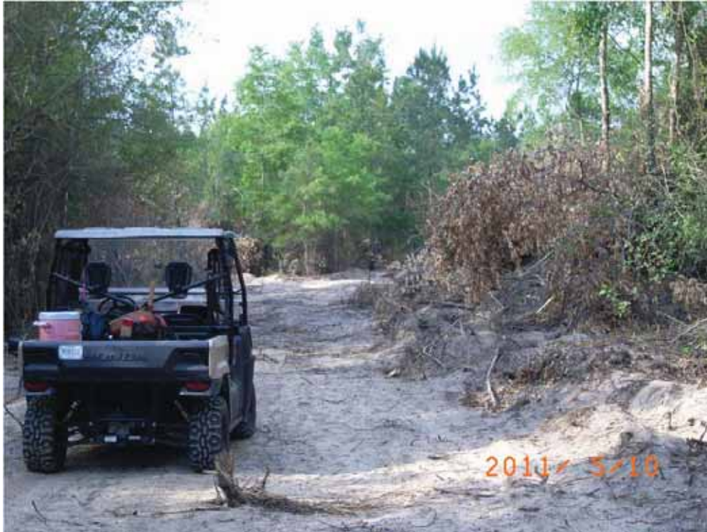
Photo 3. Vegetation pushed to the side from dozer line construction.
