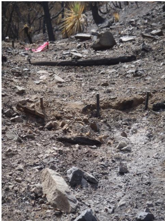
Looking up trail at burned wooden structures
