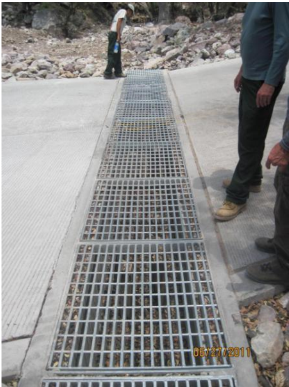
Concrete Hardened Low Water Crossing with Slotted Grates
