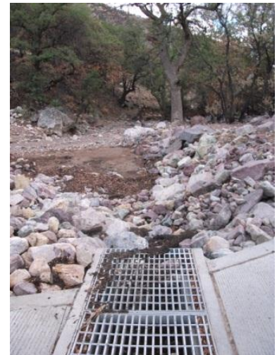
3 rd Low Water Crossing draining into Montezuma Wash
