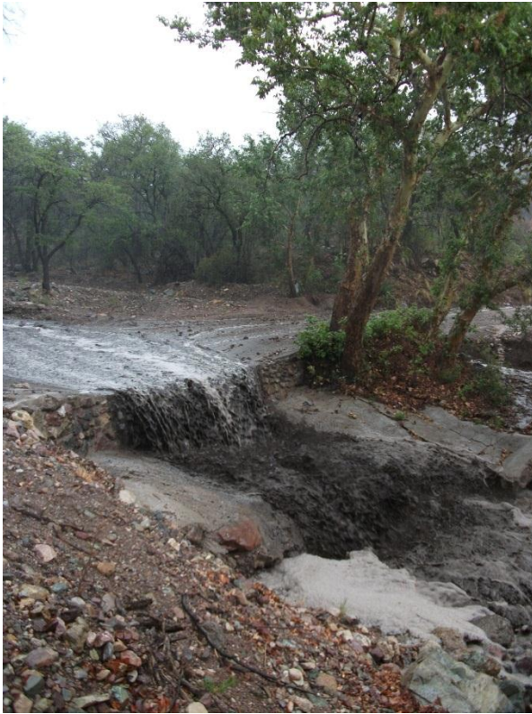
First crossing after 07/20/2011 storm
