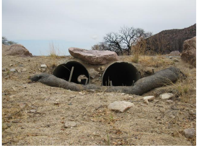
Looking south on 3 Mile Wash
