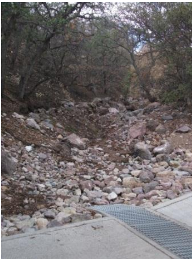
3 rd Low Water Crossing looking south
