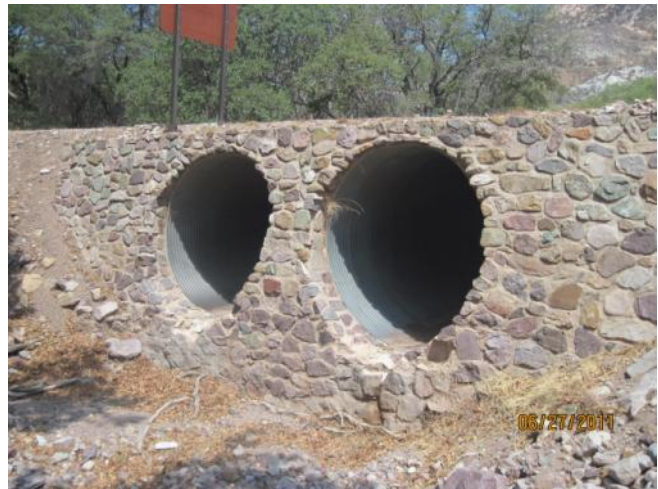
Outlet View of the Nine Feet Diameter Culverts
