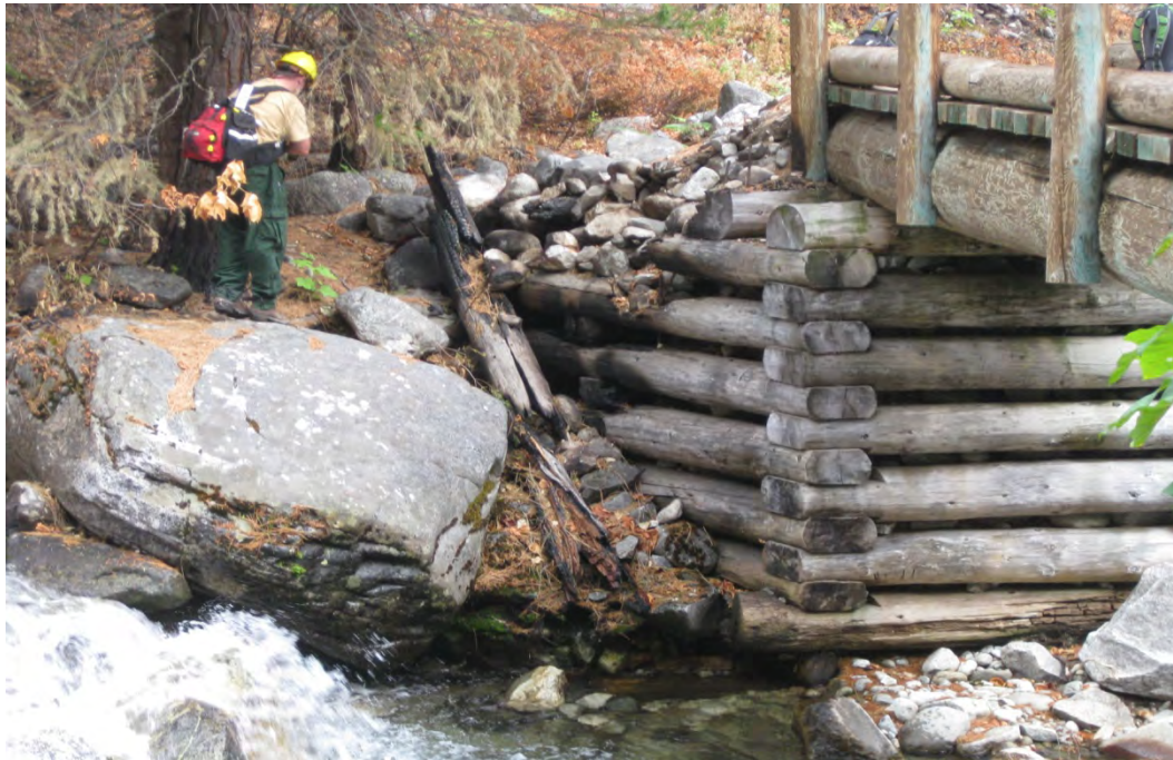
Photo 6. Crib wall of Rainbow Creek bridge.
