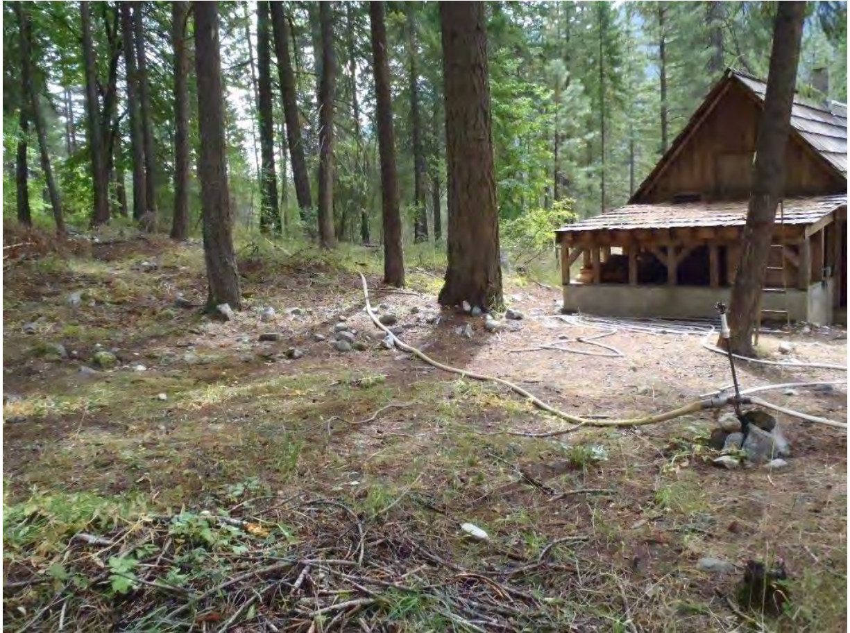
Photo 10. The back of the Stehekin School, showing the sprinkler hose layed during the Rainbow Bridge Fire.
