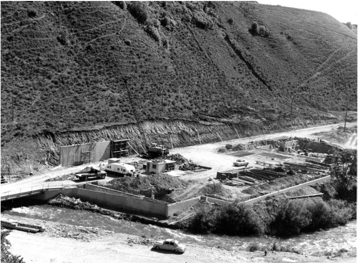
Excavation and foundation work for the Utah Water Research Laboratory, located below First Dam on the Logan River along the old Logan Canyon road. Engineers considered the site to be one of the most optimal sites in the western United States for this research.
