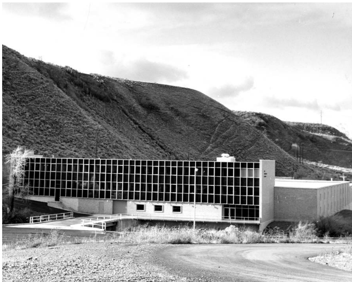
Designed by Kenneth W. Jones and built by Olsen and Davis Construction Company, the Utah Water Research Laboratory was dedicated on December 6 and 7, 1965. In August 1982, USU posthumously named the facility in honor of George Dewey Clyde.
