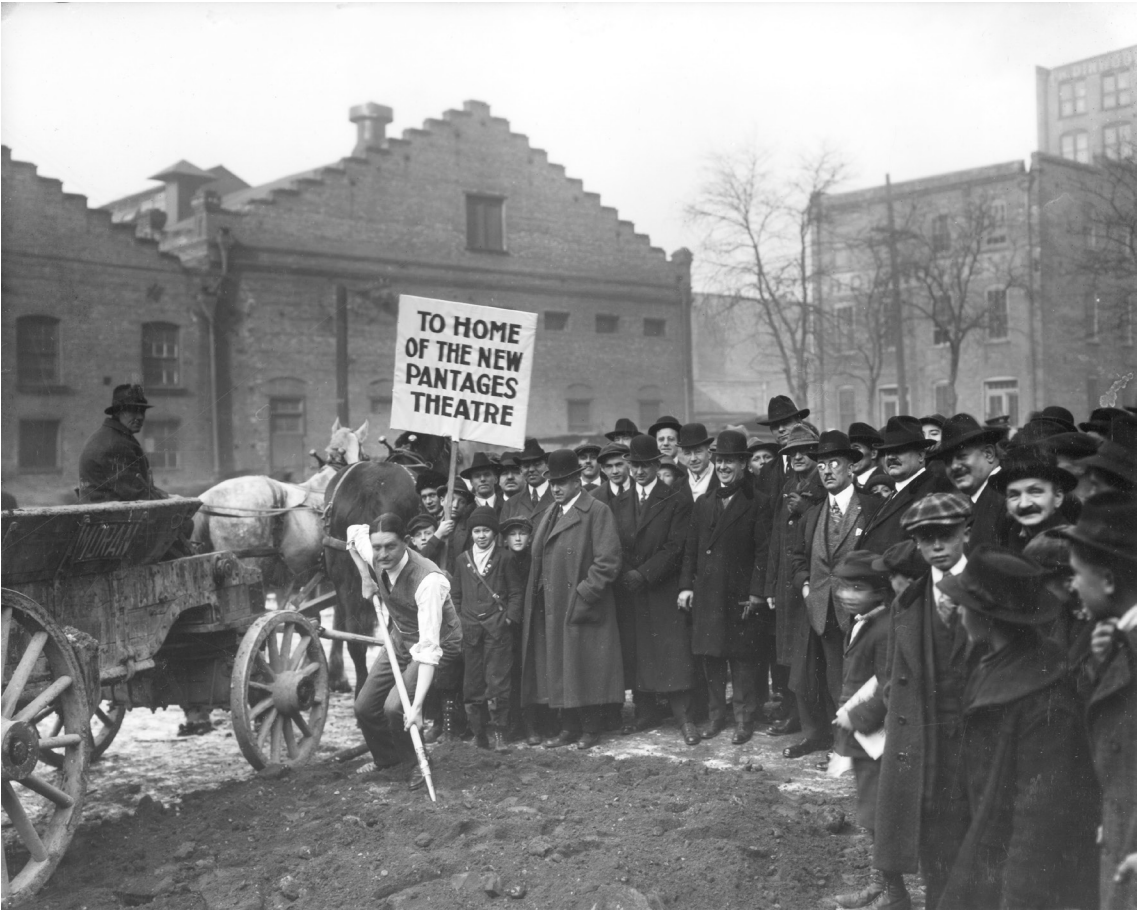
Groundbreaking for the Pantages Theater at 148 South Main took place on December 3, 1918, less than a month after the November 11 armistice ending the war in Europe. Construction of the theater was delayed because of questions regarding the appropriateness of using scarce material and manpower during the war.
