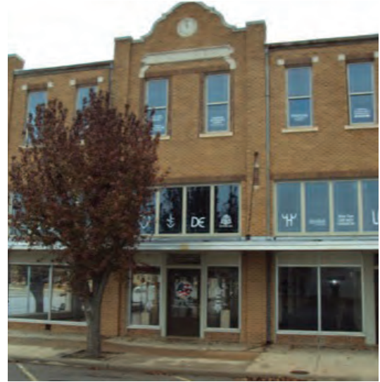
Stanley Building, Hobart. Photo: Hobart Main Street
