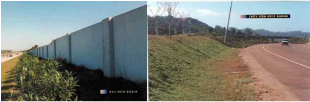
Figure 5: Example Noise barrier (left) and berm (right) (FHWA, 2011)
