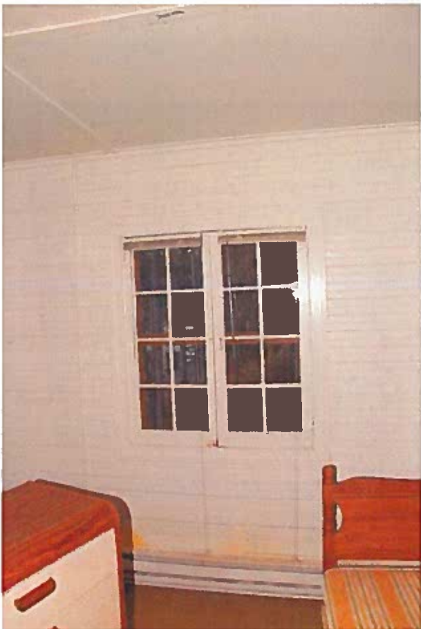
Figure 73: Typical double wood hinged window which occurs throughout the building.
