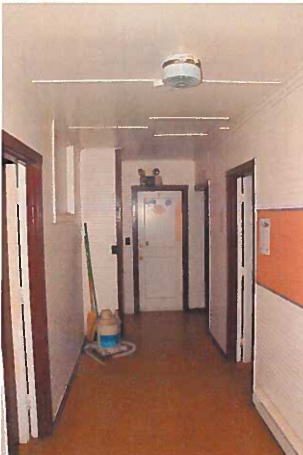
Figure 69: Note the typical hallway with doors to the bedrooms. The sheetrock ceiling is good.
