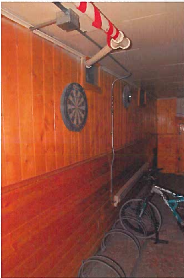
Figure 33: A wood partition wall is in good condition.
