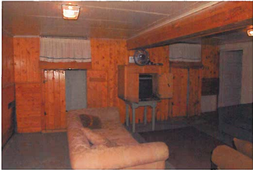
Figure 34: Knotty pine paneling is located on the south and west sides of the main room. It is in fair to good condition. The celotex ceiling is in good condition.
