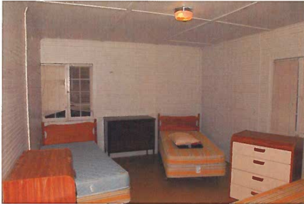
Figure 70: The painted wood bead board walls are in good condition with some minor wear. The sheetrocked ceiling has wood battens covering the joints. The windows are generally in good condition from the inside.
