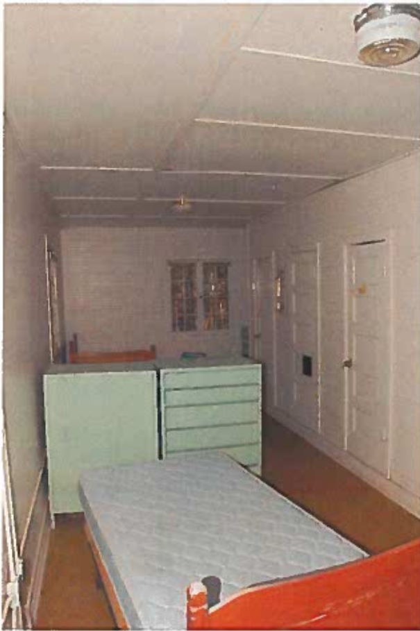
Figure 80: This room sees a lot more wear because of the number of tenants in the space.
