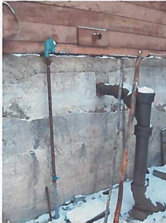
Sanitary Sewer Exiting Building
