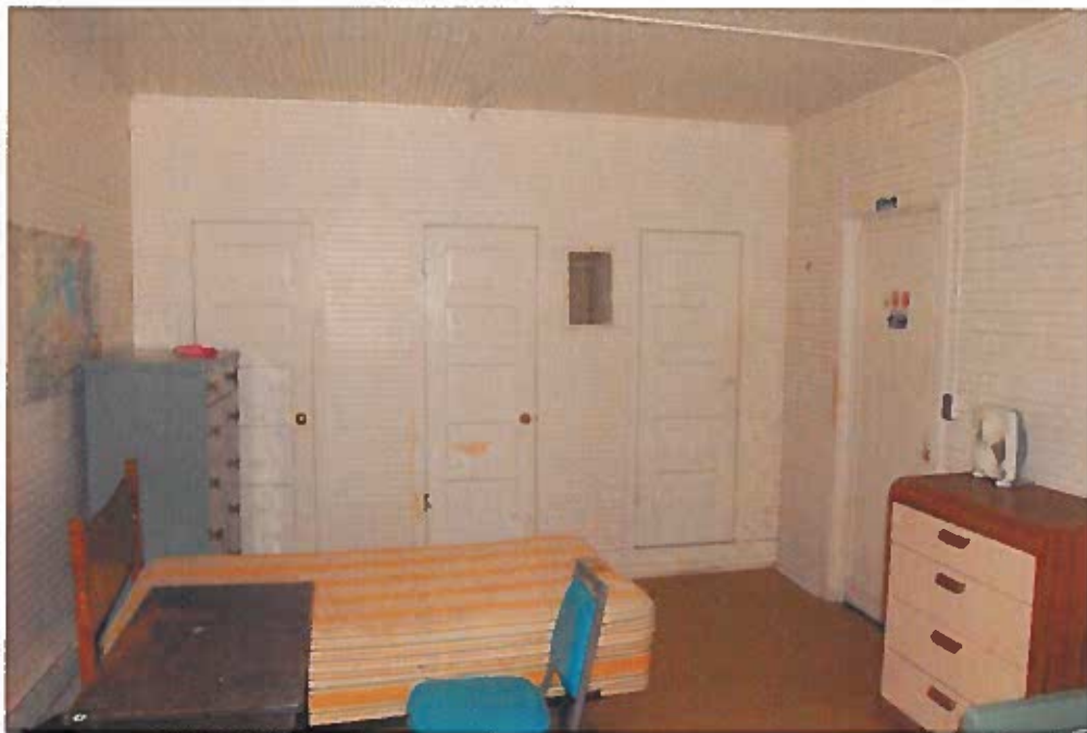
Figure 59: The painted woodwork and wood bead board walls are in good condition with some minor paint wear. Note the covered lite on the door to the right.
