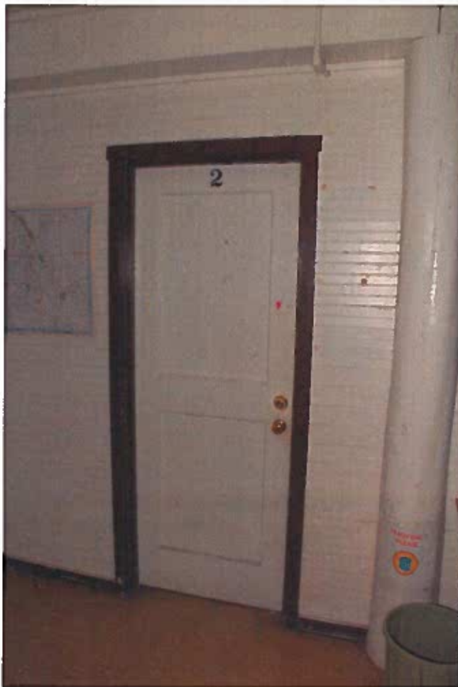
Figure 53: The original wood paneled doors still access all of the rooms.
