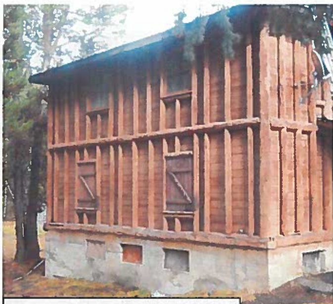
Typical Log "Stud" & Planking Wall – Three Sides
