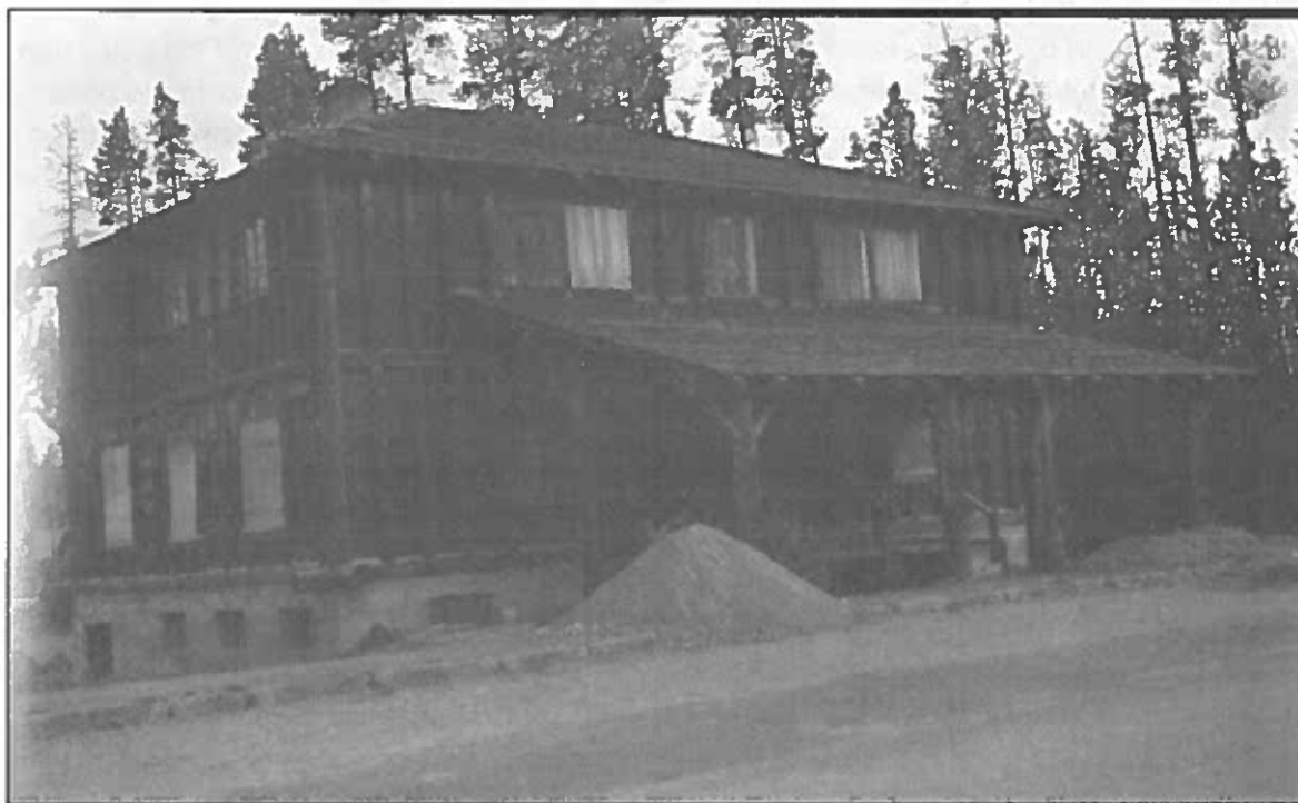
Figure 2. Undated photograph of the original porch (Courtesy Yellowstone National Park Photo Archives, YELL 29938)
