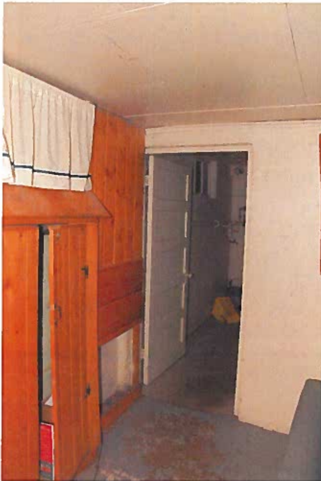
Figure 36: Entering the laundry area from the rec room. The wood panel door is typical of the upper areas. There is no second exit out of the basement.
