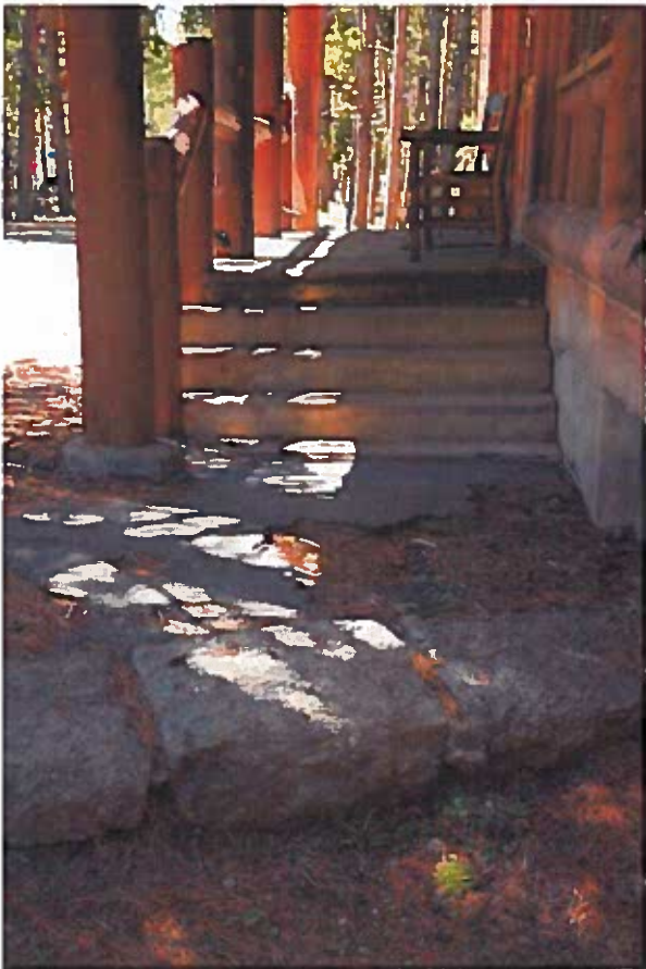
Figure 30: Looking west at the porch. Note the change in the railing and slope of the pathway into the window well.
