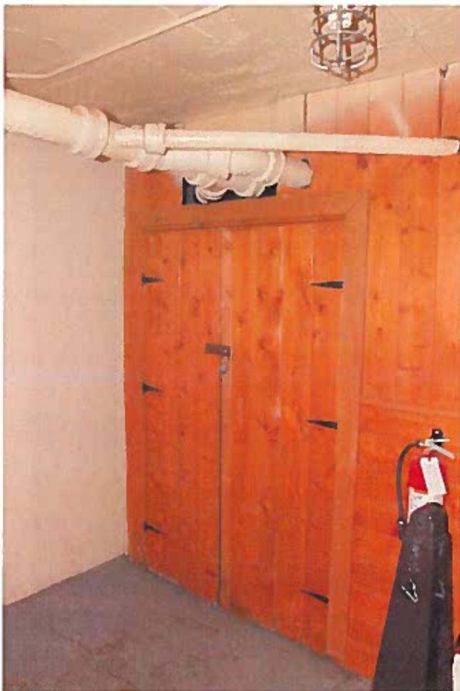
Figure 41: Entrance to the mechanical room. The wood is in good condition.
