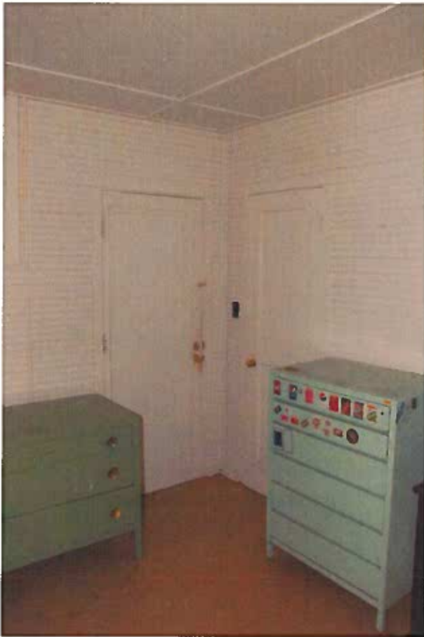
Figure 86: The materials are generally in good condition.
