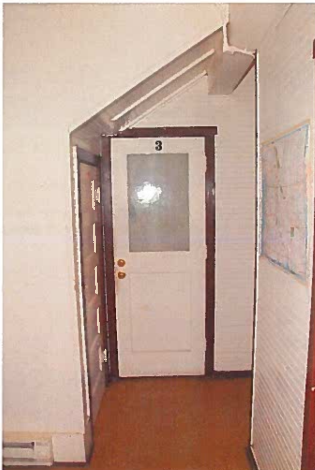
Figure 58: The original door has a half-glass lite and is covered over from the inside.
