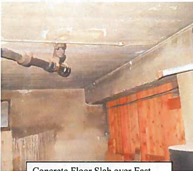
Concrete Floor Slab over East Side Storage Room
