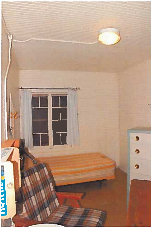
Figure 49: Room number 1 is generally in good condition. Note the missing muntins in the window. Also note the exposed electrical conduit.
