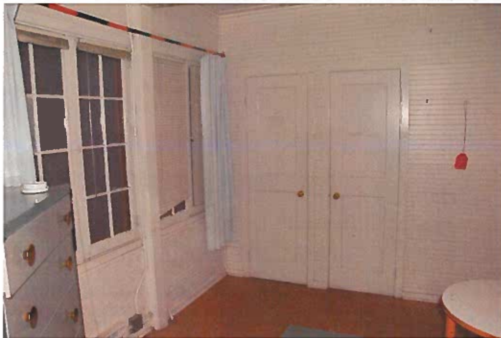
Figure 50: The painted woodwork and beaded wood walls are in good condition with some minor wear.
