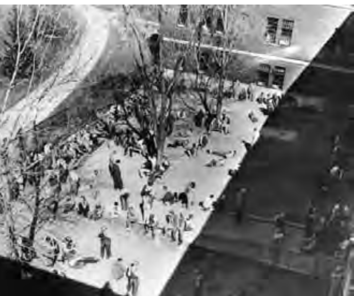
This courtyard was located behind the Dunn Building and was modeled after a prison exercise yard, without out the armed guards, c. 1935. (Utah State Hospital Museum Collection)
