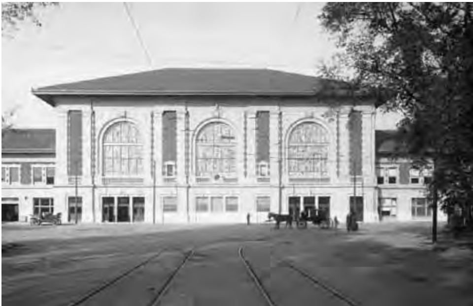
The D&RG Depot was finished in 1910 at a reported cost of about eight hundred thousand dollars.
