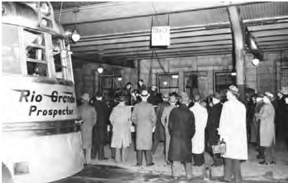
After World War II, railway passenger service gradually declined. The new Interstate Highway systems and commercial aviation competed to facilitate economic failure for many railroad lines. In consequence, railroad stations, the D&RG Depot included, fell into disrepair and faced the threat of demolition.
