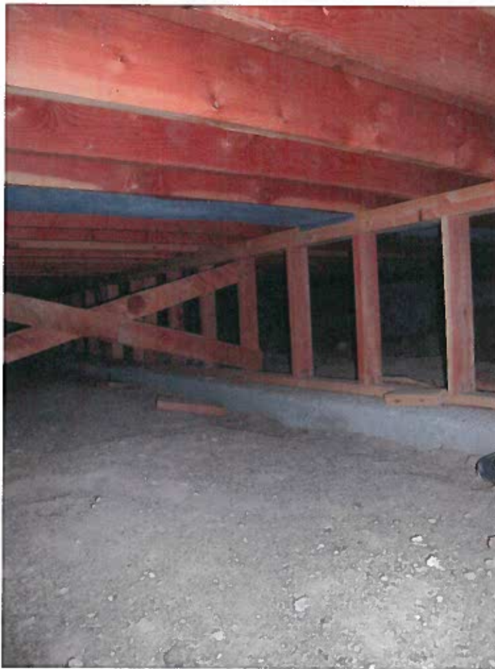
CRAWL SPACE BENEATH RETAIL WING
