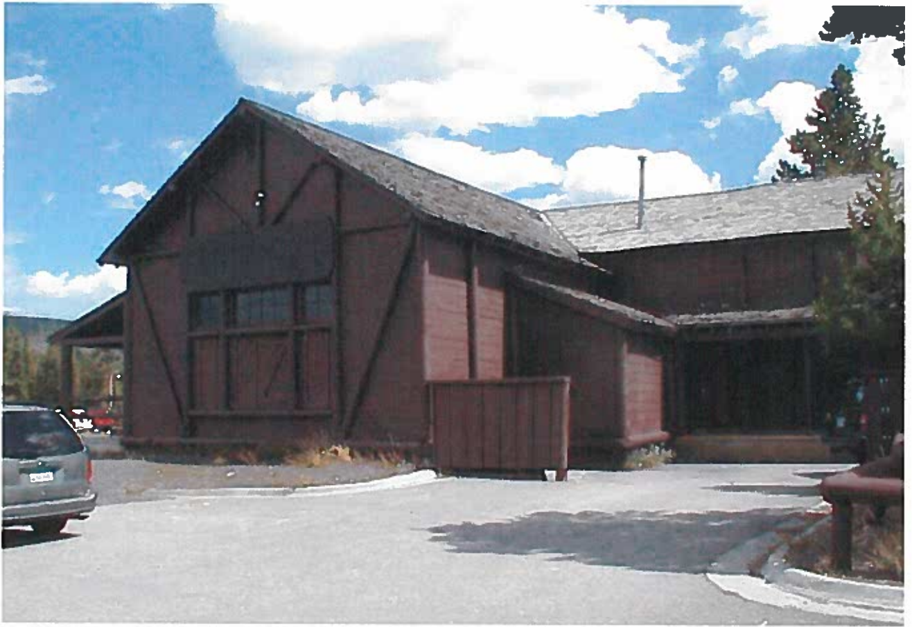
WEST ELEVATION - SIDE ENTRANCE/EXIT AND FORMER DELIVERY ENTRY INTO STRUCTURE
