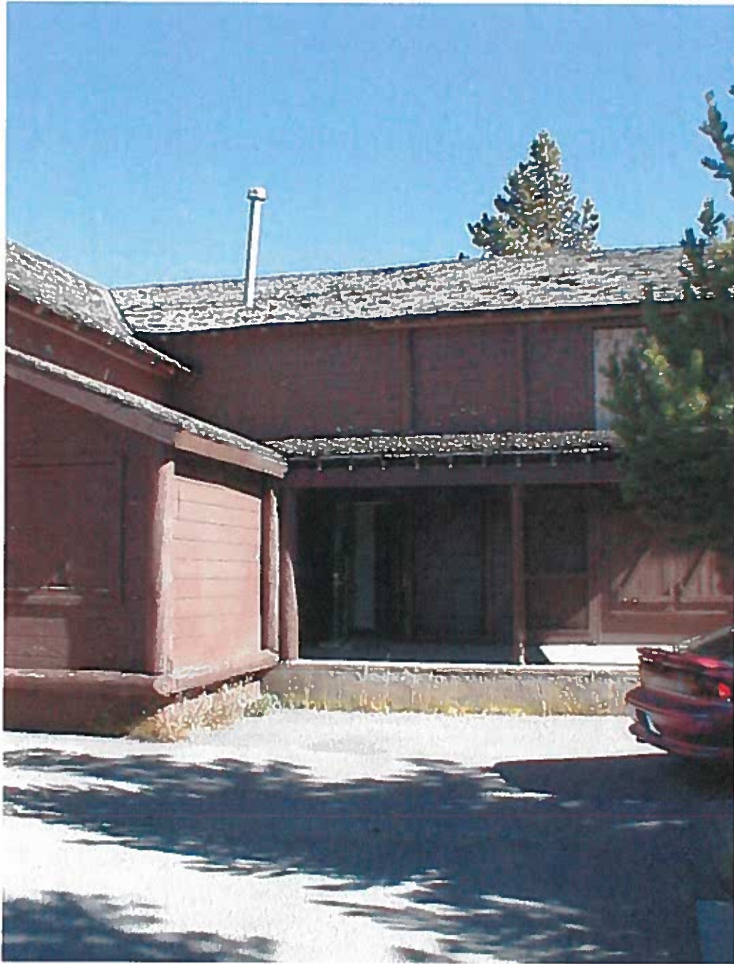
CLOSE-UP VIEW OF SIDE ENTRANCE/EXIT AND FORMER DELIVERY ENTRY INTO STRUCTURE
