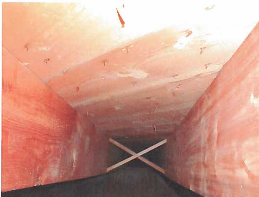
NEW FLOOR SYSTEM BENEATH DORMITORY WING
