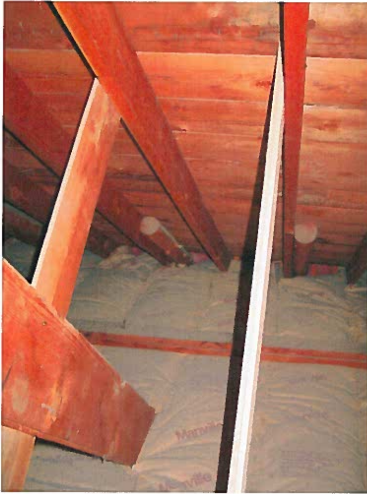
RETAIL WING - PATTERN OF WOOD BRACES AND TIES WITHIN THE ROOF FRAMING ASSEMBLY.
