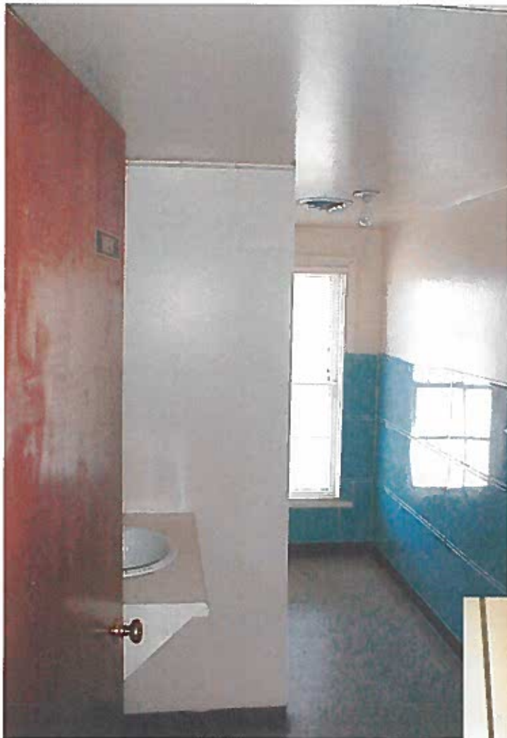
SECOND FLOOR MEN'S ROOM; DORMITORY WING
