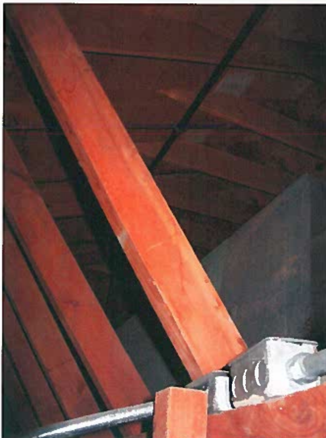
EXAMPLES OF ELECTRICAL BOXES AND CONDUIT WITHIN THE ATTIC OF THE DORMITORY WING.
