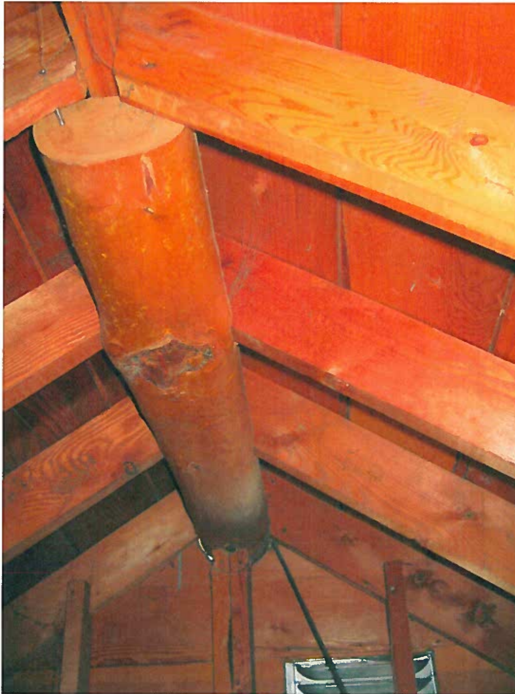
RETAIL WING - ATTACHMENT OF THE DECORATIVE LOG ROOF RIDGE PURLIN THAT CAN BE SEEN FROM THE EXTERIOR OF THE FACILITY.
