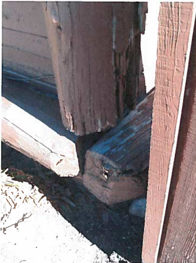
INTERSECTION - APPLIED LOG SILLS AND COLUMN
