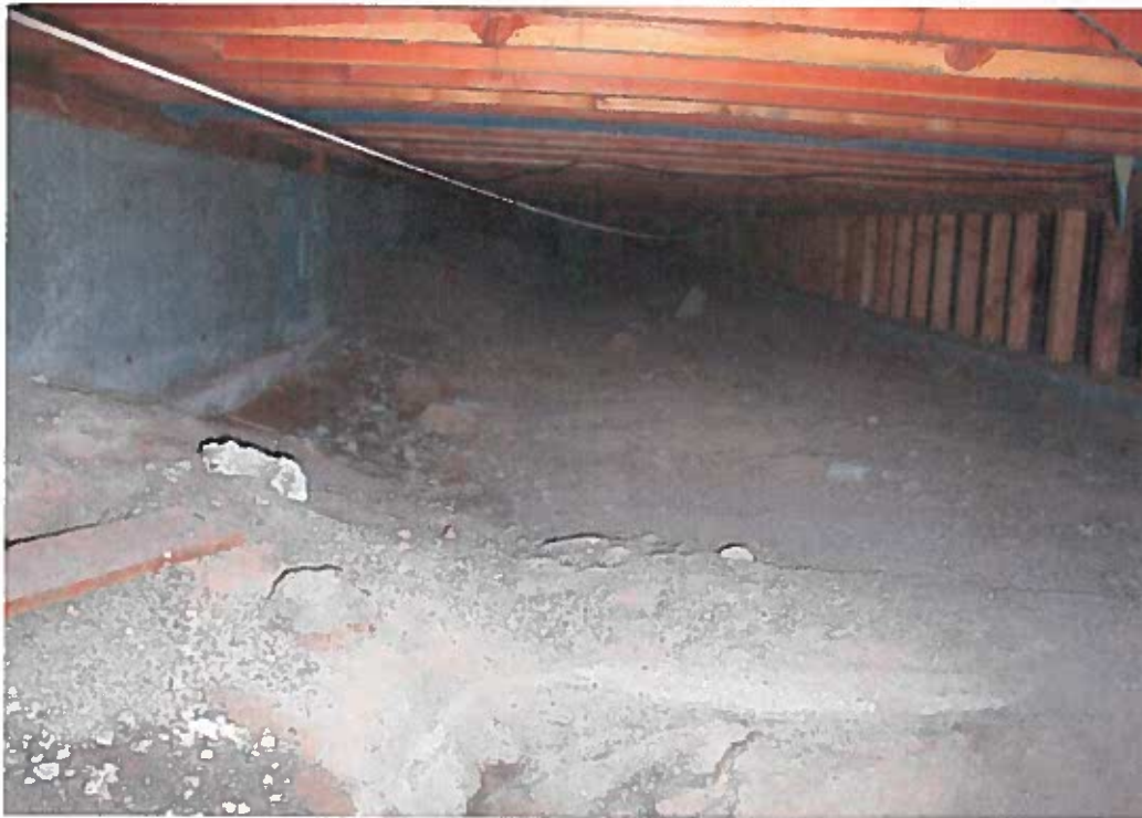
CRAWL SPACE BENEATH RETAIL WING SHOWING NEW REINFORCED CONC FOUNDATION
