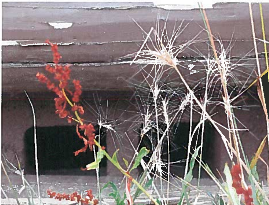
UNKNOWN FEATURE - THIS MAY BE FOR CRAWL SPACE VENTILATION
