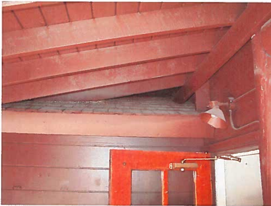
DETAIL OF SIDE (DELIVERY) ENTRANCE; Note hardware & direction of swing.
