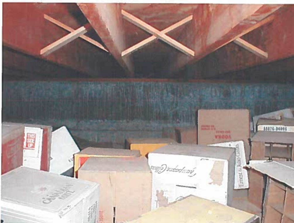
CRAWL SPACE BENEATH DORMITORY WING
