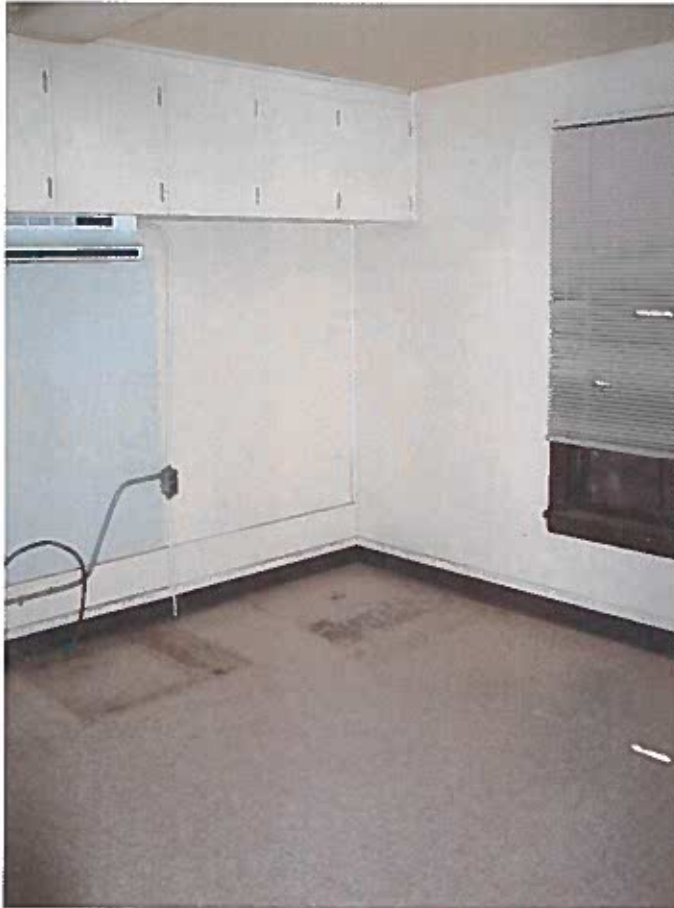
FOOD PREPARATION AREA (WITHOUT EQUIPMENT) - COMMERCIAL KITCHEN AREA - SE CORNER OF DORMITORY WING; FIRST FLOOR
