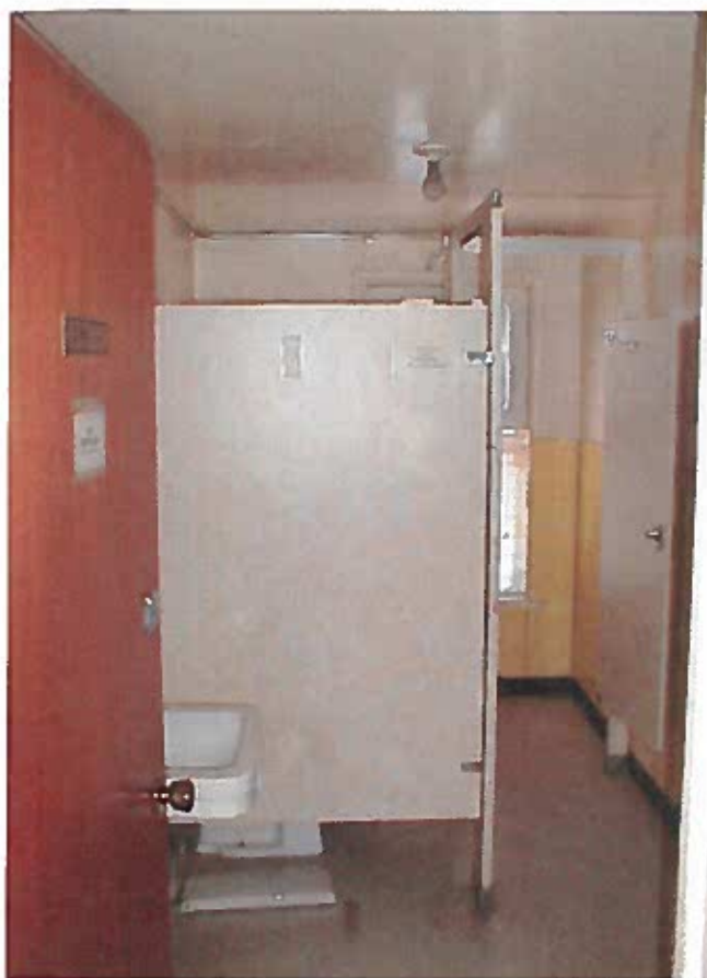
WOMEN'S ROOM - FIRST FLOOR OF DORMITORY WING
