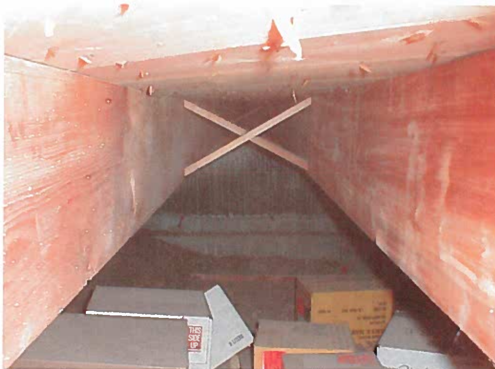
CRAWL SPACE BENEATH DORM WING
