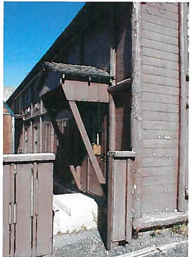
DETAIL OF SIDE (DELIVERY) ENTRANCE; Note hardware & direction of swing.
