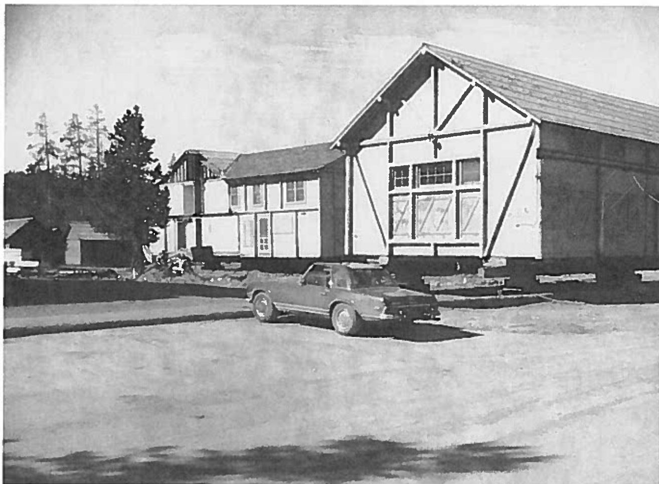
RETAIL WING IN PROCESS OF BEING MOVED TO A NEW LOCATION - 1971
