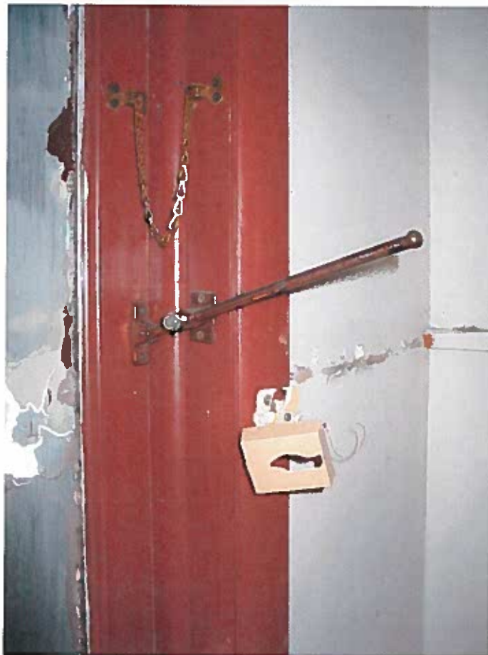
WINDOW HARDWARE AT EXHIBIT/DISPLAY SPACE
