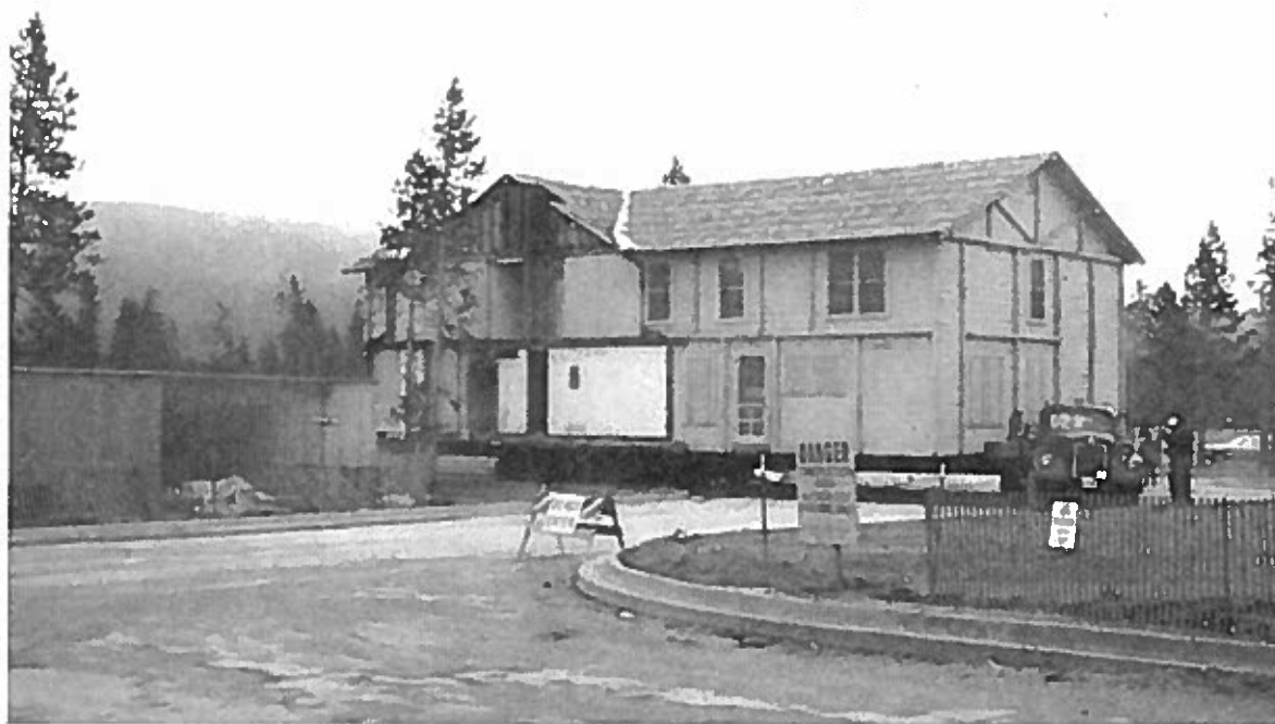
DORMITORY WING IN PROCESS OF BEING MOVED TO A NEW LOCATION - 1971
