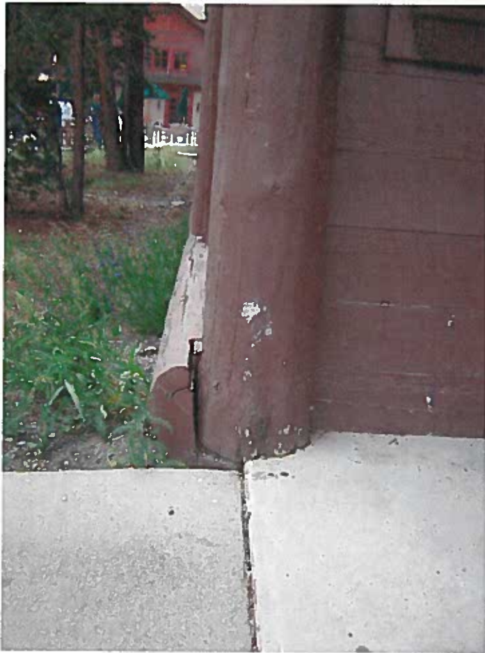
INTERSECTION - APPLIED LOG SILLS AND COLUMN
