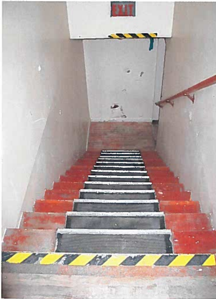
VIEWS OF THE CENTER EXIT STAIR BETWEEN THE TWO FLOORS OF THE DORMITORY WING.
