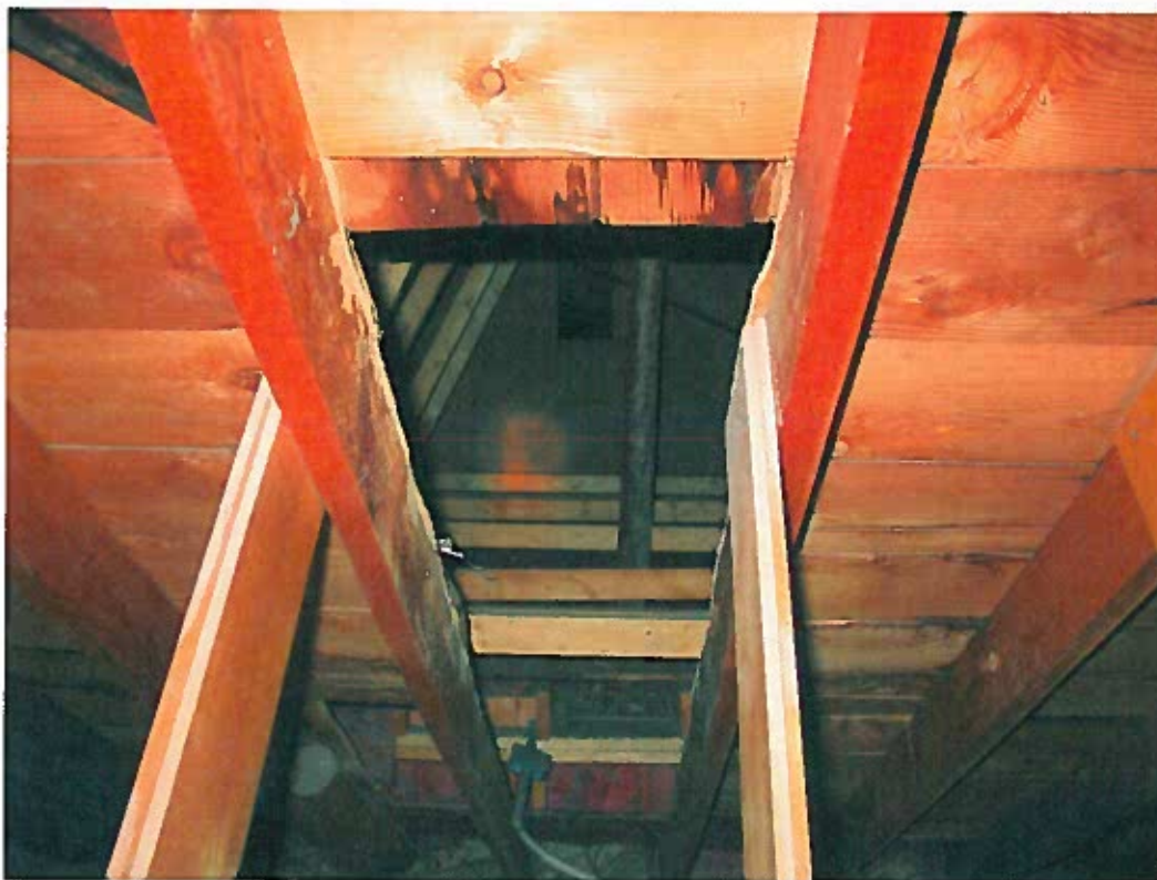
ACCESS HATCH IN ROOF BETWEEN RETAIL WING AND DORMITORY WING OF ATTIC STRUCTURE.
