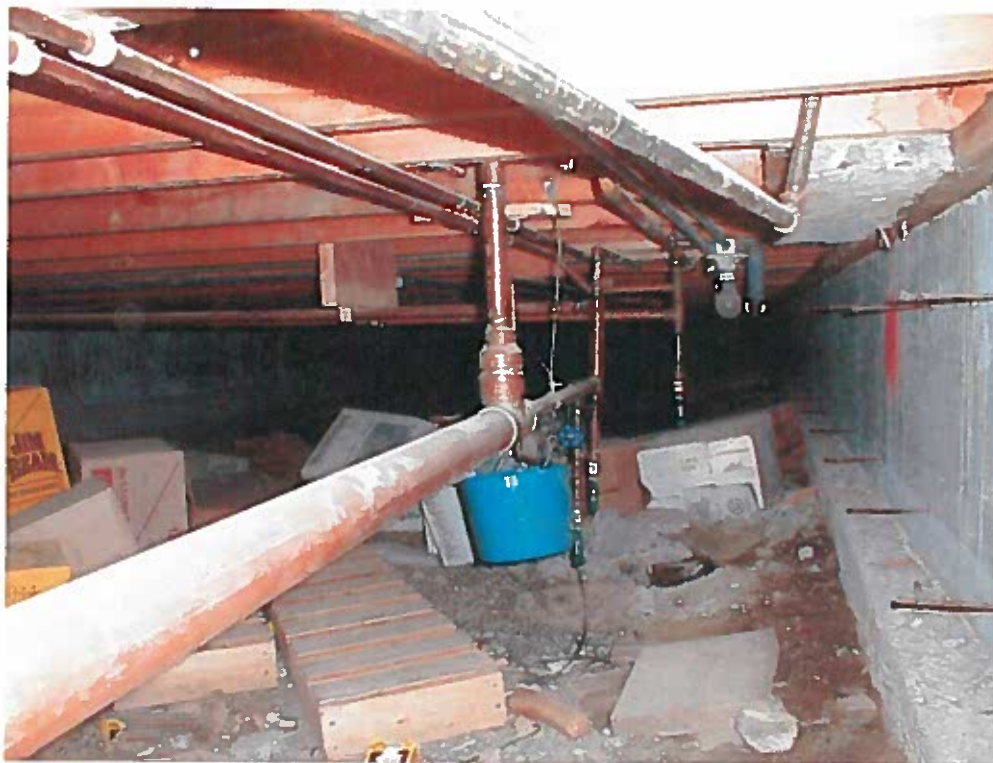
CRAWL SPACE BENEATH DORMITORY WING
