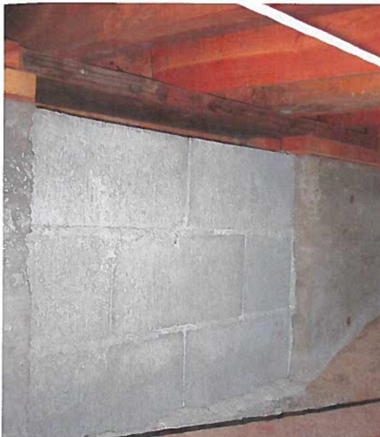
REMOVEABLE PANEL IN NEW FOUNDATION WALL.
