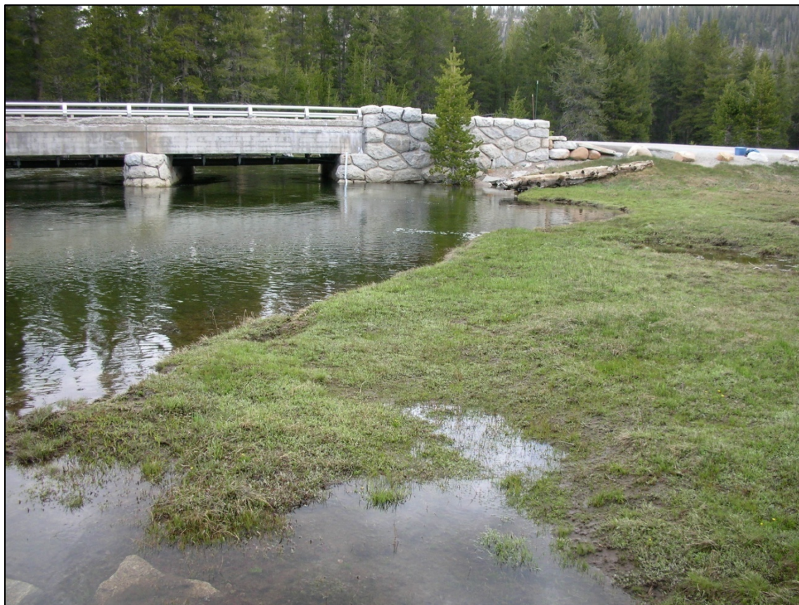
Figure 1.2. Tuolumne River at Tioga Road site. The view is facing downstream.
