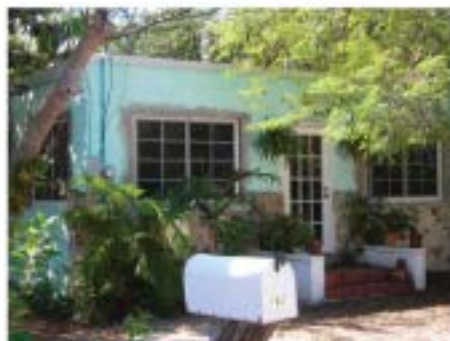
162 Sunrise Drive Facade Facing South
