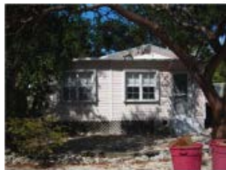
Facade of 185 Lowe Street Facing North
