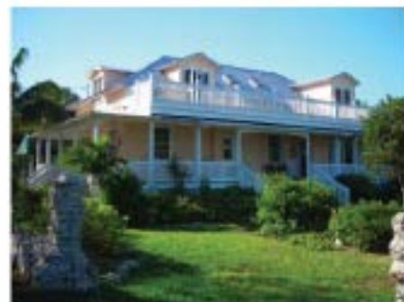
200 Beach Road Facing Northwest
