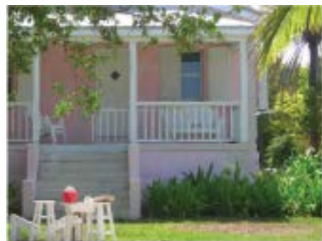
Ballast Trail Facing East
