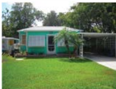
122 Lowe Street Facing Southwest
