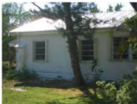
240 Lexok Avenue Facing Southwest
