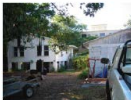
204 Ocean Boulevard Facing Northwest
