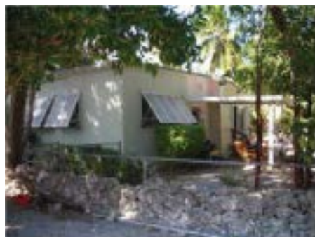
195 Lowe Street Facing North
