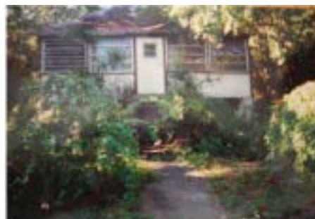
140 Sunrise Drive Facade Facing Southwest in 1994
