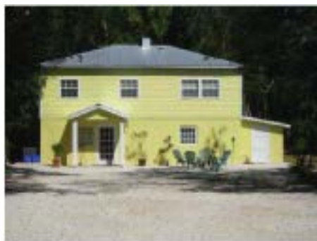
137 Sunrise Drive Facade Facing Northeast
