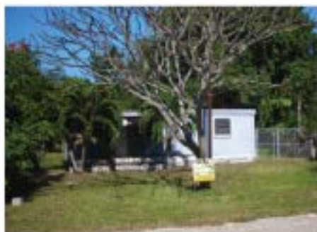
129 Coconut Row Facing Northeast
