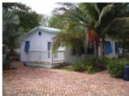
114 Lowe Street Facing Southwest
