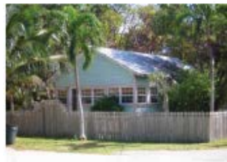
180 Lowe Street Facing Southeast
