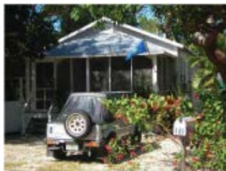
181 Lowe Street Facing North
