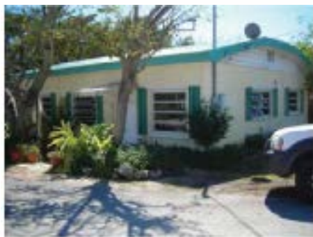
140 Atlantic Circle Drive Facing Southeast at
