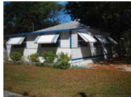
149 Sunrise Drive Facade Facing North of Northwest
