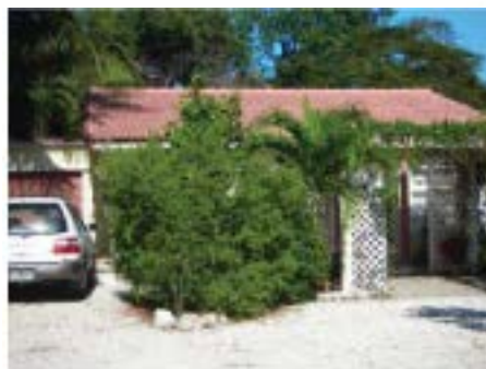
115 Coconut Row Facing North-Northeast
