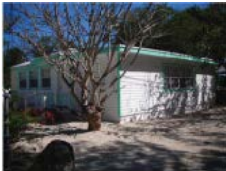
143 Sunrise Drive Facade Facing Northeast
