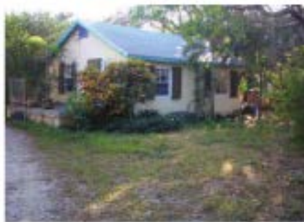
178 Beach Road Facing Northwest
