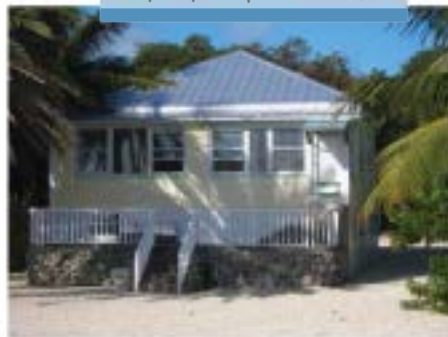
256 Tarpon Street Facade Facing West
