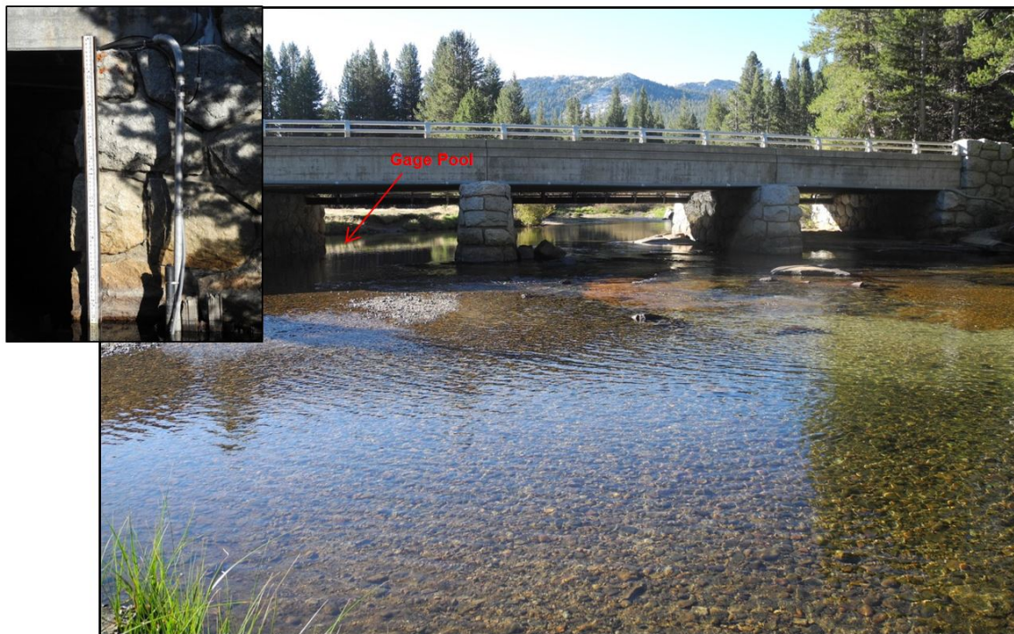
Figure 6. Looking upstream at the section control and gage pool at the Tioga Road gage. Inset: Looking downstream at staff gage.
