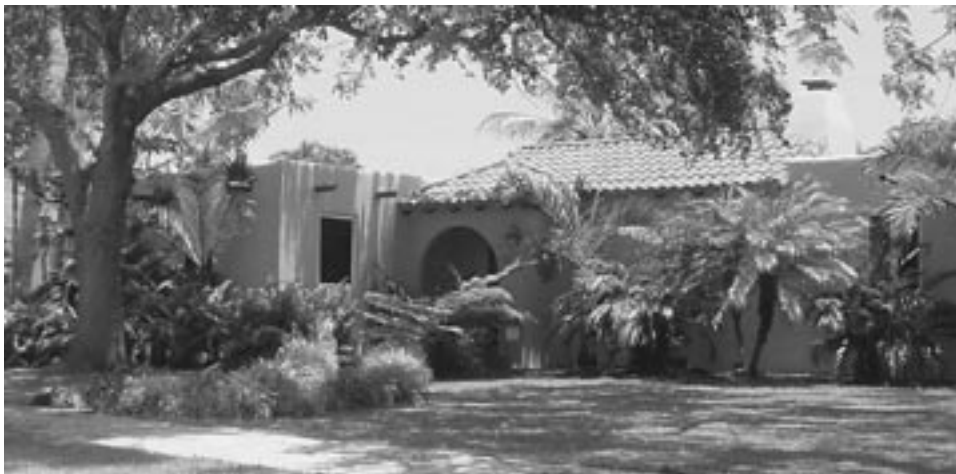
Pueblo Style Residence - Hollywood Lakes
