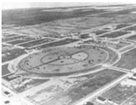
Aerial view of Harding (Young) Circle looking northeast, 1924.
