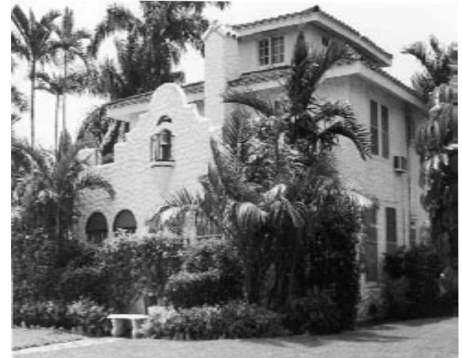
840 Hollywood Boulevard - Contributing Structure c. 1920's.
