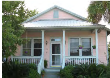
An existing building represents embodied energy. (710 Estrada)
