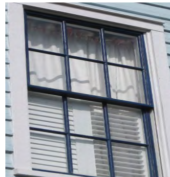
Original six-over-six wood sash windows. (715 San Fernando)
