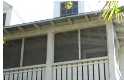
This porch has appropriate screen panels and remains transparent (902 Ladies Street).
