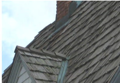
The use of wood shingle roofs as a replacement material is appropriate for contributing dwellings (910 San Fernando Street).
