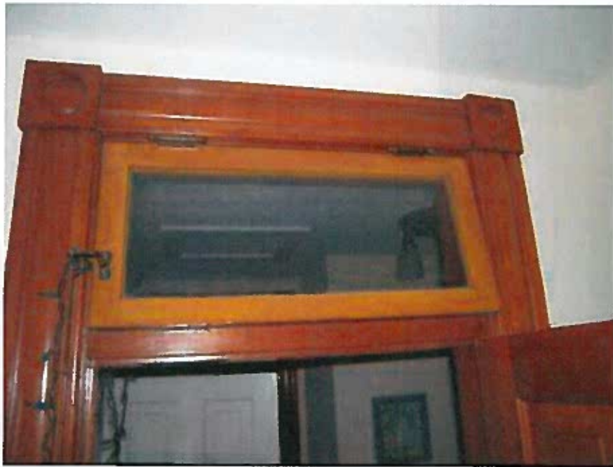
Detail of period molding and transition block surrounding the doors and windows in room 202. This woodwork is typical throughout the 2 nd floor. Photo Credit: Herb Dawson, NPS.
