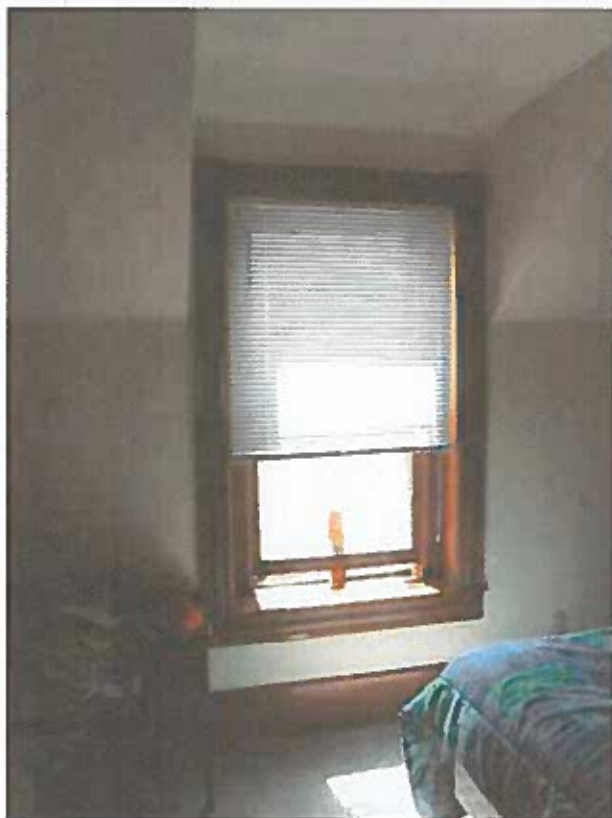
Bedroom 202 in the SW quadrant of the 2 nd floor. Note the change in ceiling slope to accommodate the original dormer window. Wall finishes have been re-surfaced within the guidelines of DOI standards. Photo Credit: Herb Dawson, NPS.
