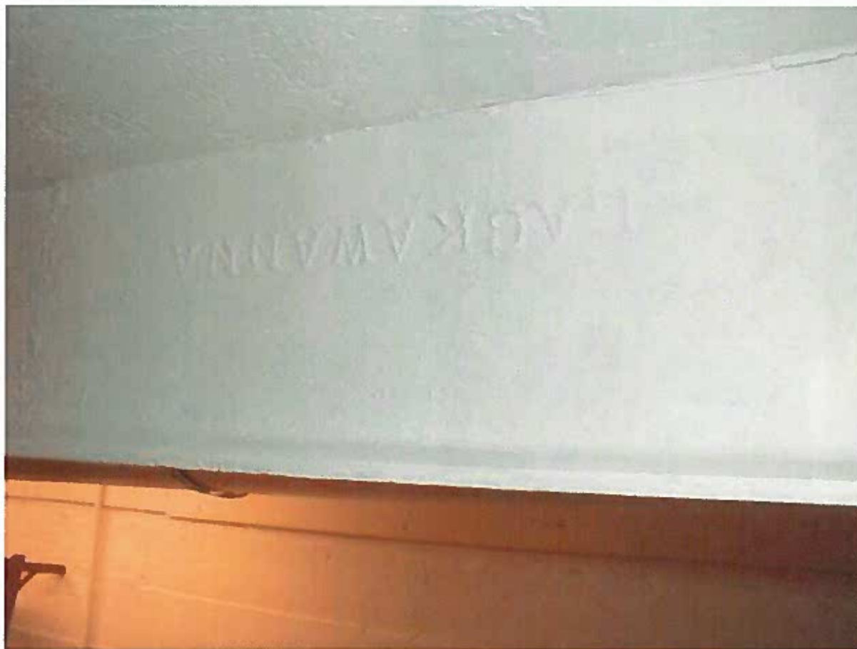
Steel support girder across the center of the north end of the house (see plan for location). The fabricator's foundry mark is visible on the side of the beam. Photo credit: Ken Sievert.
