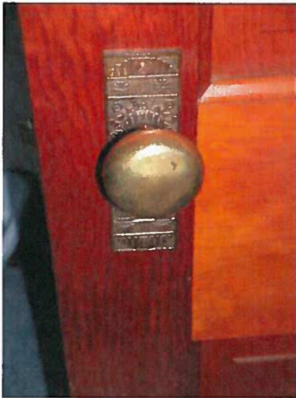
Historic door hardware on the entrance door into Bedroom 202. Photo Credit: Herb Dawson, NPS.
