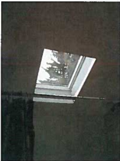
Introduced skylight above bathtub in Bathroom 203. Photo Credit: Herb Dawson, NPS.
