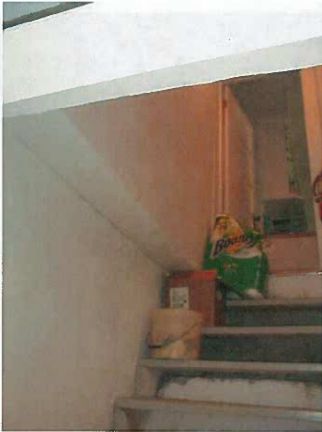
Looking up into the stairhouse of the utility stair serving the basement area.
