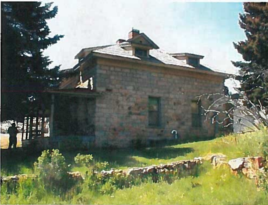
North Wall. Note that the east facing dormer windows interrupt the roof fascia whereas the north facing roof dormers are surrounded by roofing. Photo Credit: Ken Sievert.
