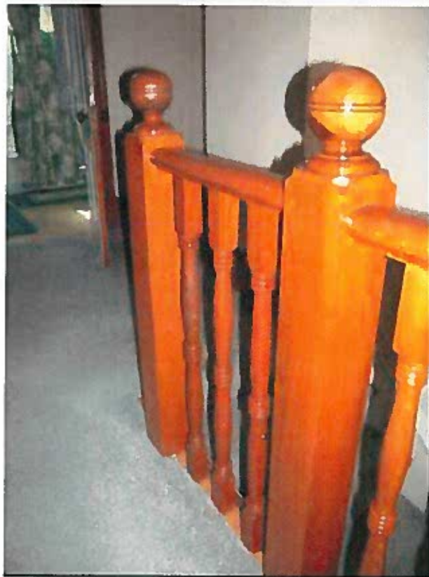
The upper landing has been re-configured at some time during the structure's history as evidenced by the duplication in Newel Posts at the top of the stair. Photo Credit: Herb Dawson, NPS.
