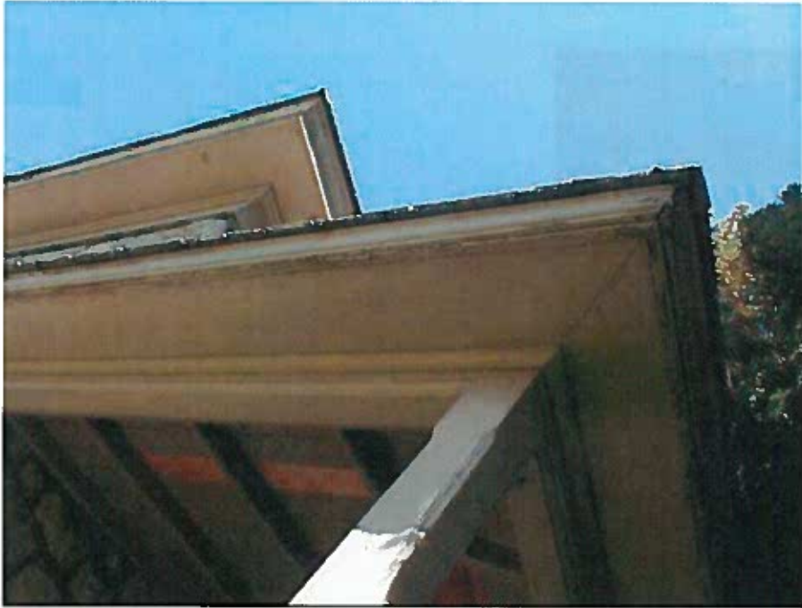
Soffit, fascia, and roof edge detailing at the porch; with the upper roof visible in the background above. Photo Credit: Ken Sievert .
