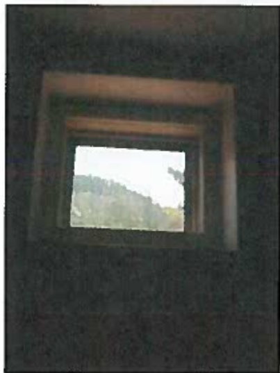
Replacement window in west wall of first floor bathroom. This window has been installed in an opening once used as a cell window.
