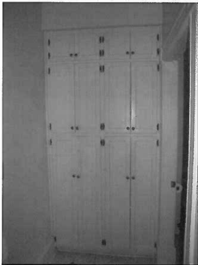
New cabinet at end of sub-co rridor from Kitchen to Bathroom / Utility. Photo Credit: Herb Dawson, NPS.
