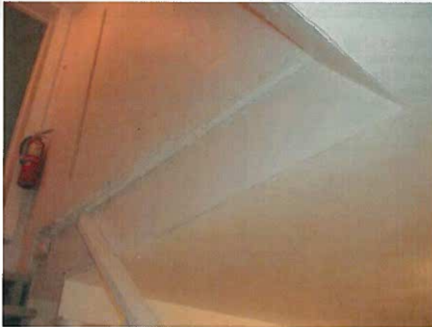
Transition of the basement ceiling to the utility stair, looking NW. Photo Credit: Ken Sievert
