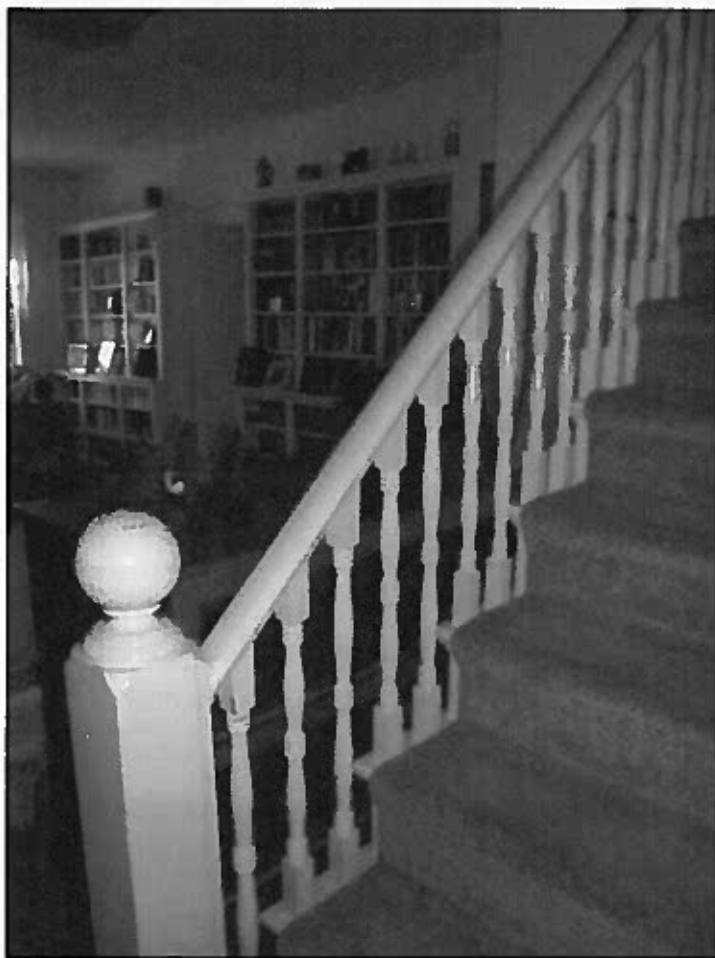
Detailing of stair between the Living Room and the sleeping areas located on the upper floor level. The woodwork in the railing, balustrade, and baluster posts may originally have been stained or natural. Photo Credit: Herb Dawson, NPS.
