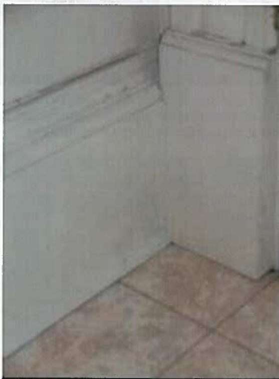
1 st floor Bathroom, base moulding. Photo Credit: Herb Dawson, NPS.
