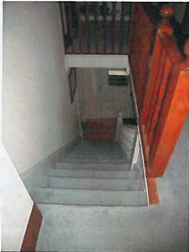
Main (and only) stair between first and second floor. Note the change in finishing of the woodwork between the floors. Photo Credit: Herb Dawson, NPS.
