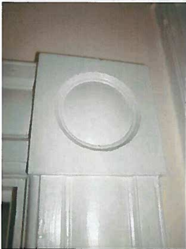
Label block and period casing around interior door between kitchen and dining. Photo Credit: Herb Dawson, NPS
