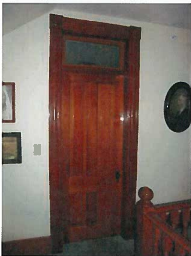
Entrance into Room 206 from the upper stairhall. The standing and running trim, transom, and door are typical throughout the floor and are all historic. Photo Credit: Herb Dawson, NPS.
