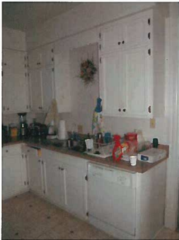
SW corner of kitchen showing treatment of cabinetry, woodwork, and flooring. Photo Credit: Herb Dawson, NPS.
