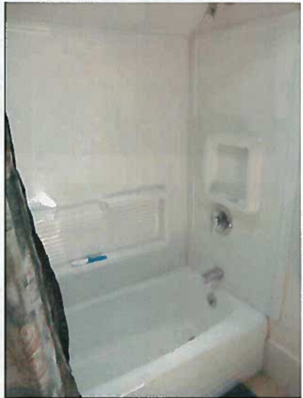
View within Bathroom 203 on the 2 nd floor of the U. S. Commissioner's house. All plumbing fixtures are contemporary. Photo Credit: Herb Dawson, NPS.
