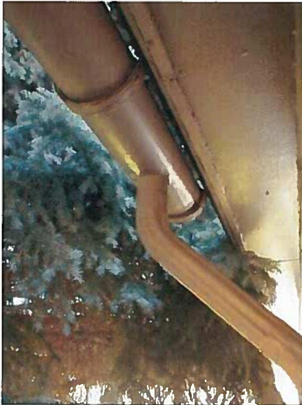
Calvary style half-round gutter at front porch. Similar gutters are used at the 2 nd floor dormers. Photo Credit: Ken Sievert.
