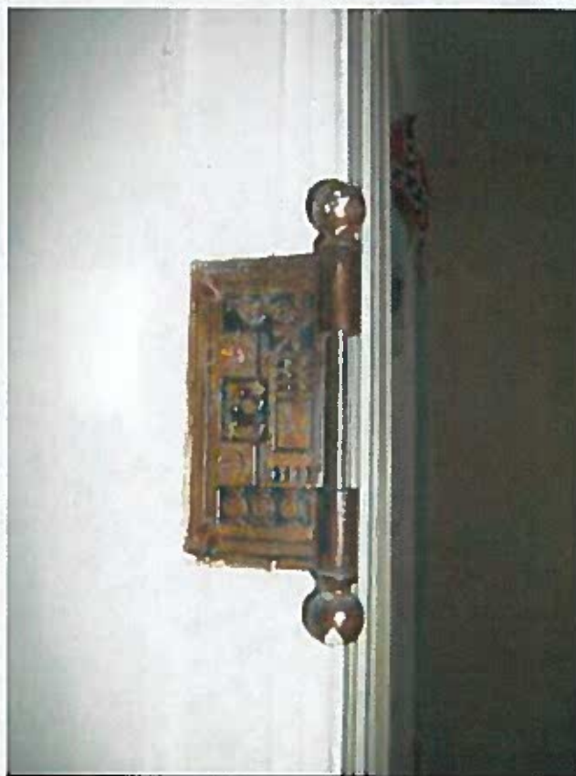
Figured hinges for door; the door is stored and the opening between kitchen and dining is open. Photo Credit: Herb Dawson, NPS.
