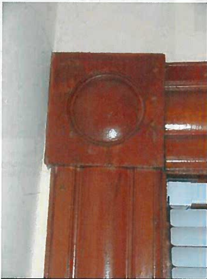
Detail of period molding and transition block surrounding the doors and windows in room 202. This woodwork is typical throughout the 2 nd floor. Photo Credit: Herb Dawson, NPS.
