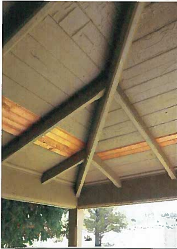
Roof framing and underside of sheathing at entrance porch. Photo Credit: Herb Dawson, NPS.
