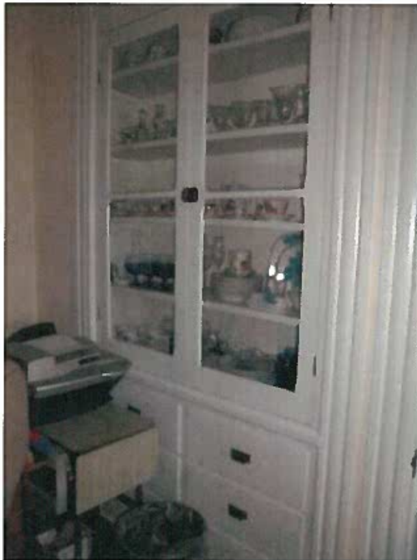
Interiors: built-in cabinetry between the kitchen and dining rooms. Note the bead pattern boards used for the back of the cabinets. Photo Credit: Herb Dawson, NPS.
