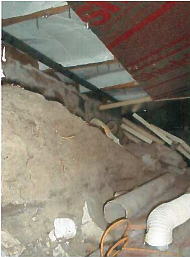
East access into the crawl space from the basement stair. The stone foundation can be seen as well as the earth berm against the footing. Note the contemporary weatherization materials applied to the floor structure. Photo credit: Ken Sievert
