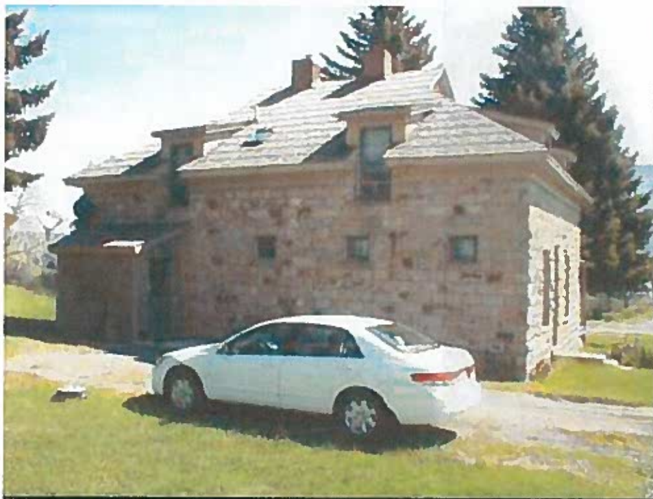
West Wall; the vestibule at the back door (shed roof) is not original. The three small square windows once served jail cells within the facility. Photo Credit: Ken Sievert.
