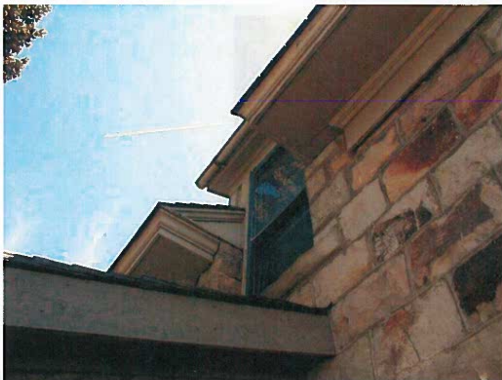
NE dormer above back door entrance vestibule. The relationship of the shaped ogee fascia, frieze board, and stonework can be seen in this photograph. Note that the newer fascia on the vestibule addition is a plain flat board. Photo Credit: Ken Sievert
