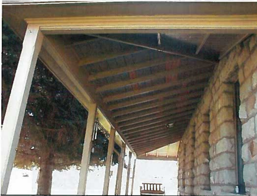
Underside of porch roof along the East (primary entrance) side of the U. S. Commissioner's house. The members supporting the roof were always intended to be exposed as evidenced by their careful positioning, finished surfaces, and chamfered corners. Photo Credit: Ken Sievert.
