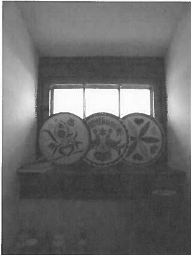
South facing dormer window within Bedroom 202. Note that this is one of the dormer windows that does not extend through the plane of the roof but is surrounded by the roof (see exterior elevations). Photo Credit: Herb Dawson, NPS.
