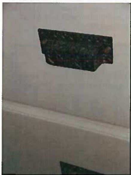
Drawer pull detail at built-in cabinets shown on previous page. Photo Credit: Herb Dawson, NPS.
