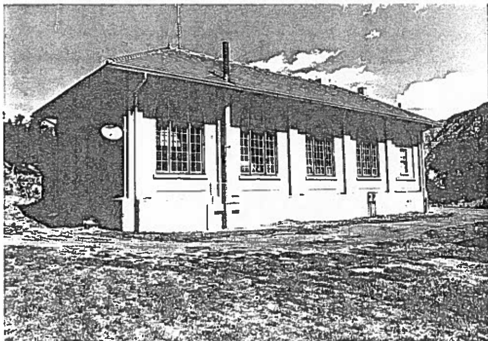
Figure 27. Looking northeast at the power house. Note the low area along the building where some of the site water drains into the foundation. There is minor concrete base deterioration at this point.
