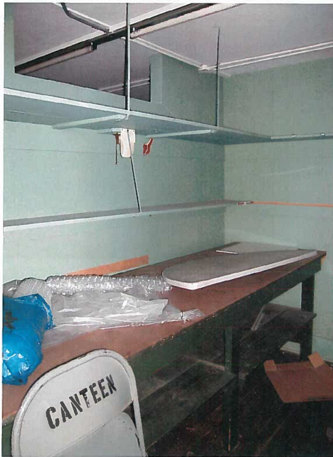
Work room 115; since this is an internal area without windows, the opening in the top of the wall is believed to be for ventilation. The use of every available space for storage continues into this space.
