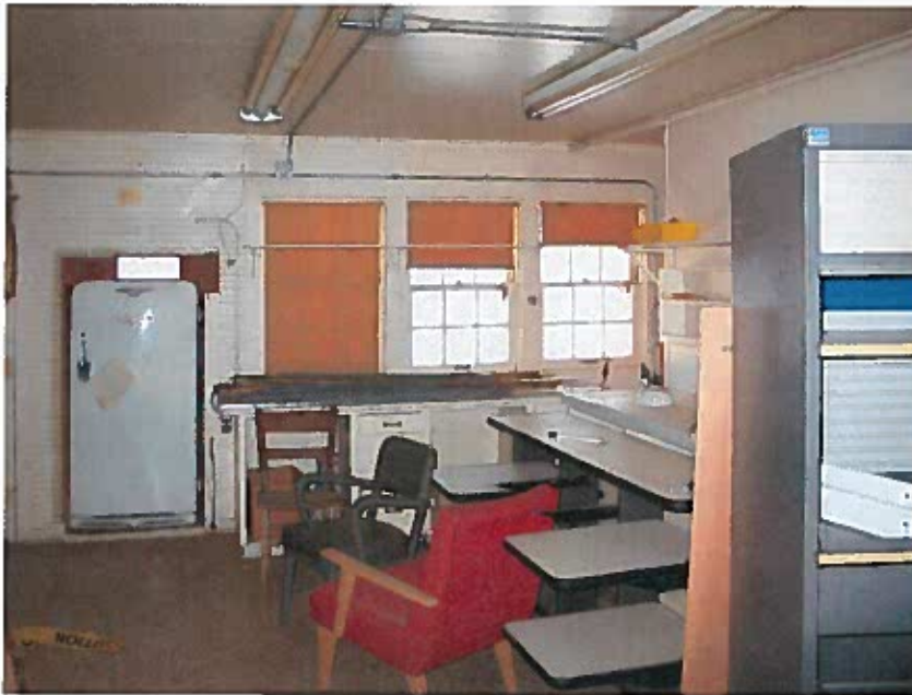
General view of the kitchen area, looking east. The refrigerator is built into a projecting alcove that extends outside the plane of the exterior wall.
