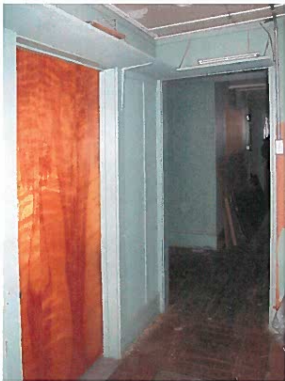
Northeast corner of room 105; note the introduction of the contemporary door.
