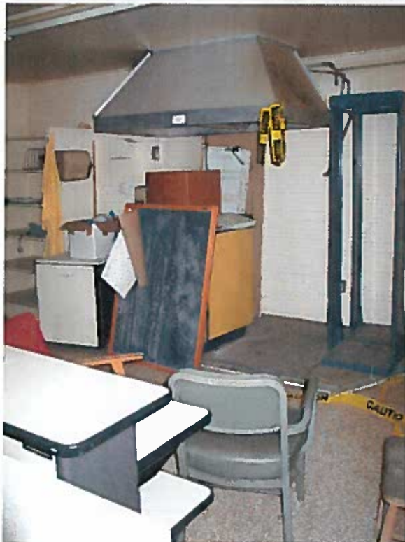
Commercial range hood attached to the ceiling of the kitchen; note the concrete slab beneath where the ranges were located.
