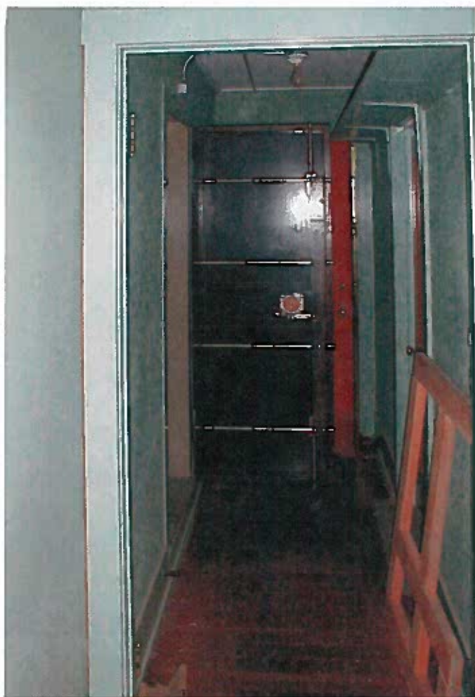
The first floor vault at the Haynes headquarters is substantially constructed with concrete and reinforcing; the interior is plastered. The steel door shown above befits the vault class used at the facility.
