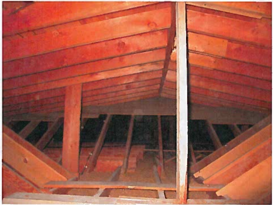
Intersection of the roof framing from the north wing with the pyramidal roof framing above the retail area.
