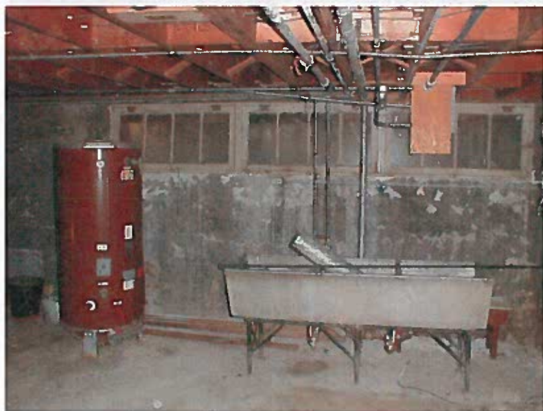
East wall of the partial basement; the windows originally admitted light through the lightwell along the east side of the dormitory wing.
