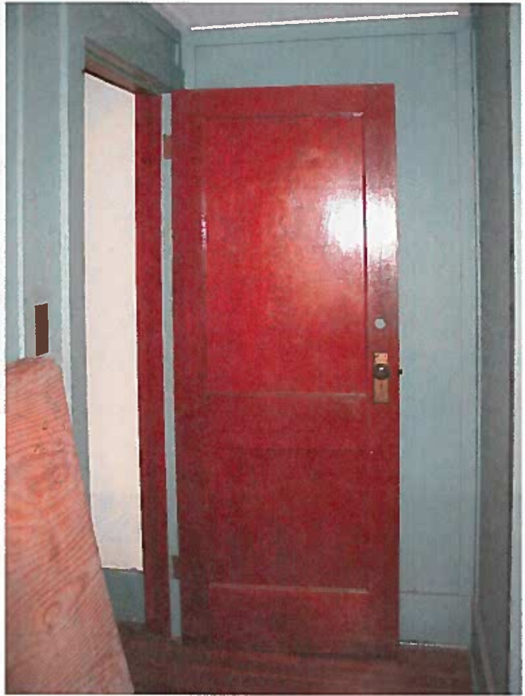
Typical rail and stile fir door used at all dormitory room locations. Many of these doors are in good condition. Their future use would depend on the level of alteration proposed for the structure and the implications of fire codes as a result of those alterations.
