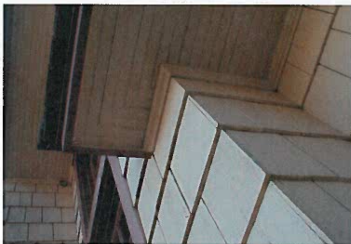
Detail of the bead-patterned wood soffits that finish the edge of the roof.
