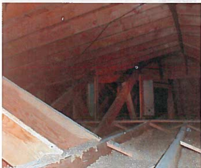
Closer view of bracing that extends back into the west wing of the dormitory.
