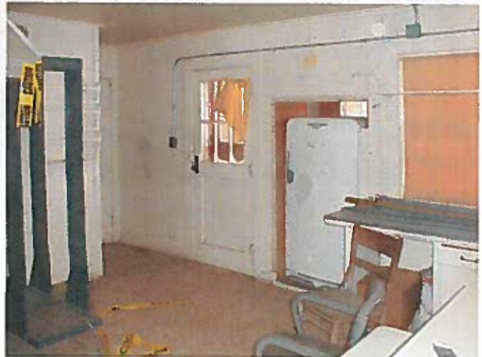
Northeast corner of the kitchen; the entrance into the basement is from the far corner of this space. Beaded-pattern wood surfacing is used extensively on the exterior kitchen wall.
