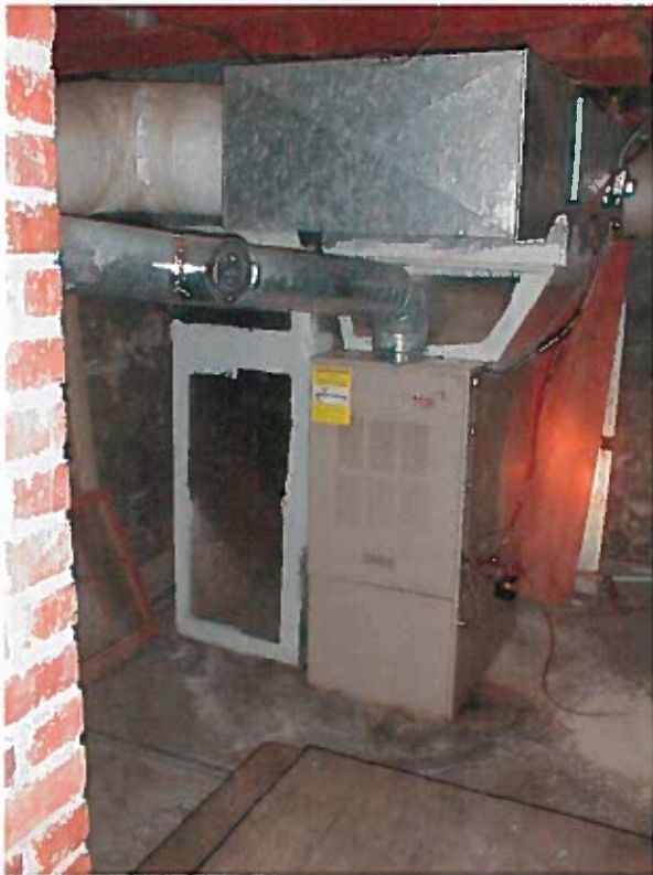
This furnace was added in the basement relatively recently during the facility's use.
