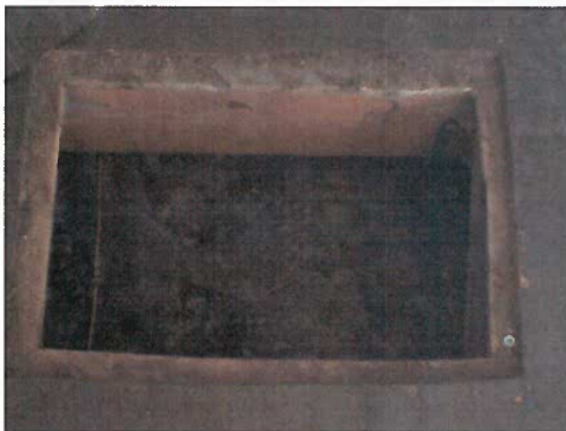
Figure 3. View of an access panel in the southwest corner of the main ground floor eastern room. The access area is about 0.5 meters (1.5 feet) in length by 0.3 meters (1 foot) in width. View to the west taken January 16, 2008, 10:11 am MDT.
