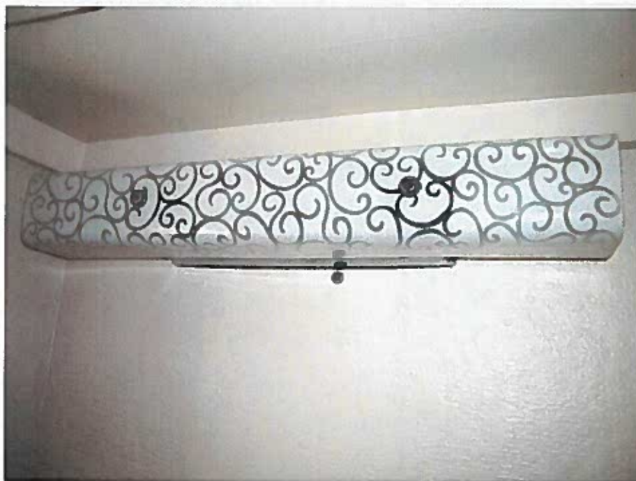
Light fixture at the first floor unisex toilet; it is judged to be of contemporary origin.
