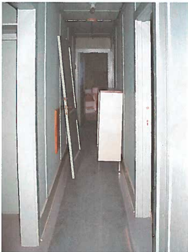
Corridor serving three dormitory rooms at the south end of the first floor. The tongue and groove fir flooring has been painted grey throughout this area.
