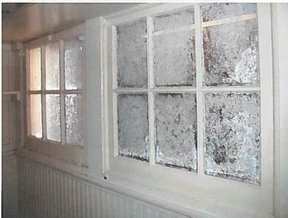
South facing windows from bathroom 106; window sills and wainscot cap heights are aligned.
