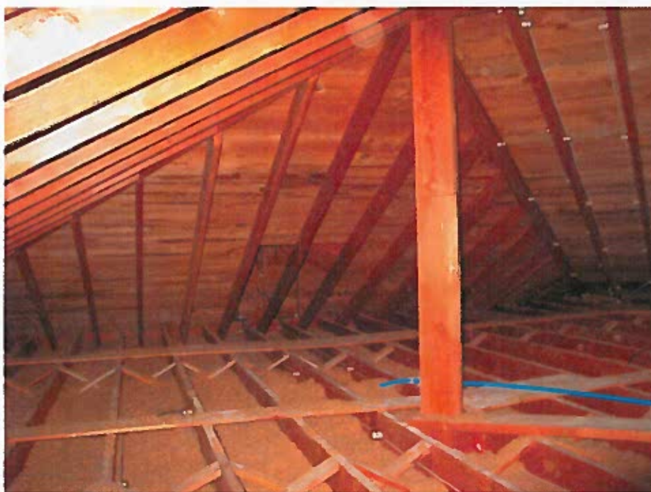
Another view of framing above the retail area; note the framing for the saddle that extends behind the north facing pediment and the extensive use of knob-and-tube wiring.
