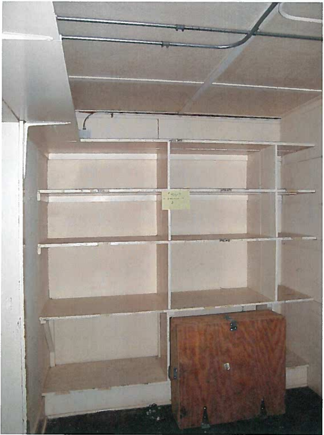
Storage room 110; a significant amount of storage space was located on the first floor in close proximity to the retail sales area.
