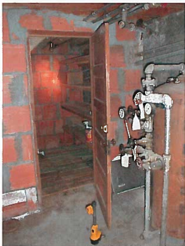
This structural clay tile enclosure is constructed below the basement access stair. Its purpose is not known, but the presence of wood floor sleepers suggests that materials that either had to be cooled or were caustic were stored here.
