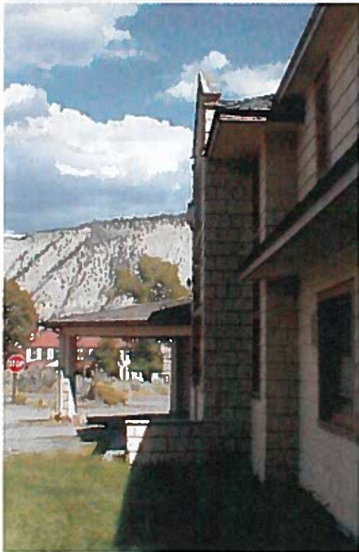
Oblique view of the north wall; structures from Fort Yellowstone and Mount Everts can be seen in the background. Note the pediment above the north wall of the retail sales shop.
