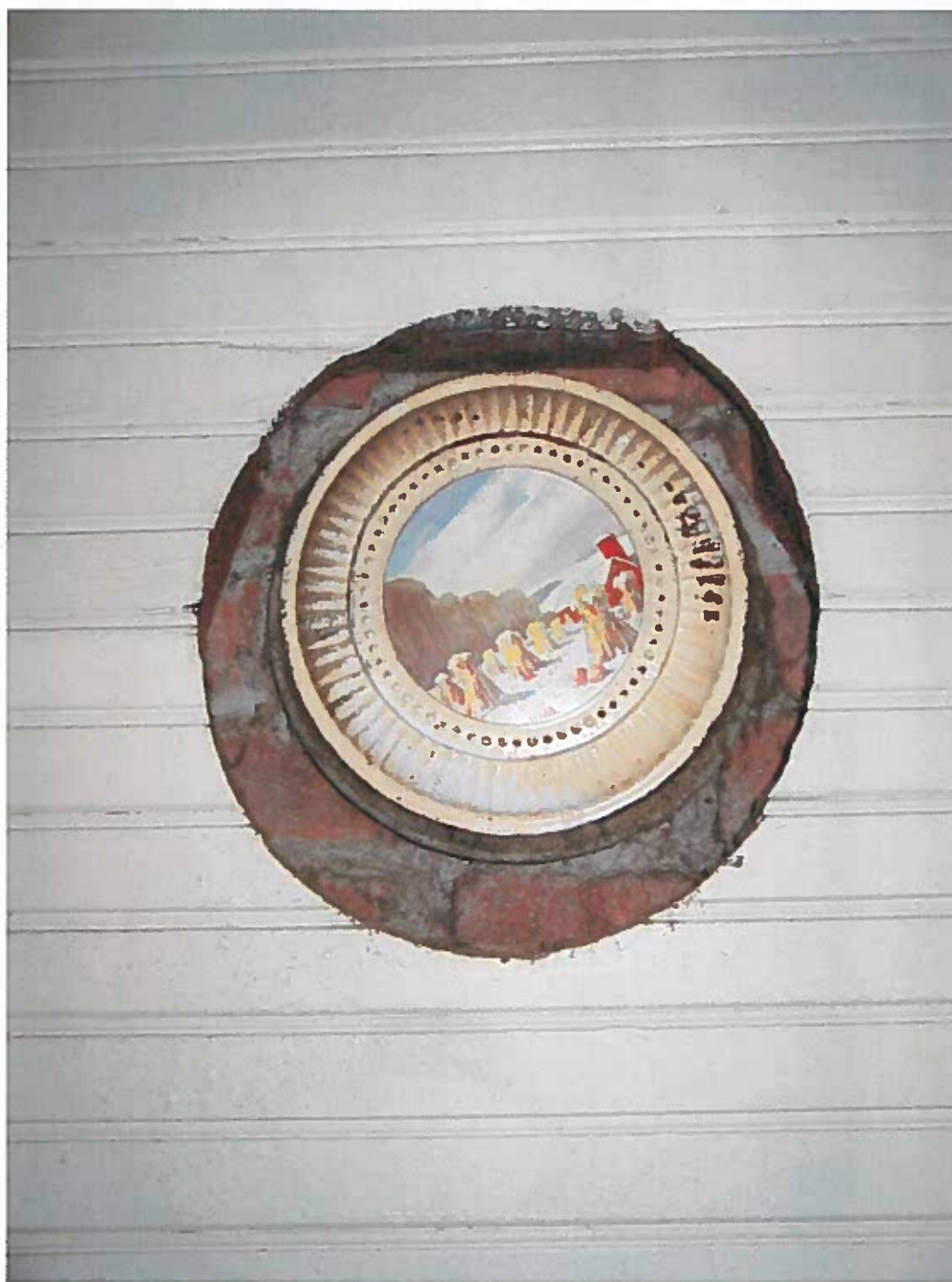
Decorative thimble in the brick chimney at the west wall of the kitchen.
