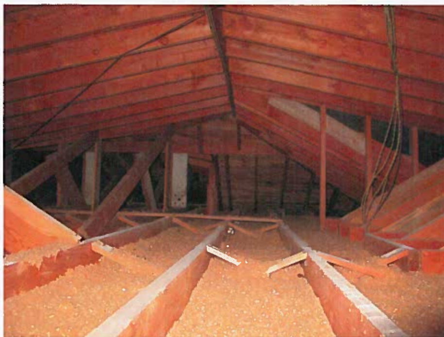
Attic framing above the northeast corner of the structure; the change in roof slope reflects the massing at the exterior of the building.
