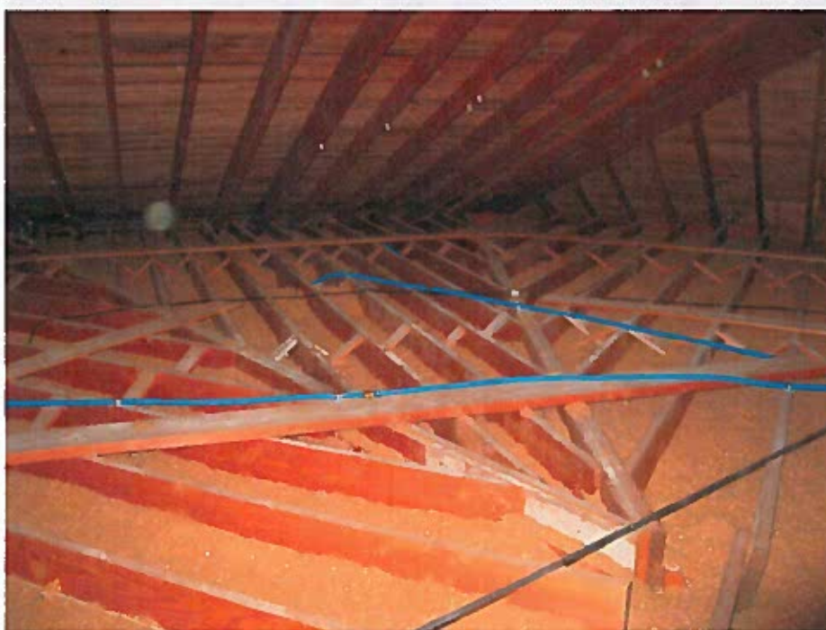
This is the ceiling joist pattern above the retail sales area's angled corner. It reflects the pattern of the fan trim on the ceiling below.
