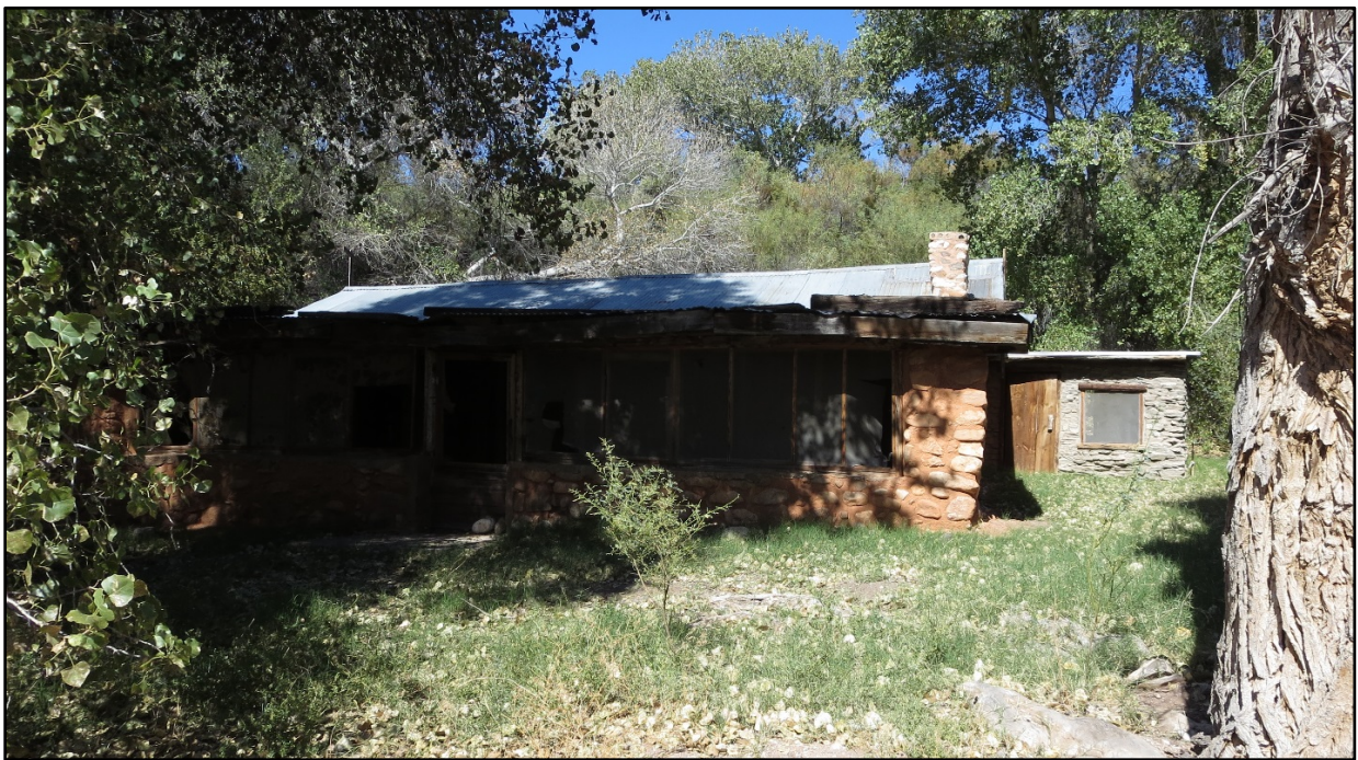
Figure 3. Historical Tassi Ranch downhill of the irrigation canal.
