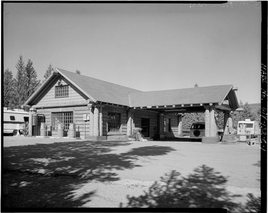
Figure 6.5. Attic attainment site and roost #3: Fishing Bridge Service Station (in the picture still referred to as Hamilton's Store). The highest elevation site. Bats exit through multiple areas on each side of the building. The upstairs window opens to the inside of the attic. Roost Type B: microclimate experiencing the greatest daily temperature variation and lowest daily temperature drops. Picture courtesy of U.S. Government, National Park Service.
