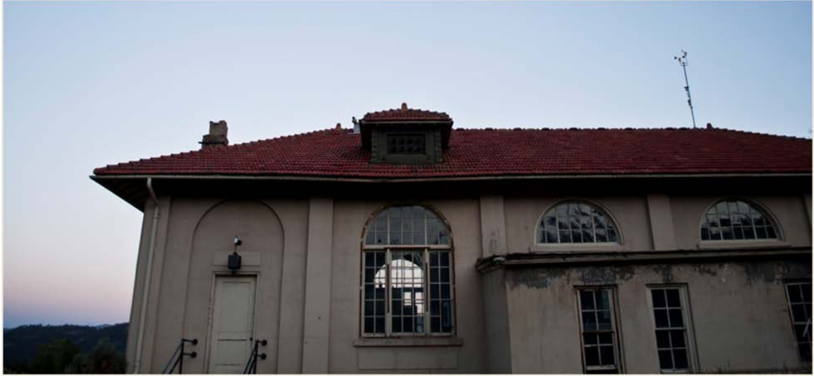
Figure 6.6. Roost #4: Power House, Mammoth Hot Springs, WY. Building is now condemned due to asbestos and other dangers. Bats exit primarily through the outcropping on the roof referred to as the “bat cannons.” Roost Type A: the warmest microclimates.
