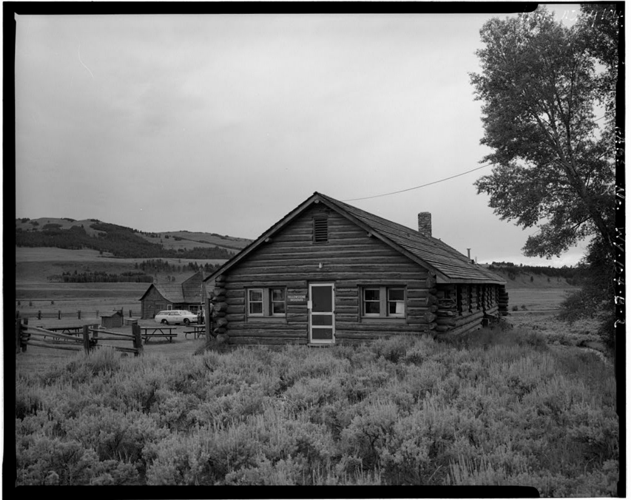
Figure 6.3. Attic attainment site and roost #1: The Bunkhouse at Buffalo Ranch in Lamar Valley. Bats exit primarily through the visible vent above the door. Roost Type B: microclimates with the most daily temperature variance. Picture courtesy of U.S. Government, National Park Service.
