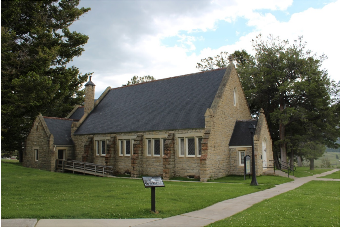
Figure 6.7. Roost #5: Chapel, Mammoth Hot Springs, WY. Bats exit primarily via non-visible cracks throughout the side of the chapel shown in the picture. Roost Type C: the most stable and steady microclimate.
